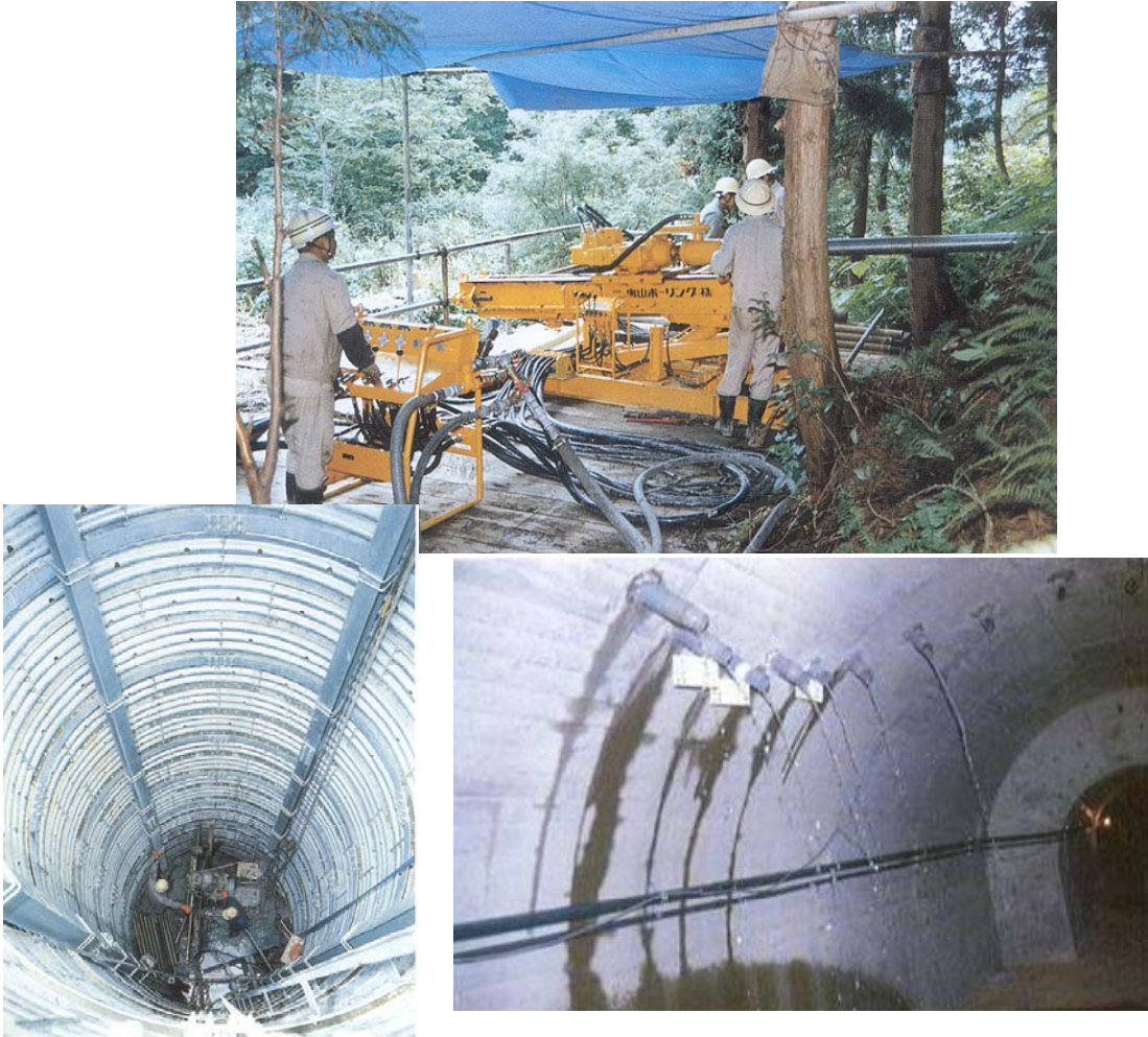
Fig.2 Comprehensive drainage measures: Sub-horizontal Drainage Boreholes (upper). Vertical Drainage Wells (lower left). Drainage Tunnels (lower right). Both drainage wells and drainage tunnels are associated with numerous sub-horizontal and sub-vertical boreholes for groundwater collection.
