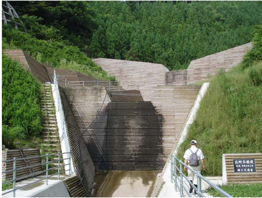
Fig.6 Check Dam with Pitching Logs: pitching logs in front of the dam body harmonize with the surrounding forest landscape.
