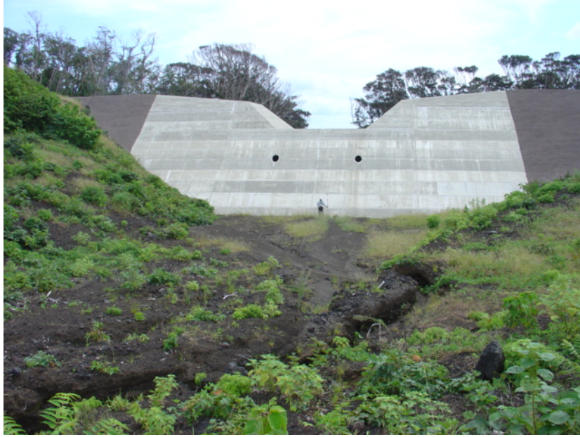
Fig.7 Check Dam Made of Soil Cement: the wings are made of soil cement and the spillway is made of concrete.
