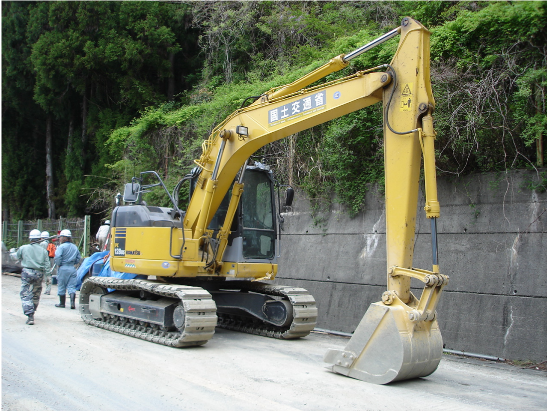
Fig.9 Backhoe operated by Unmanned Construction System (UCS). Robot arm and surveying camera are set at the operating location. Operator remotely controls the machine by the robot arm and camera.
