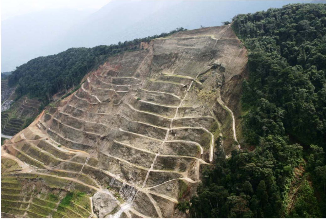
Fig.14 Pos Selim Landslide in Malaysia. Detailed investigations of the complex geology and hydrogeology conditions have been performed to define the landslide mechanisms.
