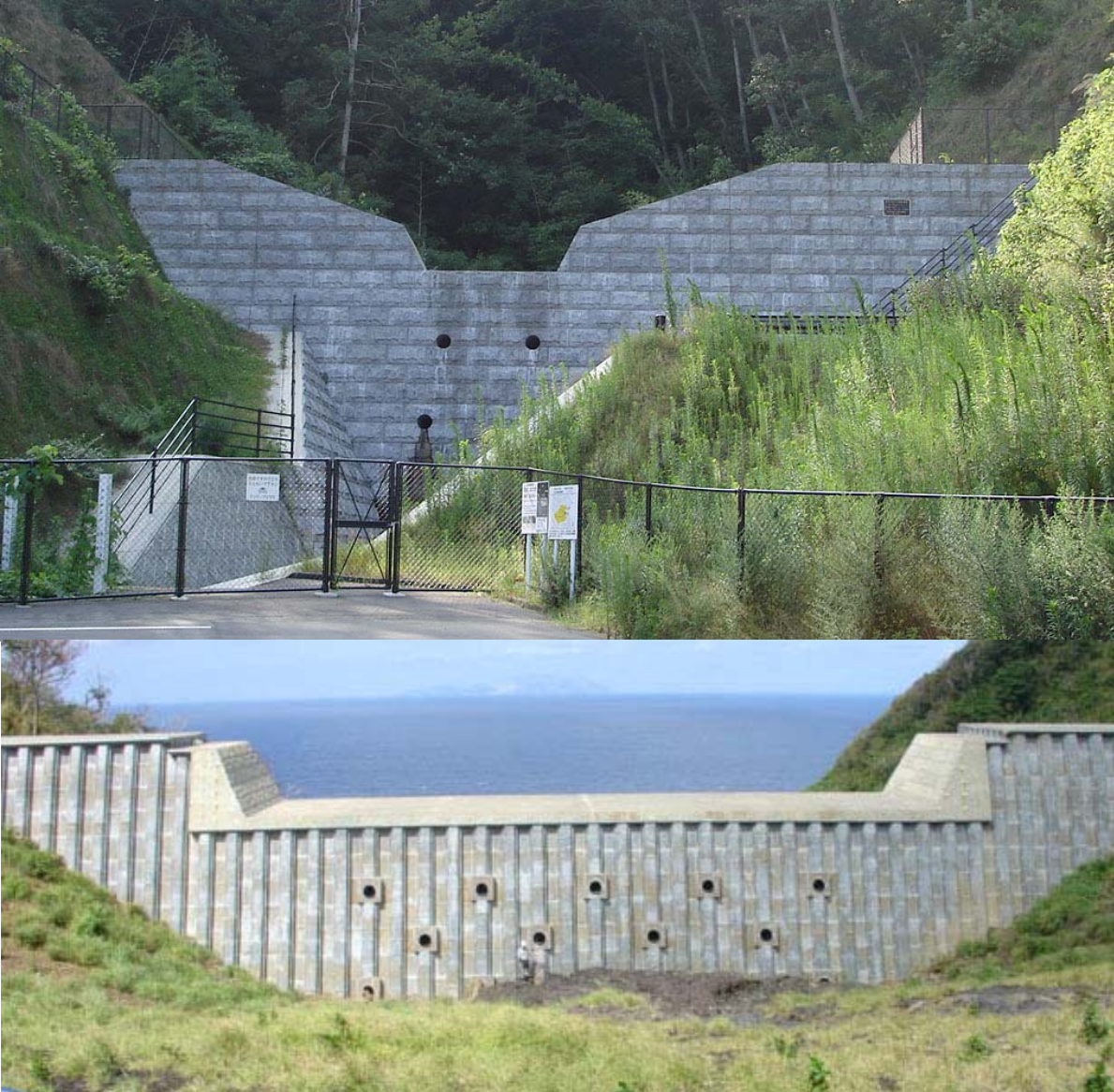
Fig.5 Concrete Check Dam (upper): concrete panels are pitched in the front of the dam body in order to harmonize with the surrounding landscape. Check Dam Filled with Local Sediment (lower): steel panels cover the dam body consisting of sediment.
