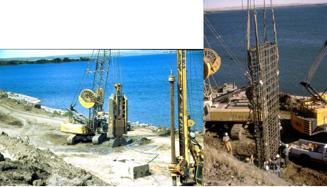
Fig.13 Remedial Measures of the Deep Seated Forest City Landslide: Excavator used to construct the one meter by three meters shear pins (left). Reinforcing cage being lowered into the excavation (right).
