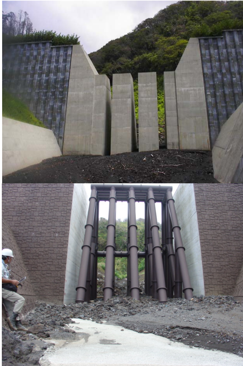
Fig.10 Open-type Check Dam: The Concrete Slit Dam (upper) is expected to have both sediment capture and retrieval functions as well as sediment discharge control function. The Steel Pipe Grid Dam is expected to catch the debris flow and discharge the captured sediment after the debris flow.
