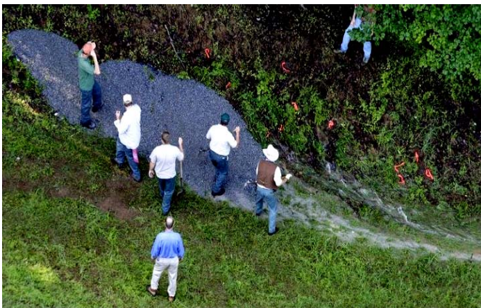
Spreading gravel over the leak in preparation for filter
