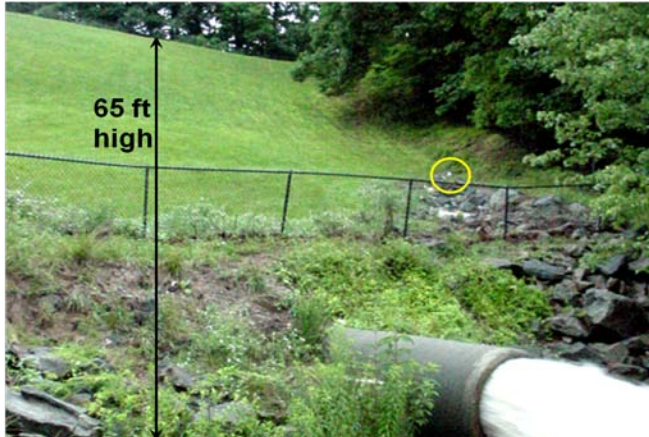
Seep on left abutment viewed from downstream slope
