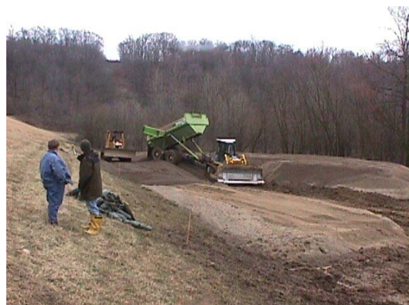
Construction of Weighted Filter Berm
