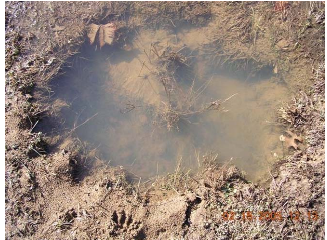
Four foot diameter boil at toe of dam
