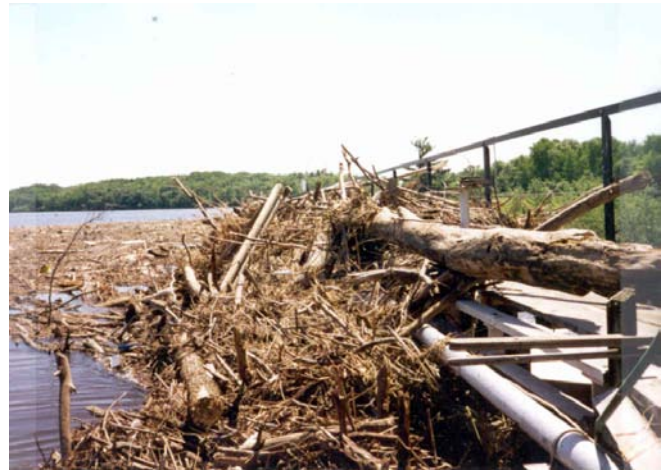
Debris clogging trip gates
