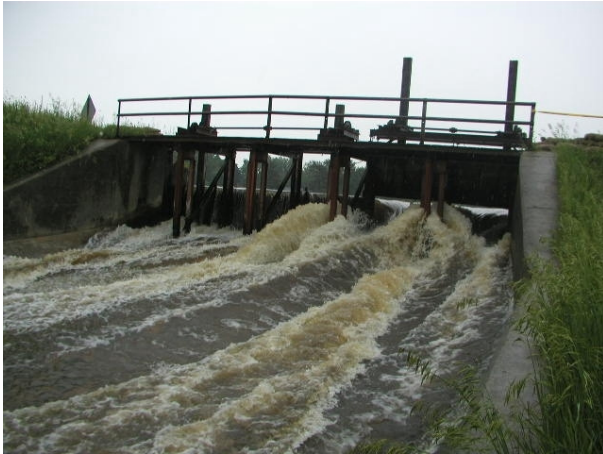
Main gates (just after flood)
