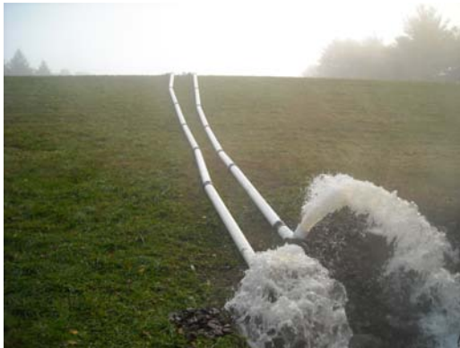
Two siphons on the downstream face.
