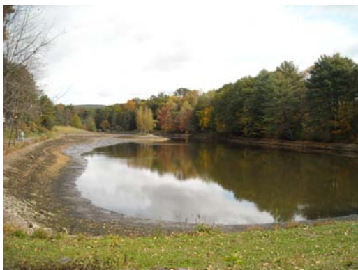
Current conditions at the dam.
