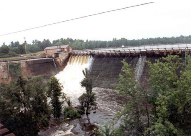
Trip gate portion of dam
