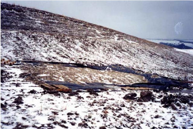
Repaired blow out
