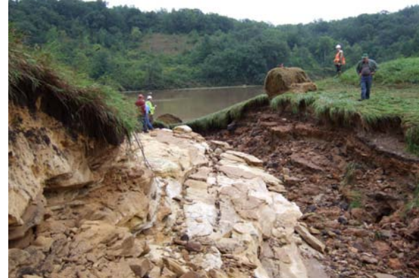
Aux. spillway crest with hay bail
