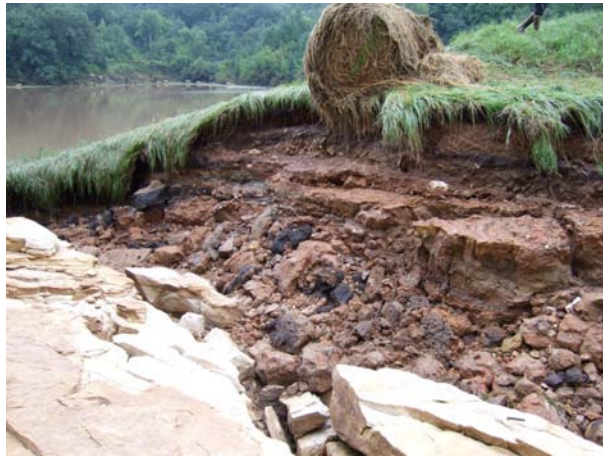
Aux. spillway crest with hay bail
