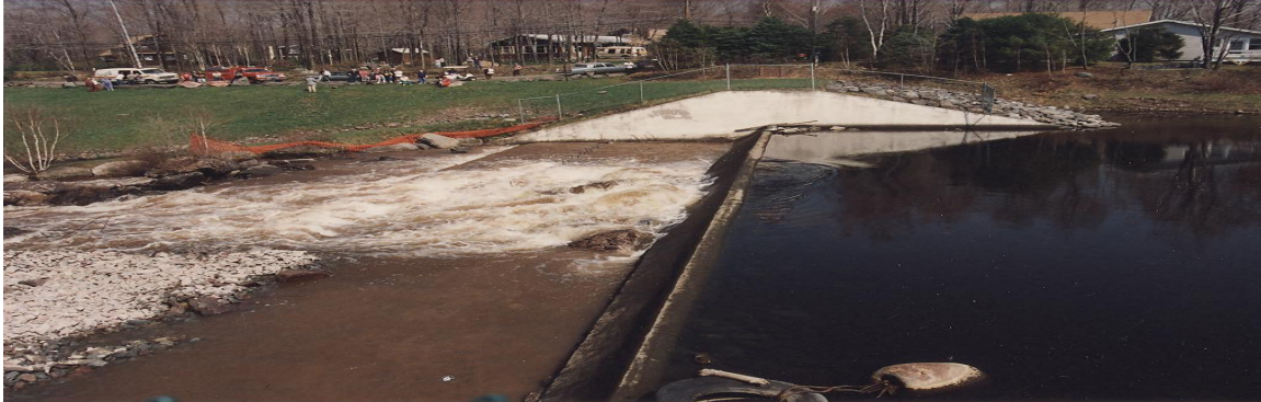
Whirlpool above weir with boil flowing downstream of weir.
