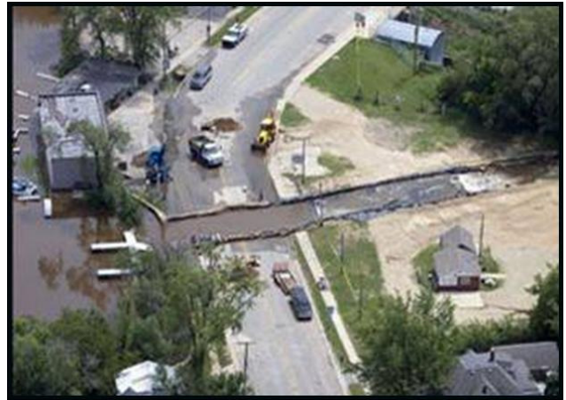
Emergency spillway from the air
