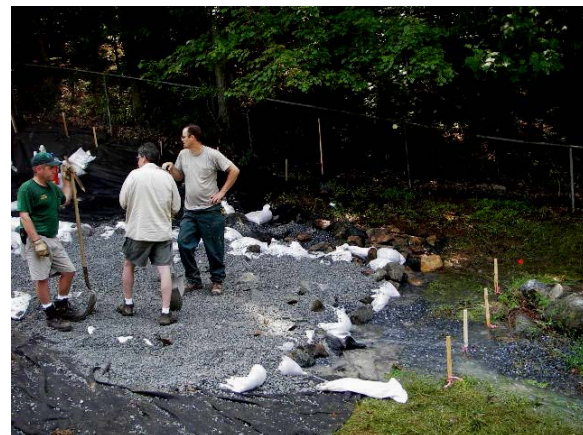
Filter Fabric with sandbags and gravel for weight
