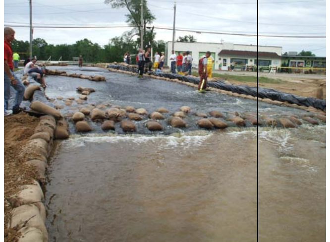
Downstream end with energy dissipation
