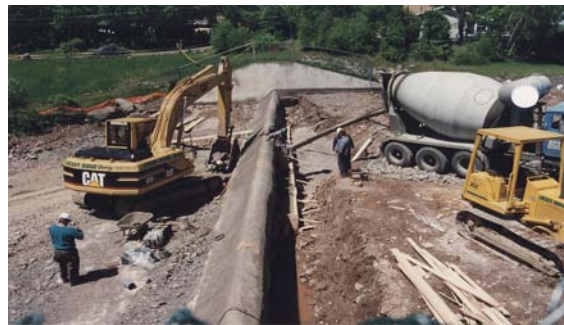
Repairing the void upstream of the weir.
