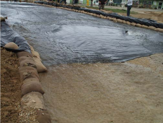
Downstream end of emergency spillway
