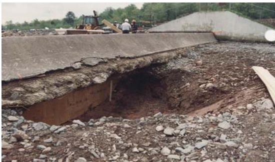
Void upstream of the weir.
