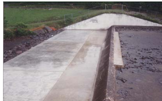
Repaired spillway.
