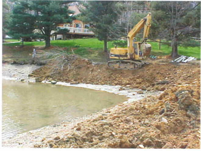
Breach in Progress
