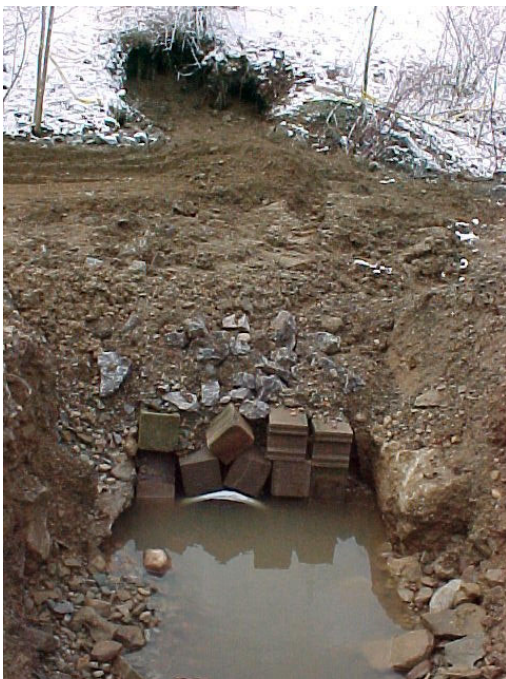
Temporary Repair Attempt
