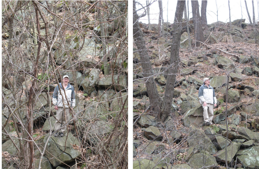
Fig. 3. Large sandstone riprap on the western (left) and eastern (right) remnants of the dam. These represent the downstream side of the dam and illustrate the excellent riprap used in the original construction, obtained mostly from excavation of the main spillway (photos by U. Kaktins). Large riprap like this was not used in reconstruction efforts by the SFFHC (see Fig. 4). The person shown stands 1.8 m high.
