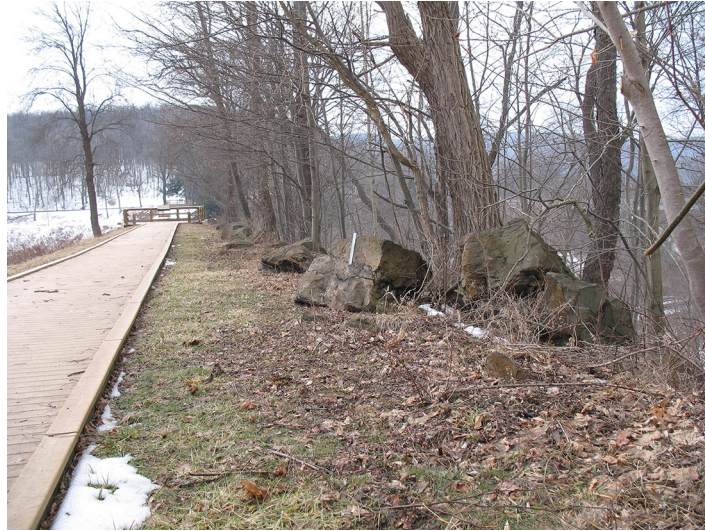
Fig. 5. View along crest of the eastern dam remnant, looking westward toward the observation platform. This part of embankment represents original construction. Large riprap from the original construction is still in place , standing more than 0.6 m higher than present crest, as a result of the embankment crest being lowered as much as 0.9 m by the SFFHC. White ruler on rock is 0.33 m long (photo by N. Coleman).
