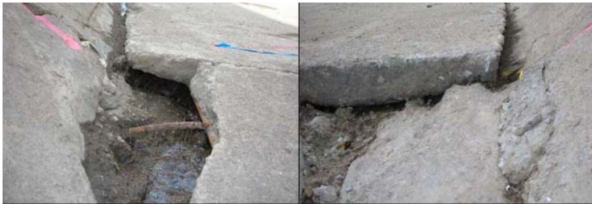
Figure 10. Unfiltered Openings in Canal Lining Immediately Downstream of Conduit Discharge Structure
