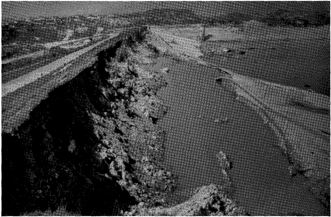
FEBRUARY 9, 1971, FAILURE LOOKING WEST Lower Van Norman Dam Figure 4
