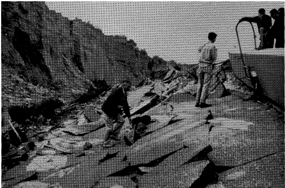
FEBRUARY 9, 1971, FAILURE COLLAPSED CREST OF DAM Lower Van Norman Dam Figure 5
