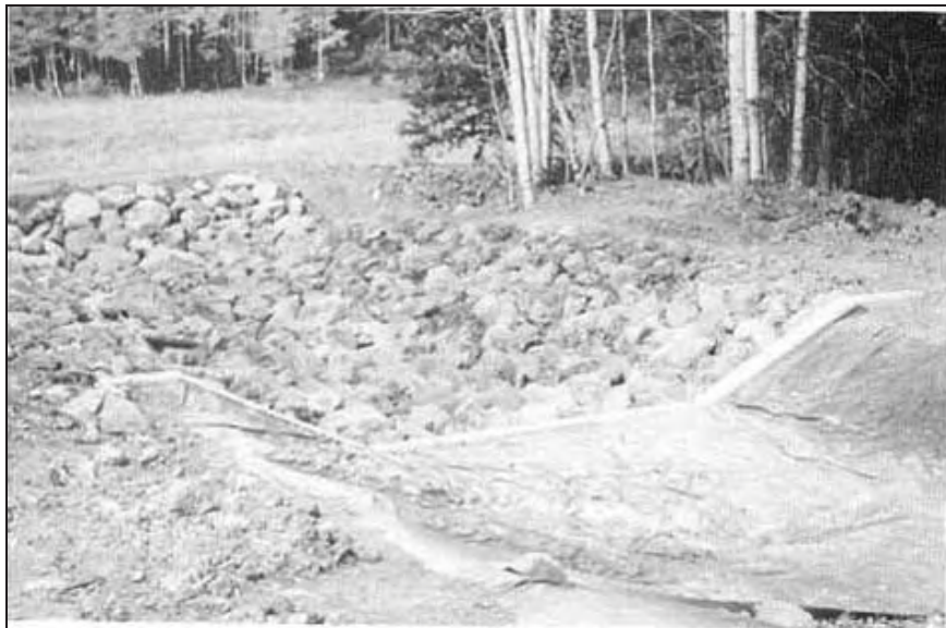
Figure Cottonwood-7.—Downstream end of geomembrane-lined spillway. Note concrete cutoff wall (Reclamation figure republished in Timblin et al., 1988).
