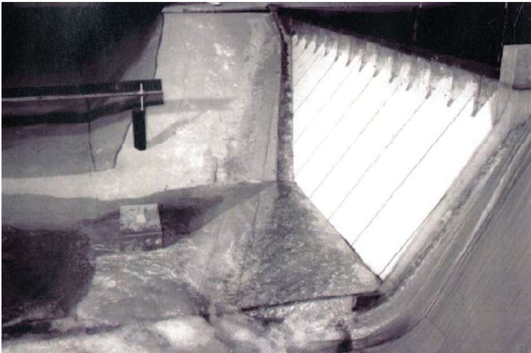
Figure Tygart-4 - Type 4 design, PMF overflow on right side of dam ( Q = 373,120 \text{ ft}^3/\text{s} ) (Courtesy of USACE, 1999)
