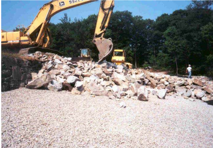
Figure 8-1.— Dumped riprap placement on 6-inch bedding layer for Upper Stoneville Reservoir Dam, Massachusetts (Wooten and Wood, 2002, Courtesy of ASDSO and GEI Consultants, all rights reserved).
