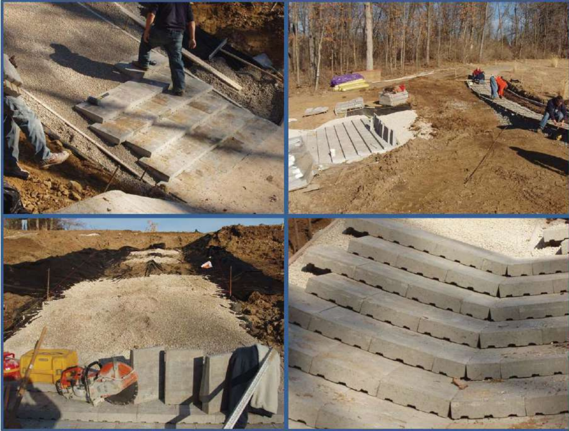
Figure Friendship Village-2. — Top left photo is of ArmorWedge block placement over graded bedding material near toe
