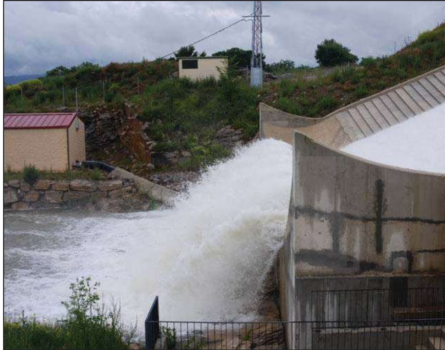
Figure Barriga-16.—Side view of the flip bucket operating (courtesy of Morán and Toledo, 2006, all rights reserved).
