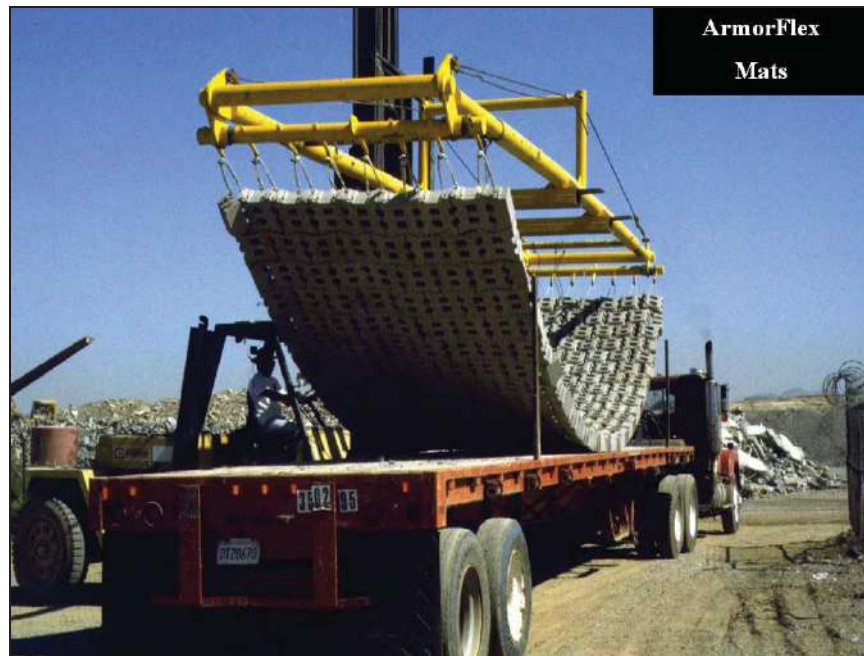
Figure Strahl 1.—Typical transport and stretcher bar, and crane, used for placing cable-tied block mats (Courtesy of Contech Engineering Solutions, all rights reserved).
