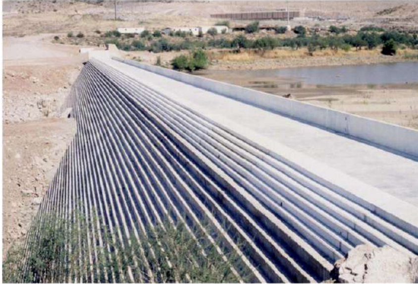
Figure 12-1.—Completed RCC buttress at downstream face of Camp Dyer Diversion Dam in Arizona. Conventional concrete was used for the overflow crest and approach apron. The stepped surface provides energy dissipation for overtopping flows (Reclamation).
