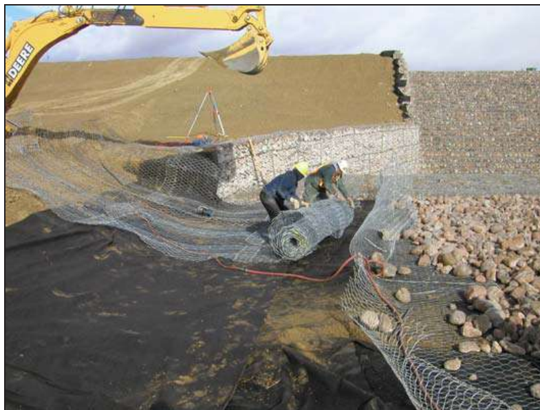
Figure West Cornfield-3.—Unrolling gabion mats in stilling basin (Courtesy of Maccaferri, Inc., all rights reserved).
