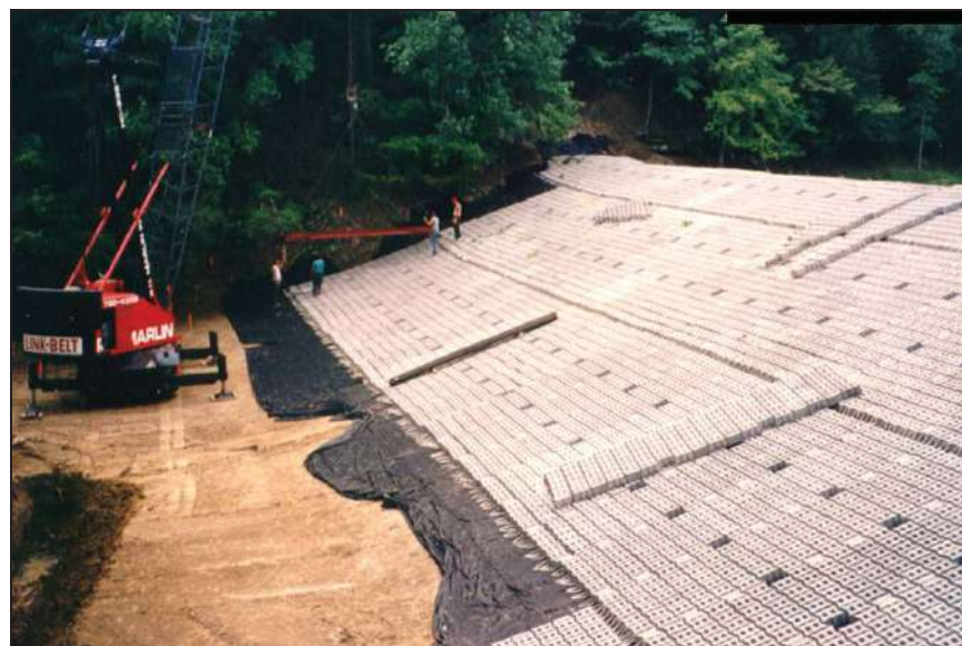
Figure Strahl-2.—Placement of the cable-tied mats over a geotextile on the downstream face of Strahl Lake Dam (Courtesy of Contech Engineering Solutions, all rights reserved).
