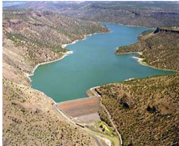
Figure Bowman-1.—A.R. Bowman Dam and Reservoir (Reclamation).
