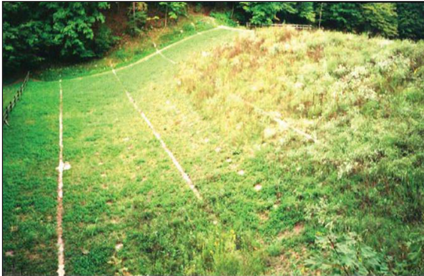
Figure Strahl-7.—Vegetative cover on Strahl Lake Dam overtopping protection (Courtesy of Contech Engineering Solutions, all rights reserved).
