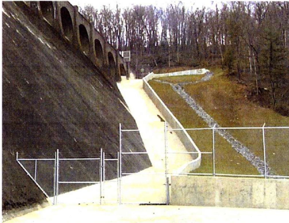
Figure 13-5.—Concrete channel using guide wall to convey overtopping flows (USACE republished in Zaitsoff, 2003).
