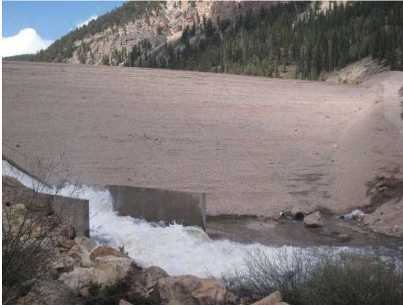
Figure Spring Creek-1.—RCC overtopping protection placed on downstream face of Spring Creek Dam between left abutment groin and right abutment service spillway (shown operating in foreground). (Courtesy of Colorado Department of Natural Resources)
