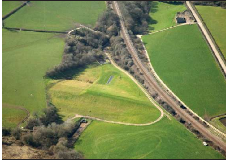
Figure Bruton-1.—Bruton Flood Storage Reservoir embankment prior to new wedge block spillway installation (Courtesy of Pether et al., 2009, all rights reserved).
