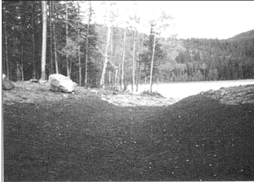
Figure Cottonwood-10.—Completed spillway looking upstream into the reservoir (Reclamation figure republished in Timblin et al., 1988).
