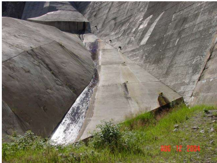
Figure 13-4.—Concrete overtopping protection at downstream toe of dam (Reclamation).
