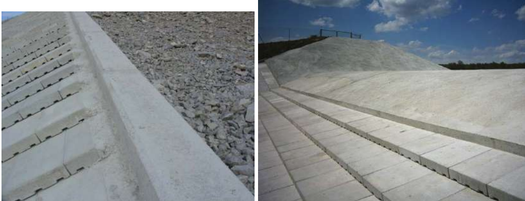
Figure Barriga-13.—View of top caps for the side slope blocks on left and of the completed crest cap on right (courtesy of Morán and Toledo, 2006, all rights reserved).
