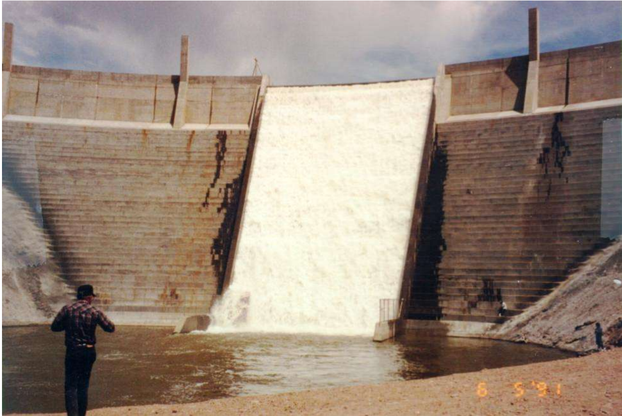
Figure 12-4.—Service spillway flows confined by training walls on stepped downstream face of Santa Cruz Dam (Reclamation).
