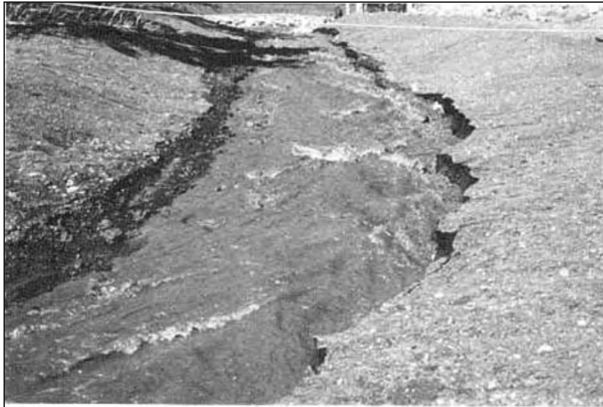
Figure Cottonwood-13.—Flow in the membrane-lined channel during operation. View looking upstream towards the crest with the flat bottom eroded to the edges of the 2:1 side slopes (Reclamation figure republished in Timblin et al., 1988).
