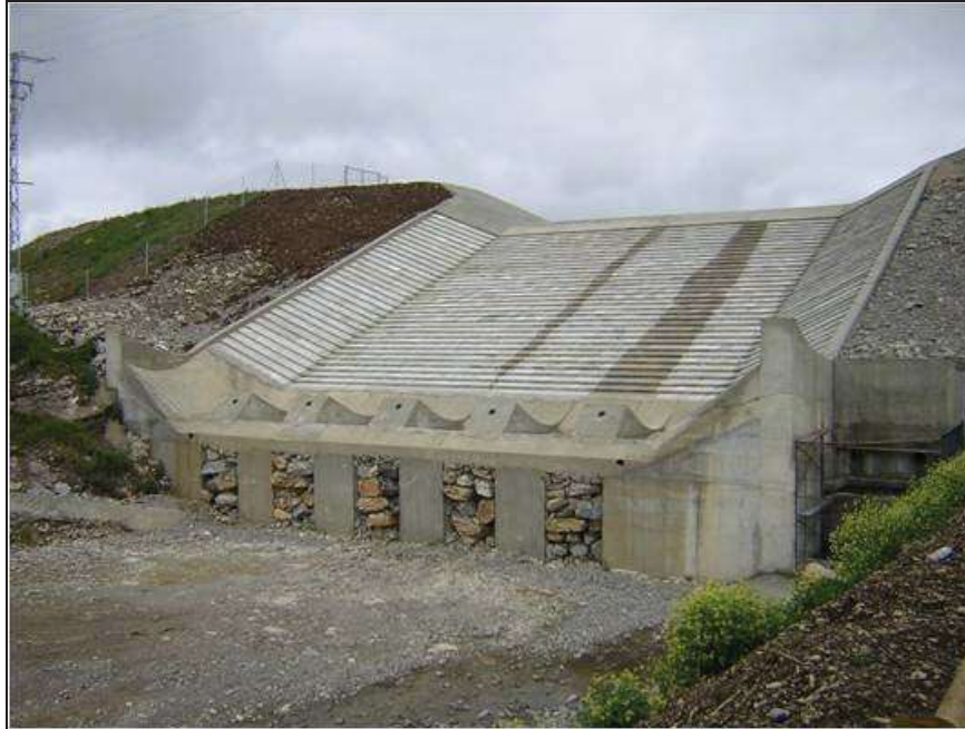
Figure Barriga-14.—Completed spillway prior to operation (courtesy of Morán and Toledo, 2006, all rights reserved).
