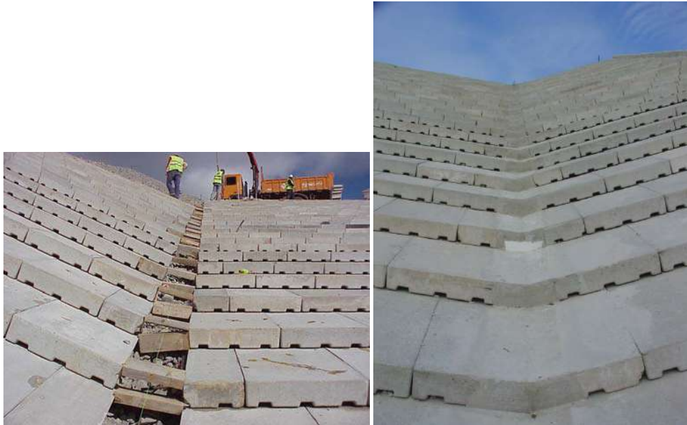
Figure Barriga-12—Views of shimmed joint on left and completed concrete transition on right between invert and side slope (courtesy of Morán and Toledo, 2006, all rights reserved).
