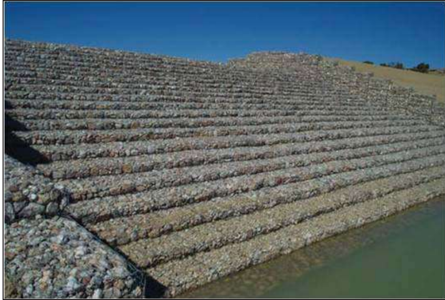
Figure West Cornfield-6.—Completed gabion spillway in 2003 (Courtesy of Maccaferri, Inc., all rights reserved).
