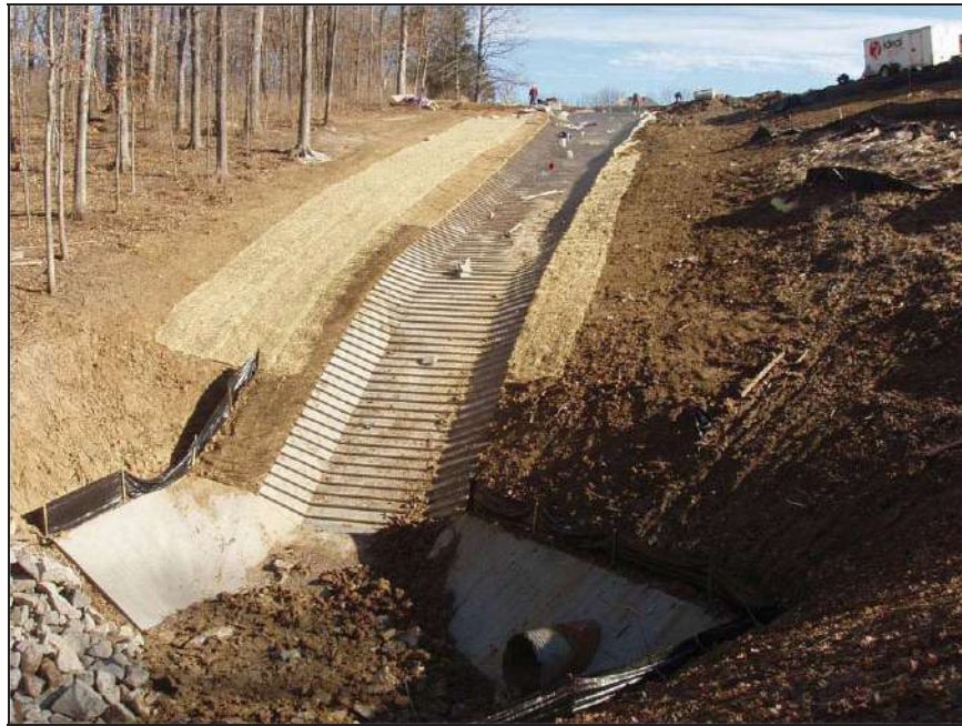
Figure Friendship Village-1. —Overall view of the ArmorWedge auxiliary spillway for the Friendship Village Project nearing completion. The spillway is converging near the top, with three slope changes. The flow will enter an energy dissipating basin shared with the service spillway pipe located to the right in the photo (courtesy of Contech Engineering Solutions, all rights reserved).
