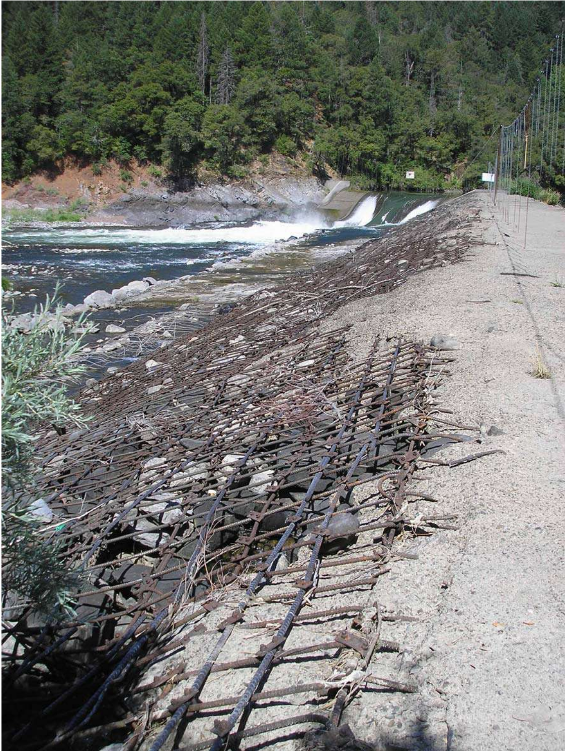
Figure 7-2.—Pit No. 7 Afterbay Dam, looking at downstream face, toward right abutment spillway. Dam crest has been capped with concrete. (Reclamation, 2007, courtesy of Jared Vauk).
