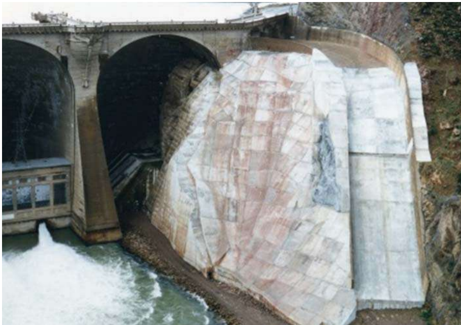
Figure Coolidge-9.—Photo showing finished left spillway concrete overlay and overtopping protection on lower left abutment of dam (Reclamation).
