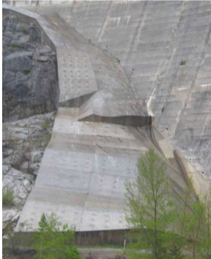
Figure 13-3.—Concrete overtopping protection at downstream toe of dam (Reclamation).
