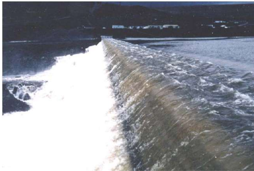
Figure 12-2.—RCC buttress for Camp Dyer Diversion Dam during overtopping in January 1993 (Reclamation).
