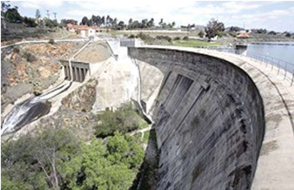
Figure Sweetwater-1.—Sweetwater Dam (Courtesy, Sweetwater Authority, all rights reserved).
