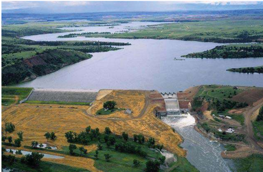
Figure Tongue-2.—Aerial view of Tongue River Dam in Montana, with service spillway shown at right and RCC overtopping protection shown at left. (Courtesy of Montana DNRC).
