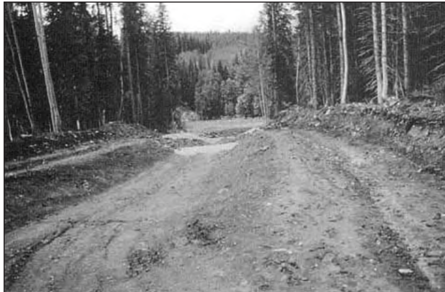
Figure Cottonwood-5.—Preparation of subgrade before geomembrane liner installation in spillway (Reclamation figure republished in Timblin et al., 1988).
