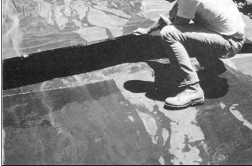
Figure Cottonwood-18.—The overlapped seams were inspected after the test. The geomembrane liner and the earthen materials were all dry under the overlapped areas (Reclamation figure republished in Timblin et al., 1988).
