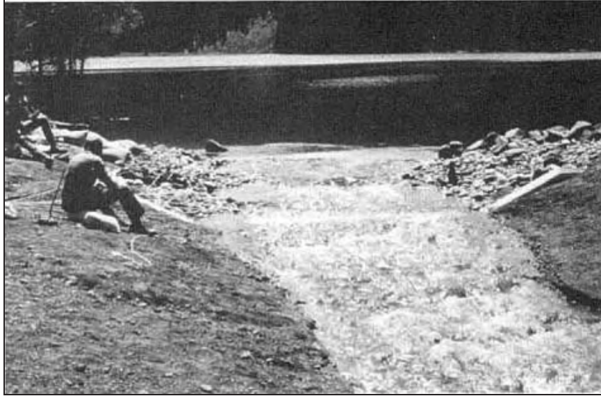
Figure Cottonwood-12.—Flow over spillway crest during operational test. The flow was estimated to be 21 to 25 ft 3 /s at a maximum velocity of 19 to 26 ft/s (Reclamation figure republished in Timblin et al., 1988).
