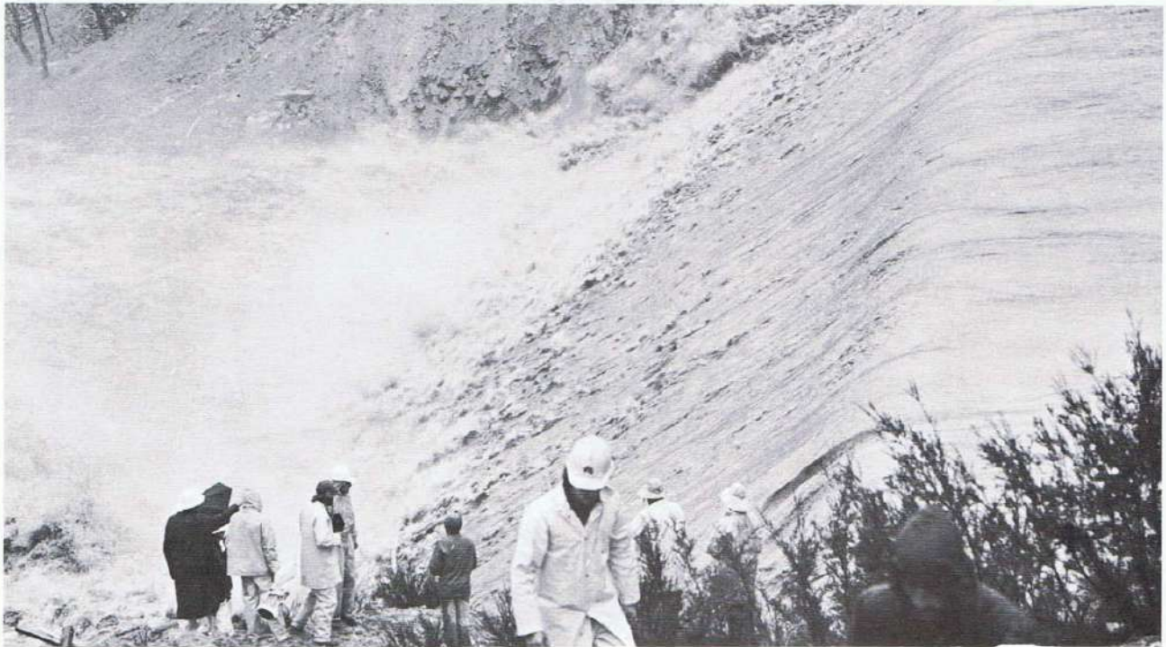
Figure Googong-1.—Overtopping of Googong Dam during construction, October 1976. (Courtesy of Engineering Heritage Canberra, all rights reserved).
