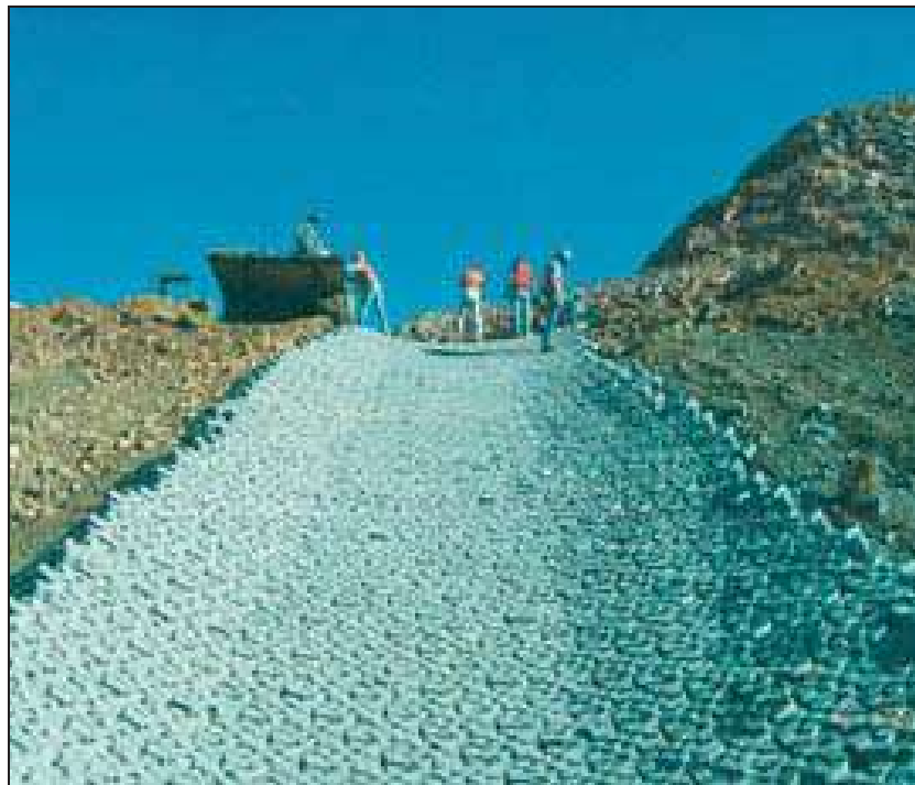
Figure Richmond Hill-5.—Nearly completed downchute constructed of interlocking ACBs. The upstream end of the Tri-lock mat was not anchored as it would be in today's installations. The sides of the mat were anchored into the overburden stockpile cover material (Courtesy of Jacobs et al., 2004, all rights reserved).
