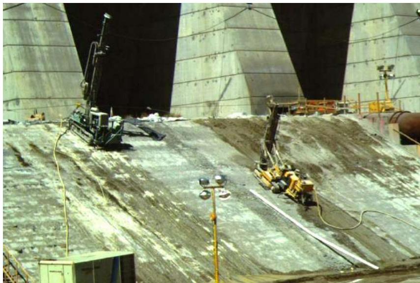
Figure 12-6.—Mechanical anchors being installed through the RCC toe block into the foundation for Pueblo Dam spillway, to improve sliding resistance (Reclamation).
