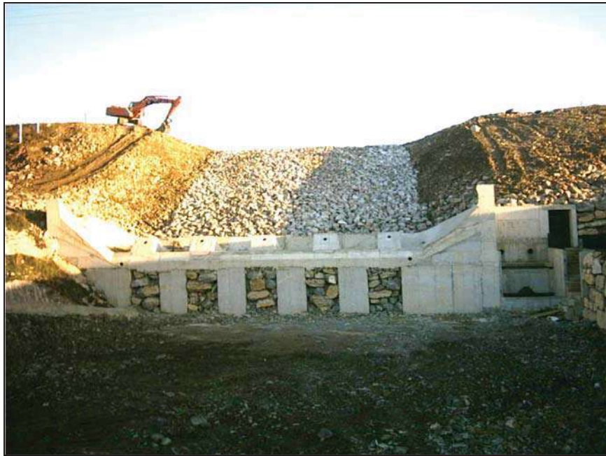
Figure Barriga-7.—Completed flip bucket toe block and drainage with initial grading for block spillway (courtesy of Morán and Toledo, 2006, all rights reserved).
