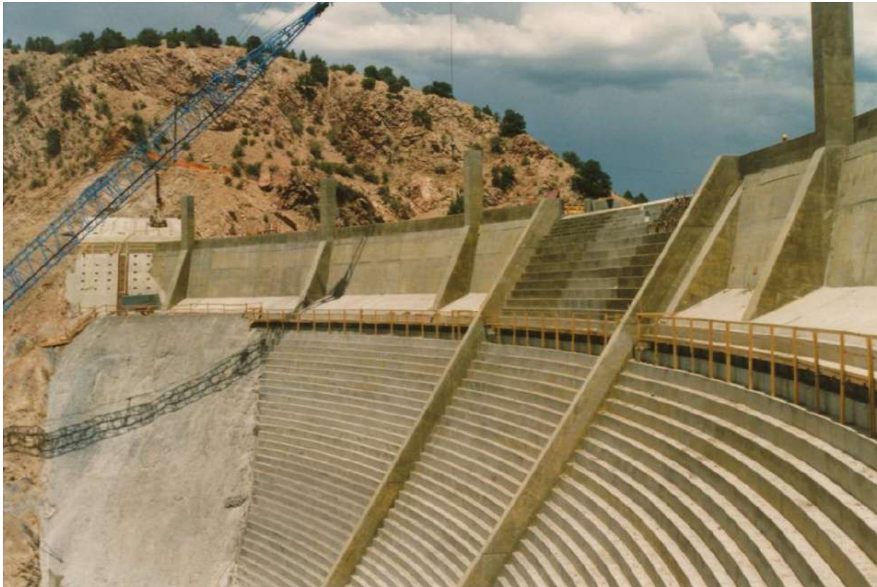
Figure 12-3.—Concrete overtopping protection for Santa Cruz Dam in New Mexico. Splitter piers were provided for overtopping of the entire dam crest (Reclamation).
