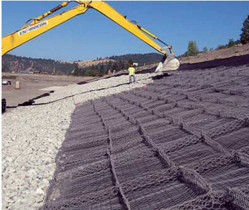
Figure 5-13.—Gabion baskets on slope being filled with rock, Milltown Dam Removal project in Milltown, Montana (Courtesy of Envirocon, all rights reserved).
