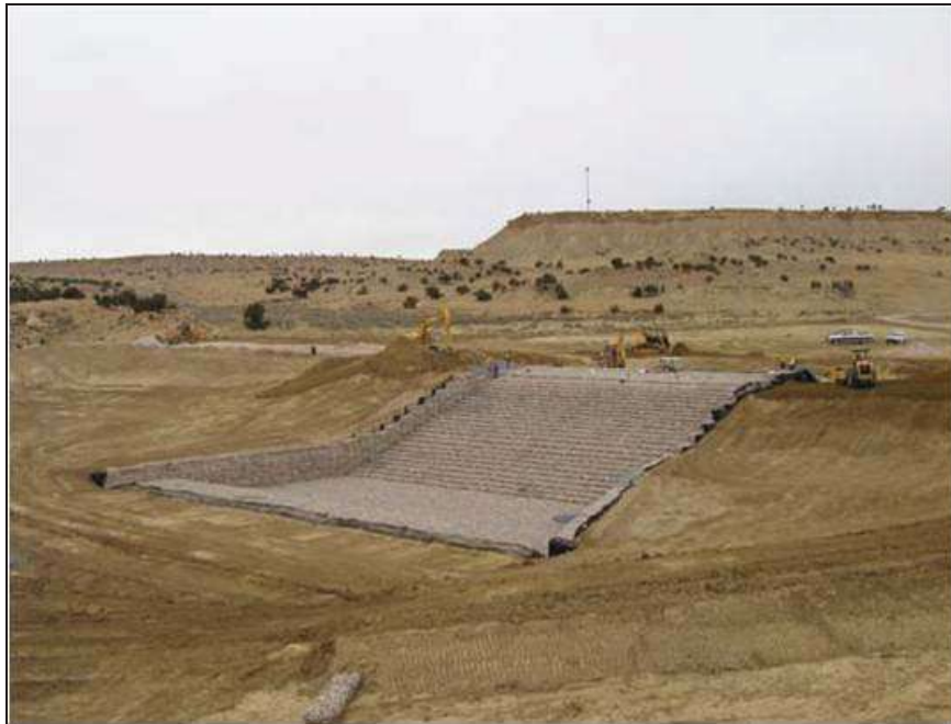
Figure West Cornfield-5.—Construction nearing completion (Courtesy of Maccaferri, Inc., all rights reserved).
