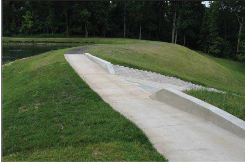
Figure Friendship Village-3.—Finished crest forming a sidewalk for the lake and the top of the ArmorWedge block spillway (courtesy of Contech Engineering Solutions, all rights reserved).
