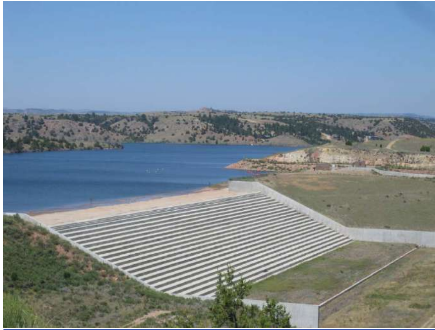
Figure Tongue-1.—Closeup view of RCC overtopping protection constructed on the downstream face of Tongue River Dam. (Courtesy of Montana Department of Natural Resources and Conservation [DNRC]).
