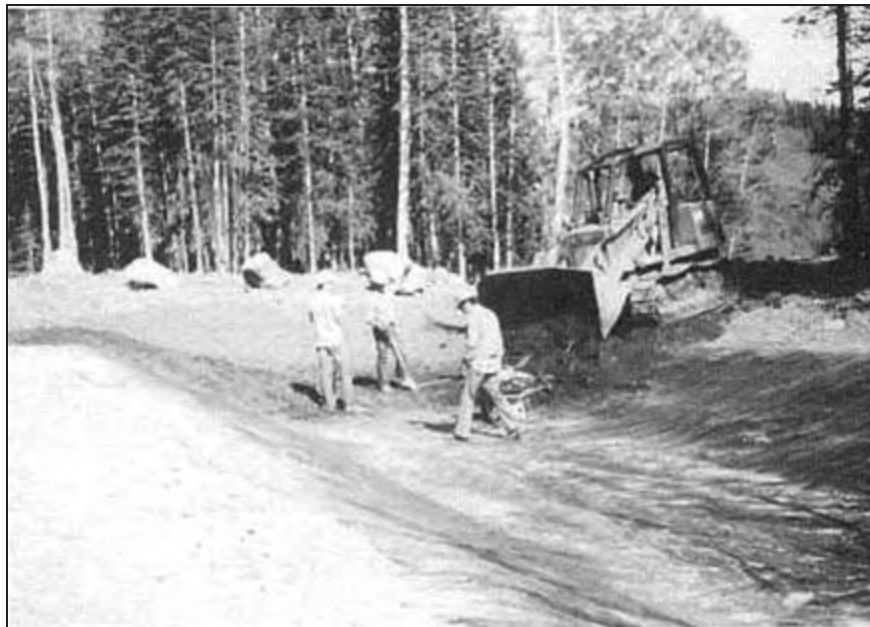
Figure Cottonwood-9.—Placement of soil cover to protect geomembrane liner from the elements and mechanical damage (Reclamation figure republished in Timblin et al., 1988).
