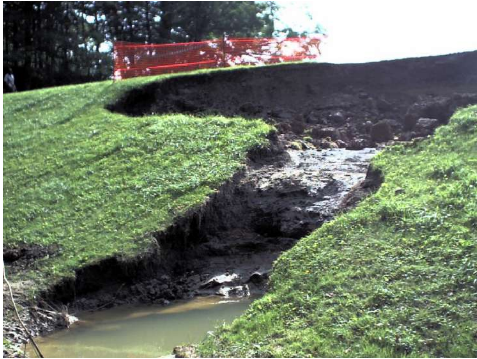
Figure 6-4.—Virginia Kendall Dam in Ohio after 3 hours of overtopping flow (Reclamation, 2003, courtesy of David Gillette).
