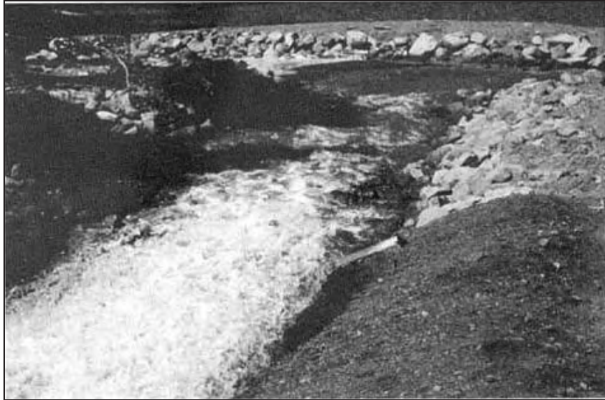
Figure Cottonwood-14.—Flow at the downstream end of the spillway as it entered the riprap basin (Reclamation figure republished in Timblin et al., 1988).
