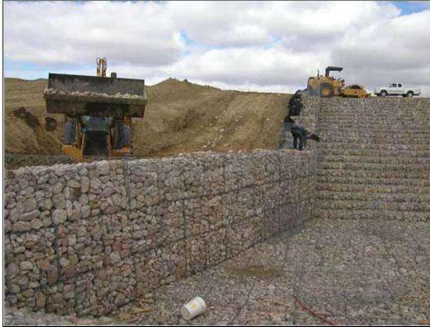
Figure West Cornfield-4.—Constructing stilling basin retaining walls (Courtesy of Maccaferri, Inc., all rights reserved).
