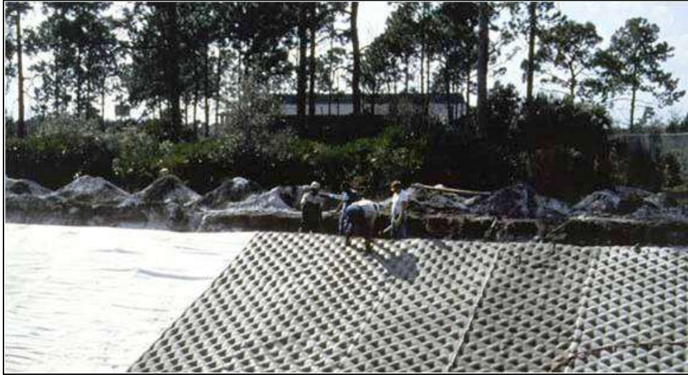
Figure 9-7.—Fabric forms being filled with fine aggregate concrete. (Courtesy of Donnelly Fabricators, all rights reserved).
