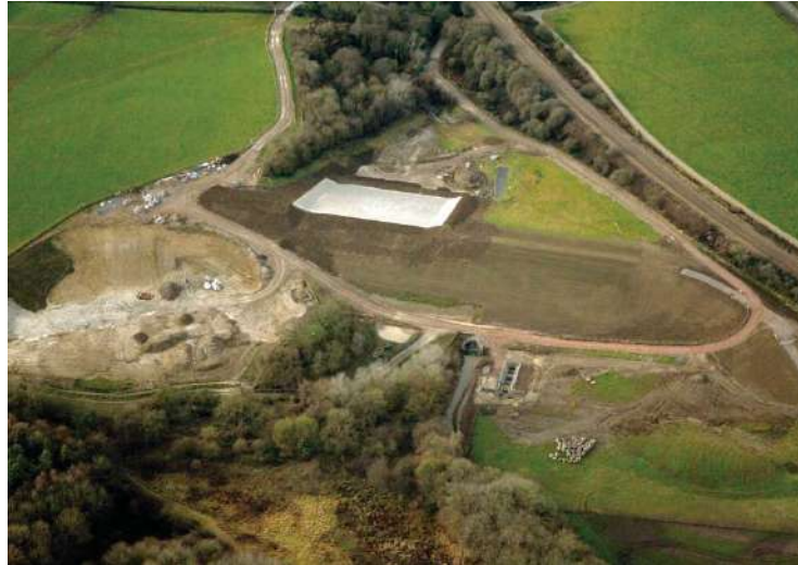
Figure Bruton- .—Aerial view of completed project.
