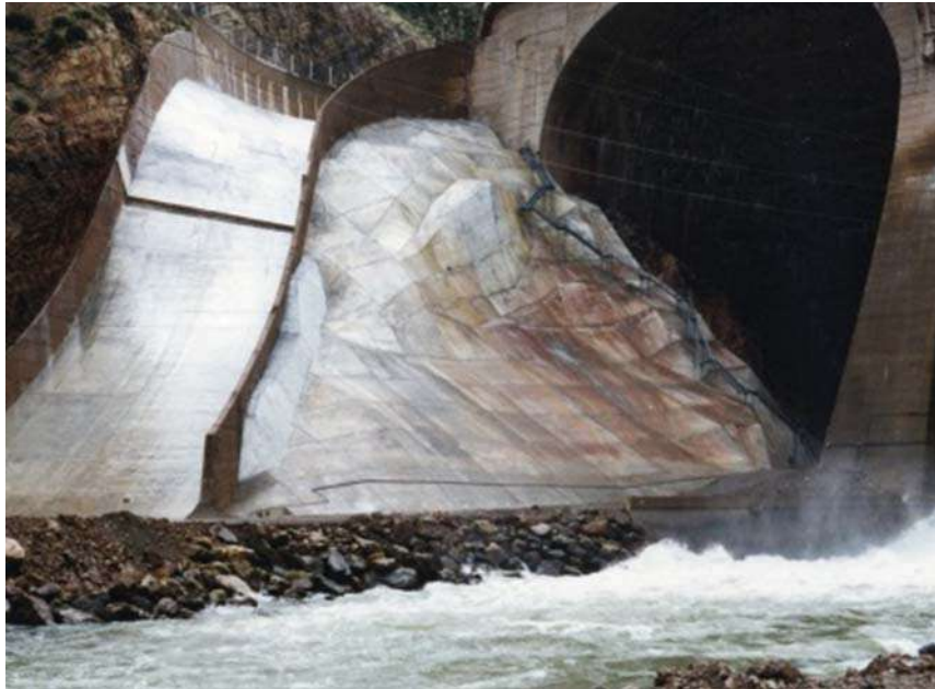
Figure Coolidge-8.—Photo showing finished right spillway concrete overlay and overtopping protection on lower right abutment of dam (Reclamation).
