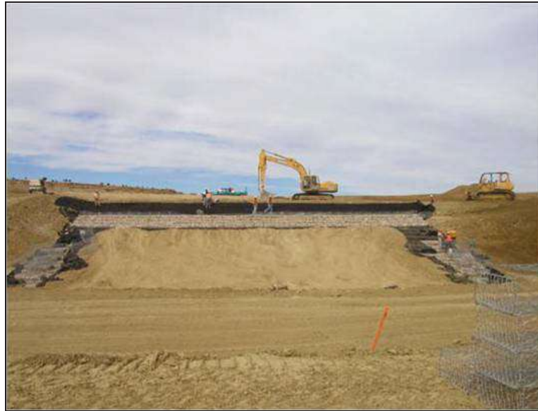
Figure West Cornfield-2.—Dam beginning construction (Courtesy of Maccaferri, Inc., all rights reserved).
