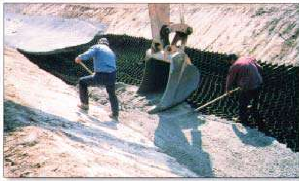
Figure Empire-1– Installation of the GeoWeb CCS with concrete infill for Empire Landfill (courtesy of Presto Geosystems, all rights reserved).
