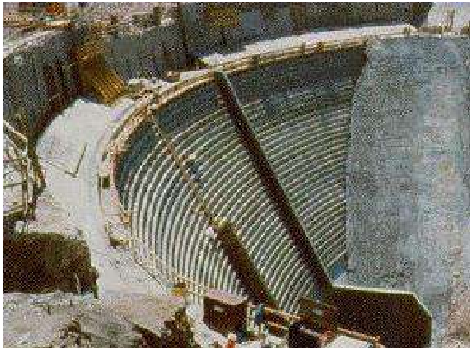
Figure 12-8.—RCC placements followed curvature of existing arch dam, Santa Cruz Dam (Reclamation).
