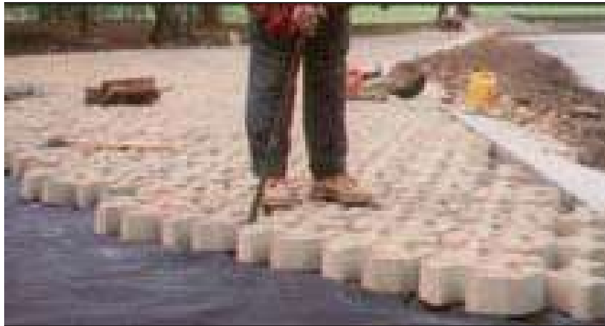
Figure Richmond Hill-3.—Installation of the 40-in-thick ACBs directly over the geotextile prior to backfilling the open space between blocks with topsoil (Courtesy of Jacobs et al., 2004, all rights reserved).
