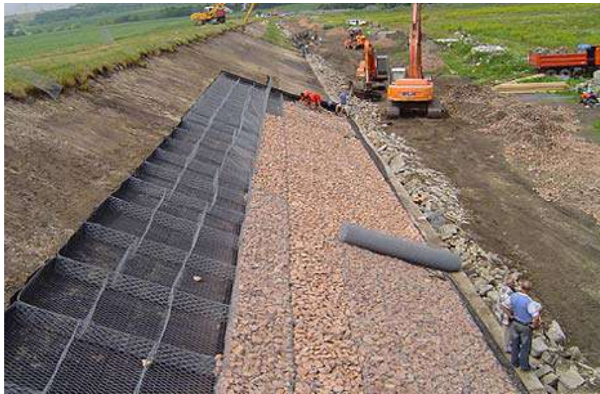
Figure 5-6.—Gabion erosion protection on slope of embankment. Zamoly Reservoir, Hungary (Courtesy of Pannon Gabion Kft, all rights reserved).
