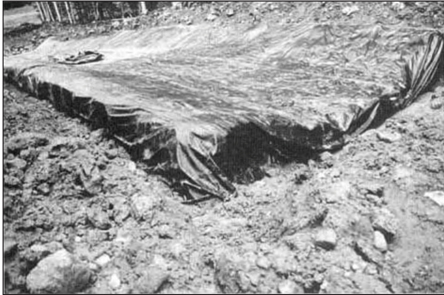
Figure Cottonwood-6.—Section of geomembrane liner installed in spillway before backfilling and compacting anchor trenches (Reclamation figure republished in Timblin et al., 1988).
