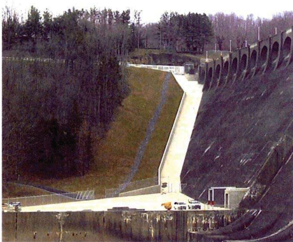
Figure Tygart-1.—Concrete Paving and Channel Along Downstream Right Abutment (Courtesy of USACE).
