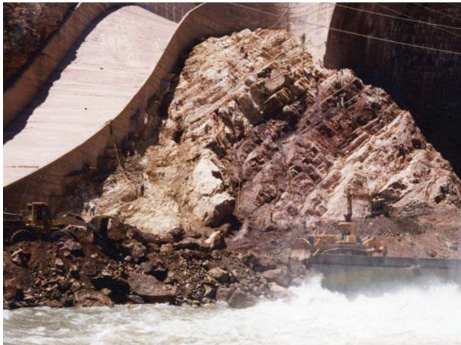
Figure Coolidge-7. —Photo of lower right abutment of dam and right spillway chute. Right abutment overtopping and excavation and cleanup in progress (Reclamation).
