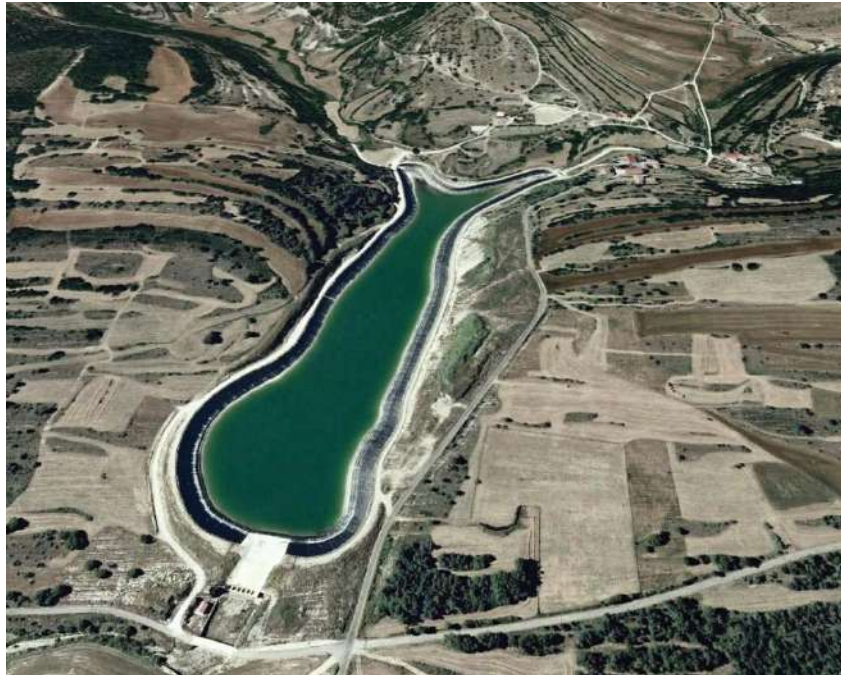
Figure Barriga-1. —Overall view of the completed Barriga Dam water storage project showing the membrane-lined reservoir and stepped block spillway in the lower left hand corner (courtesy of Rafael Morán, all rights reserved).
