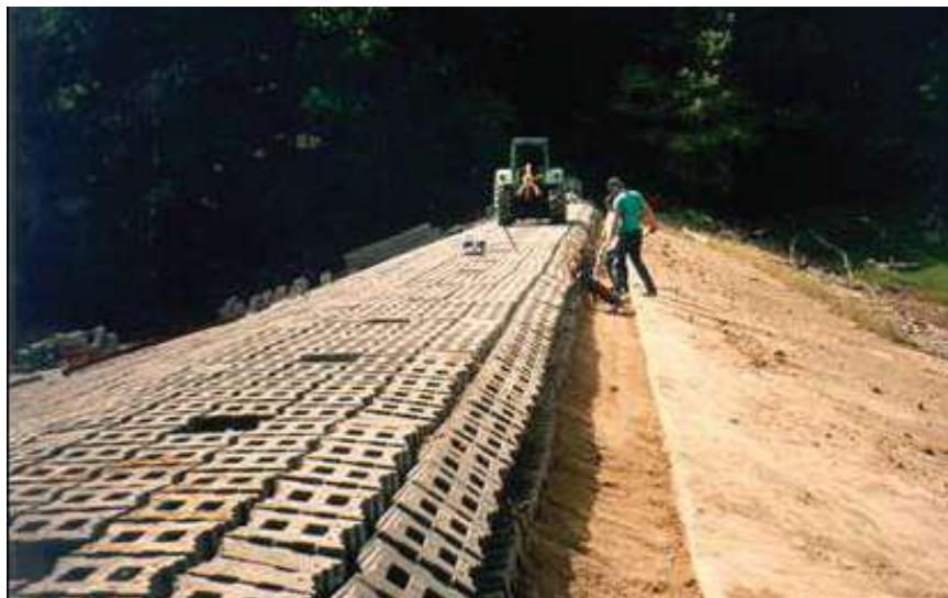
Figure Strahl-5.—View of the upstream trench used to anchor the system at the crest (Courtesy of Contech Engineering Solutions, all rights reserved).
