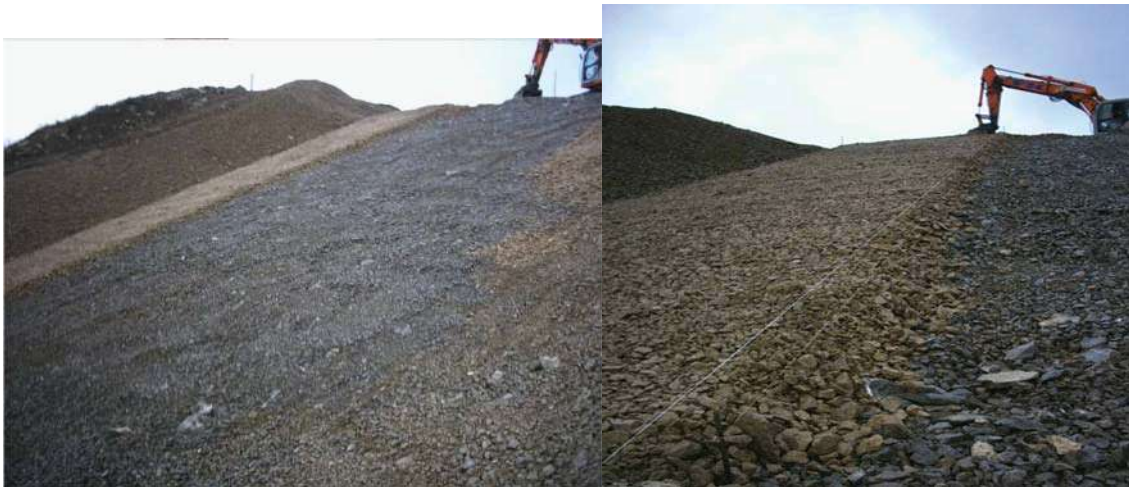
Figure Barriga-8.—Views of the two filter-compatible gravel layers beneath the block system, (a) top bedding layer (left) and (b) bottom drainage layer (right) (courtesy of Morán and Toledo, 2006, all rights reserved).
