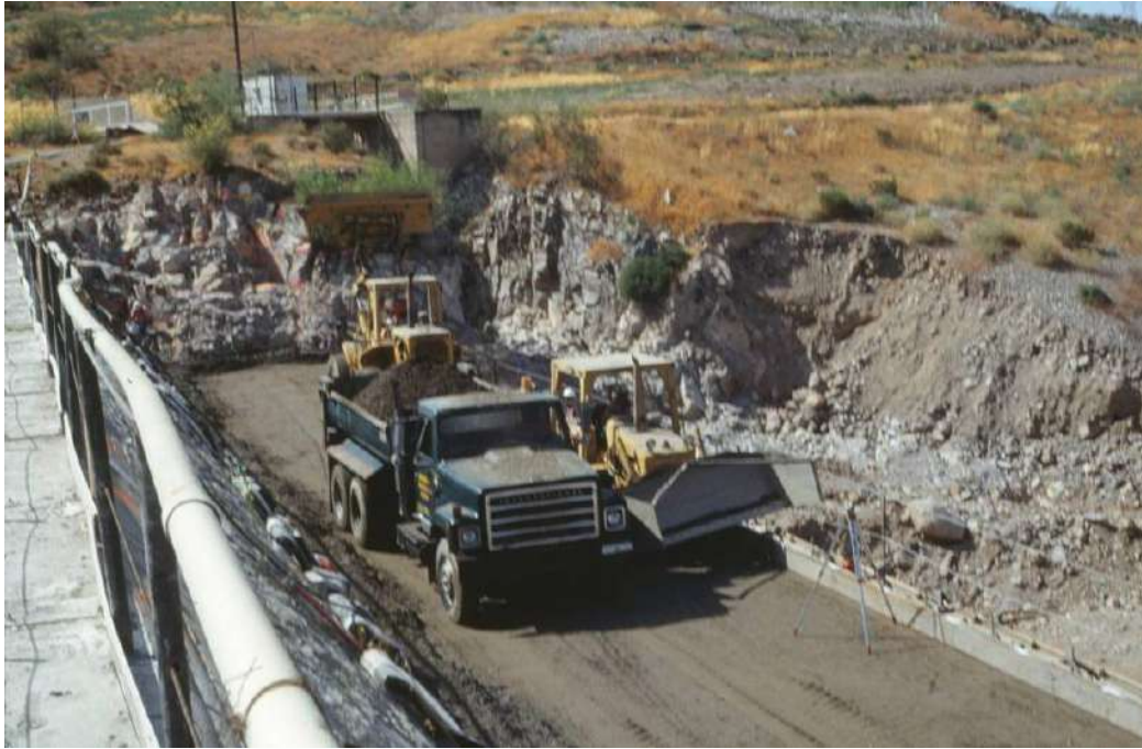
Figure 12-7.—RCC buttress being constructed at downstream face of Camp Dyer Diversion Dam. Width of RCC placement is sufficient for passing construction equipment. Note flat drains on contact surface between dam and buttress. (Reclamation)
