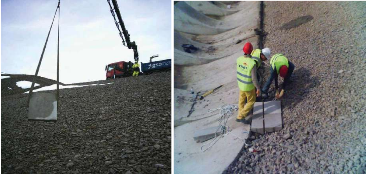
Figure Barriga-9.—Crane passing down a block and placement of the first block at the flip bucket (courtesy of Morán and Toledo, 2006, all rights reserved).
