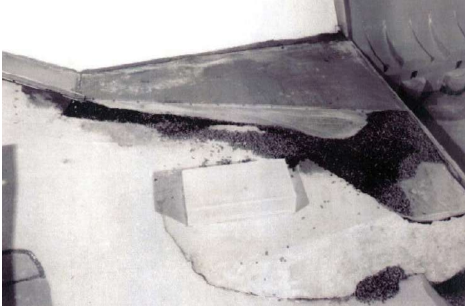
Figure Tygart-3.—Type 2 design, damage resulting from PMF flow for 1 hour (Courtesy of USACE, 1999).
