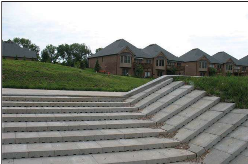
Figure Friendship Village-4.—View looking upstream toward the Friendship Village community and the finished top of spillway (courtesy of Contech Engineering Solutions, all rights reserved).
