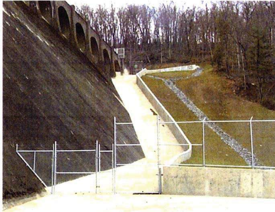
Figure Tygart-2.—Concrete Paving and Channel Along Downstream Left Abutment (Courtesy of USACE)
