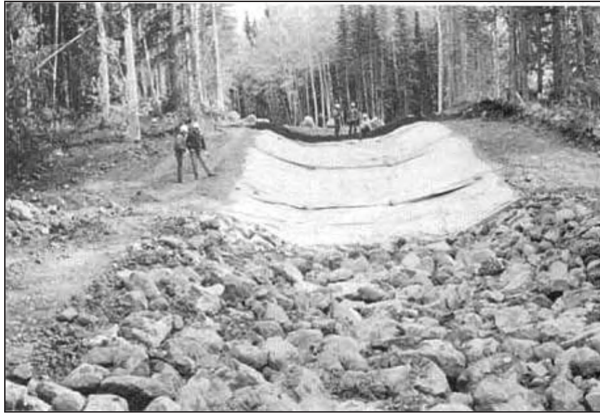
Figure Cottonwood-8.—Looking upstream at geomembrane-lined spillway (Reclamation figure republished in Timblin et al., 1988).
