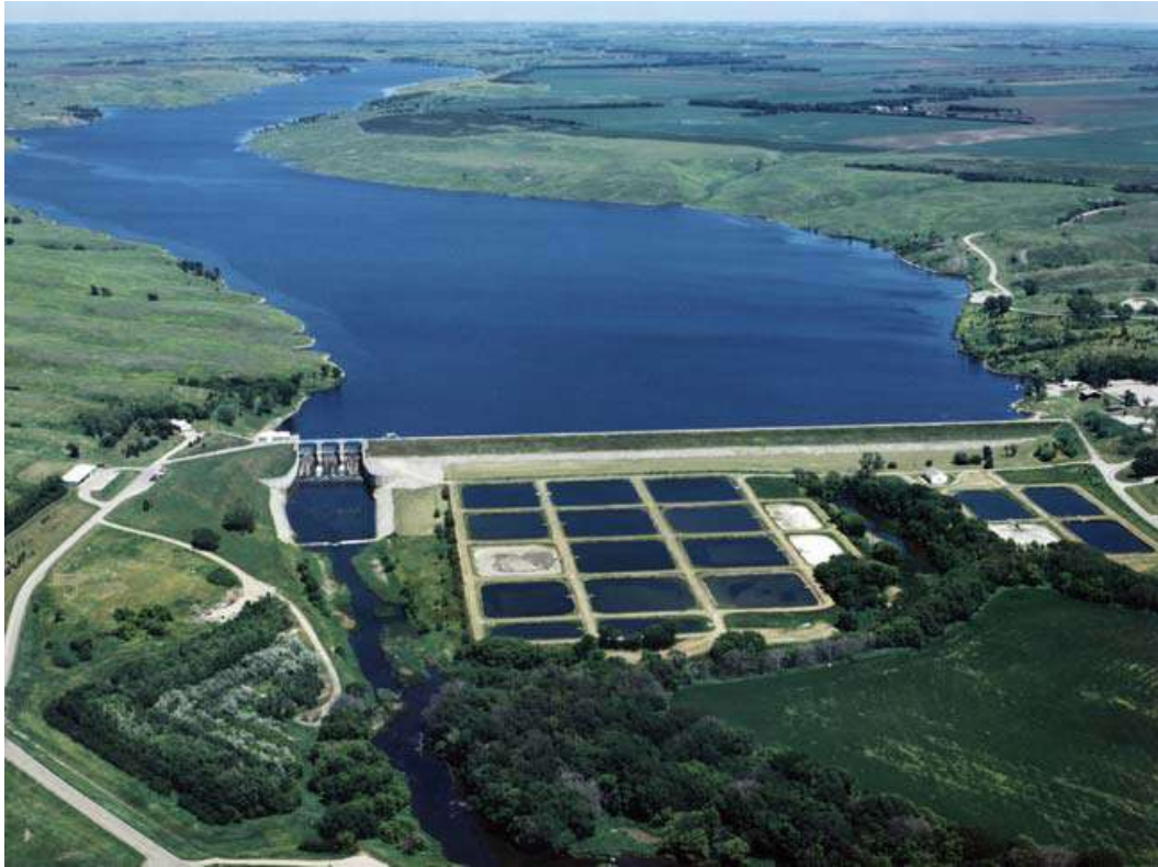
Figure Baldhill-1.—Baldhill Dam, with service spillway at the right end of the dam (looking downstream) and the uncontrolled auxiliary spillway on the downstream face of the dam (Courtesy of USACE).
