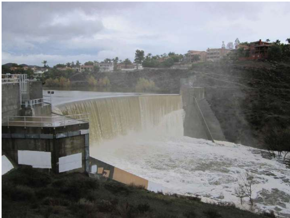
Figure Railroad Canyon-1.—Railroad Canyon Dam during flood event in 2010 (Courtesy of Elsinore Valley Municipal Water District).
