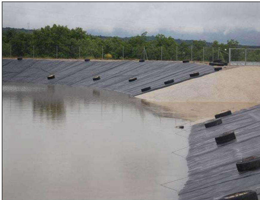
Figure Barriga-17.—View of the lined reservoir and approach conditions into the completed spillway (courtesy of Morán and Toledo, 2006, all rights reserved).
