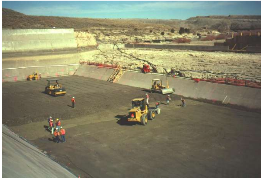
Figure 12-5.—RCC buttress construction within the original spillway plunge pool for Pueblo Dam in Colorado (Reclamation).
