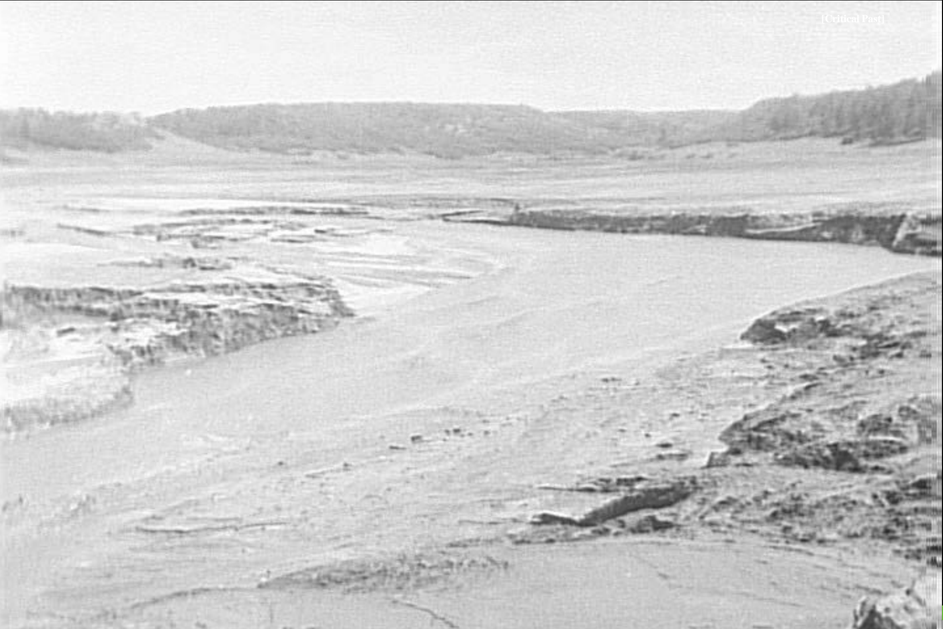
Castlewood Dam Failure, 1933
