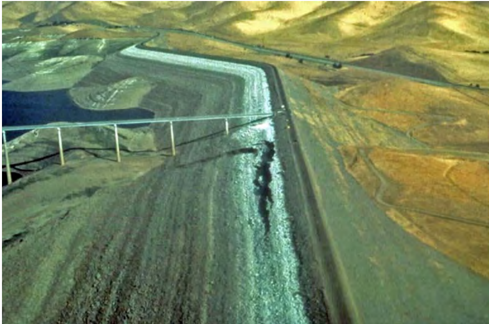
Figure 4.5.7-1. B.F. Sisk Dam (near Los Banos, California). View showing upstream slope failure during reservoir drawdown.
