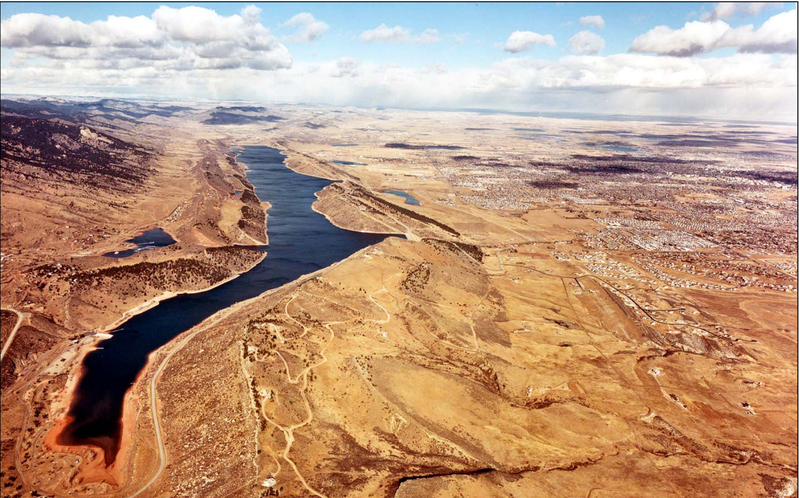
Horsetooth Reservoir Dam (near Fort Collins, Colorado).
