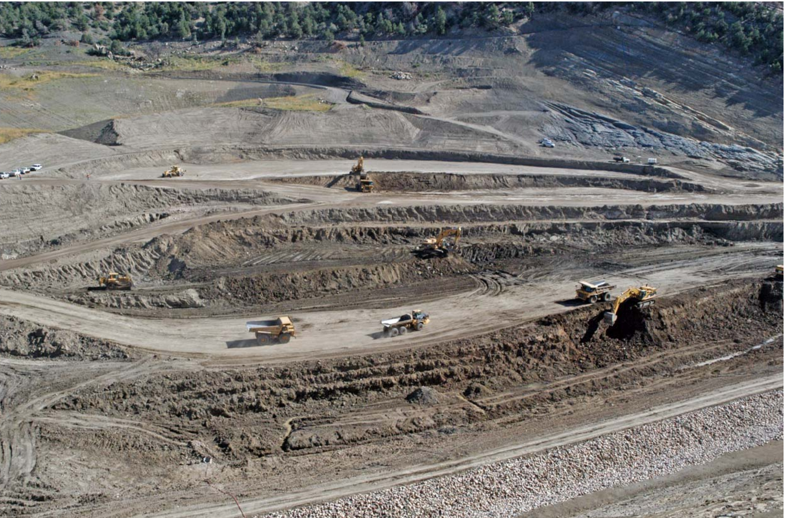
Ridges Basin Dam (near Durango, Colorado). View showing foundation excavation during construction.
