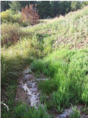
Photo 2. Seepage exiting dam face
