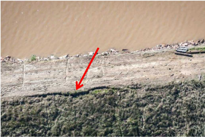
Photo 1. Severe longitudinal cracks in downstream slope
