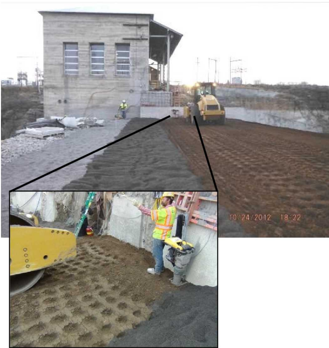
Photo 2. Core Compaction. Note compacting in paths parallel to dam axis and the hand tamper in photo that will be used to compact zone immediately next to wall.
