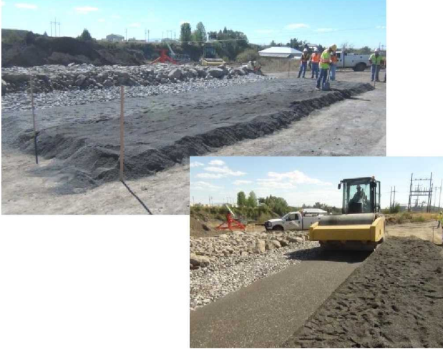
Photo 3. Test Pad for Granular Filter Materials
