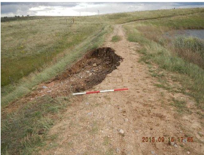
Photo 3. Slope failure on downstream slope
