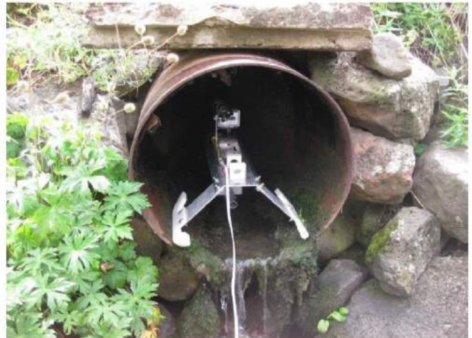
Photo 3: Manually operated CCTV sled. 3
