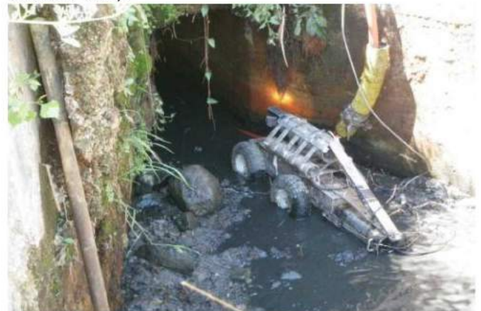
Photo 2: ROV entering a conduit for inspection.
