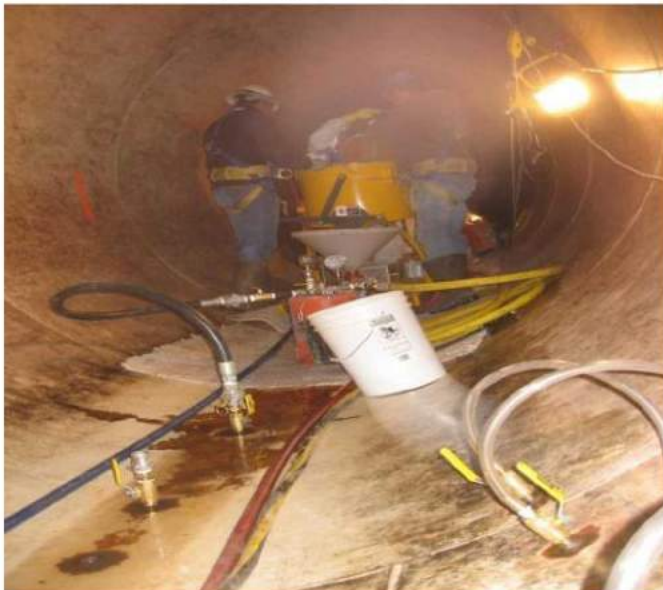
Photo 9: Injection grouting voided encasement behind steel liner.
