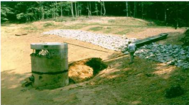
Photo 1: Sinkhole around a spillway riser 2
