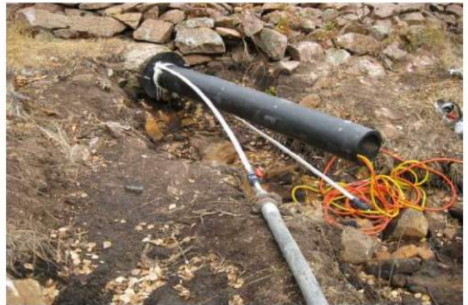
Photo 10: Grouting HDPE liner pipe. 3
