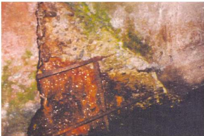
Photo 4: Spalled concrete inside a conduit. 2
