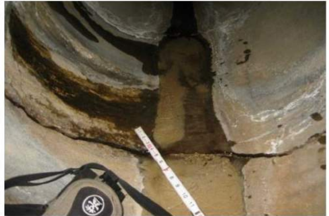
Photo 5: Crack in precast concrete conduit.
