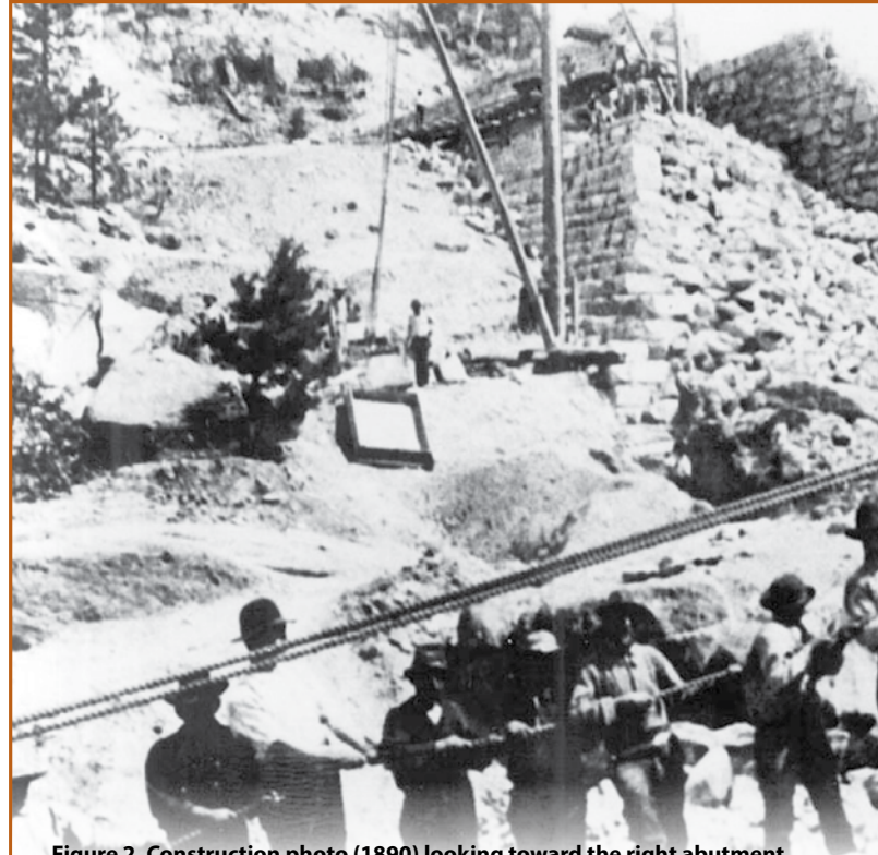
Figure 2. Construction photo (1890) looking toward the right abutment (Photo Courtesy of the Denver Public Library, Western History Collection)
