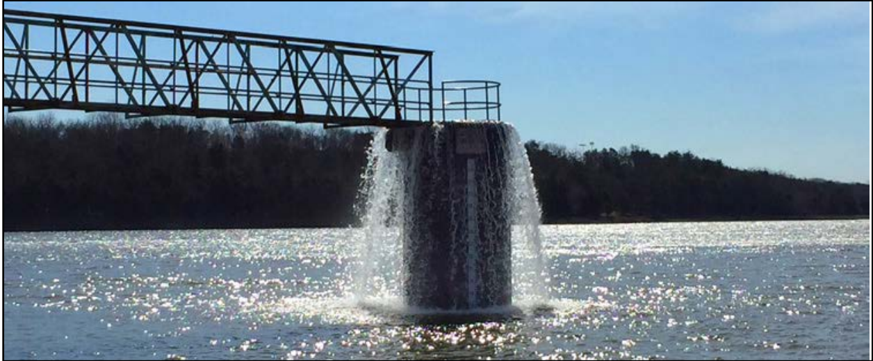
Figure 14: Existing Reservoir Refill Pumping Operations through Inlet Control Tower at Beaverdam Creek Dam
