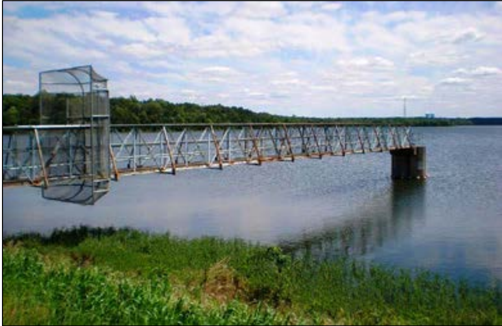
Figure 11: Existing Access Bridge and Security Gate at Beaverdam Creek Dam to be Removed
