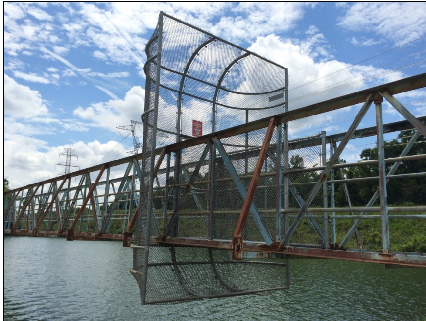
Figure 12: Close-up of the Existing Security Gate
