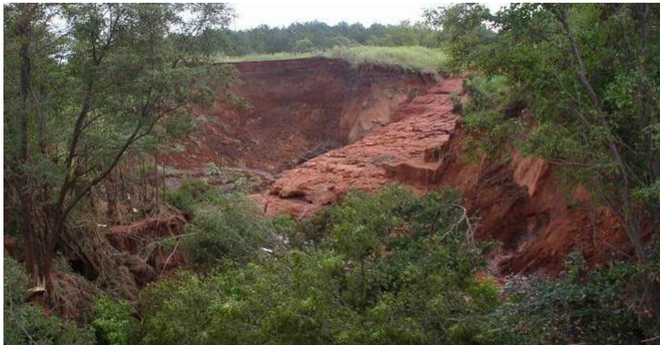
Figure 4 Eroded Auxiliary Spillway taken from Road
