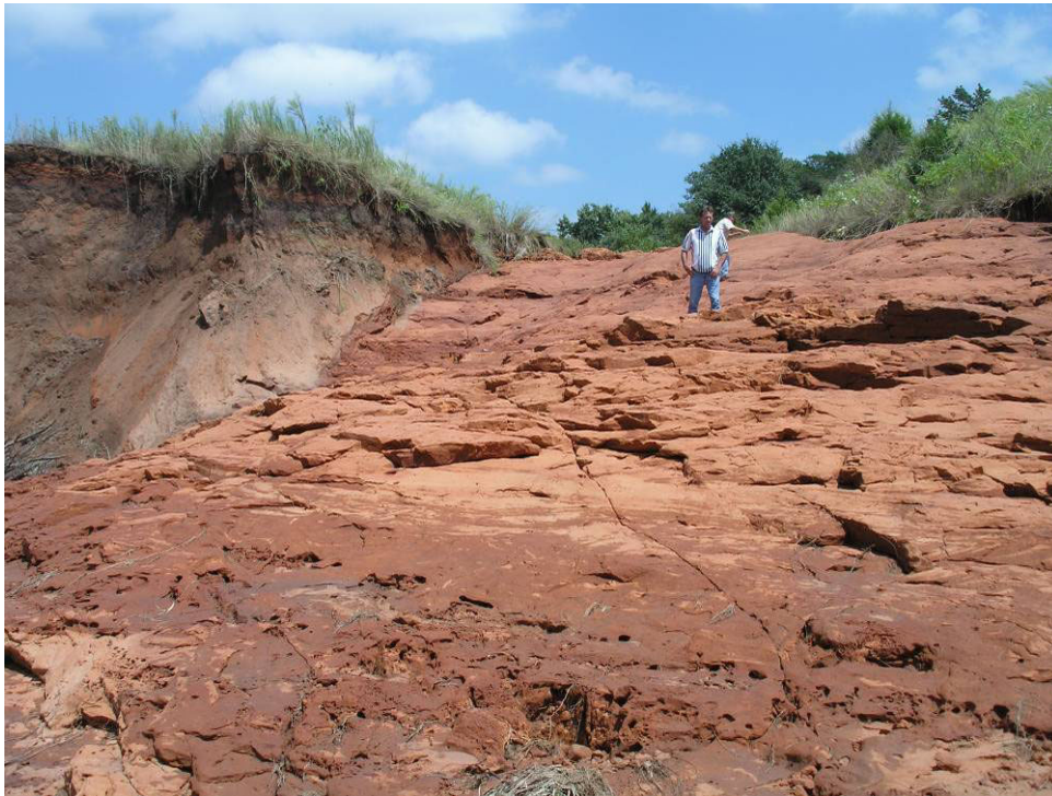
Figure 6 Exposed bedrock in ASW sloping toward dam
