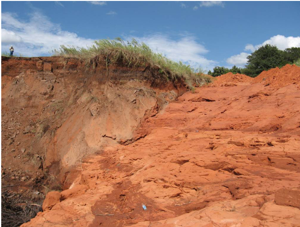
Figure 10 Headcut advance into abutment and embankment groin
