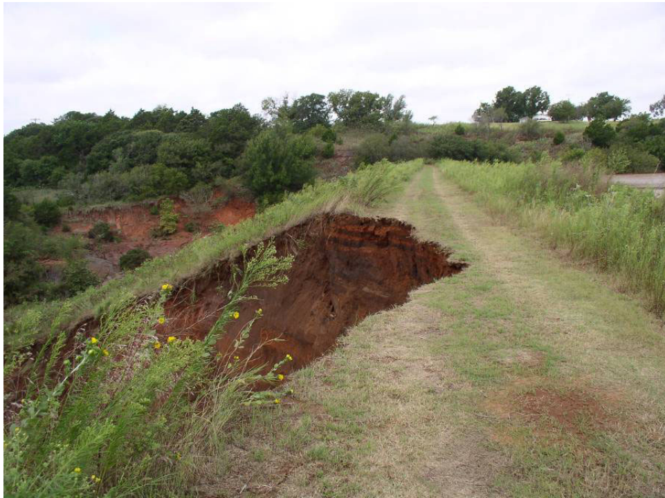
Figure 3 Crest of Dam
