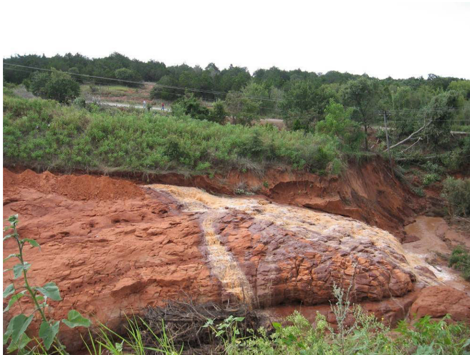
Figure 8 Near vertical outfall running entire length of ASW outlet channel Note: Uncontrolled pumped discharge attempting to flow towards the dam
