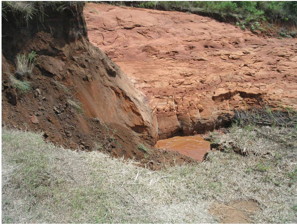
Figure 7 Near vertical outfall of over 10 feet at groin of dam and abutment
