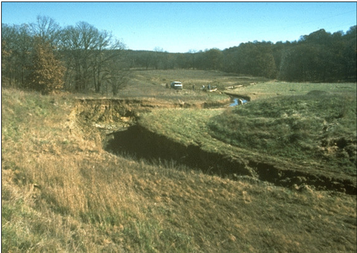
Figure 3. Twin Caney Site 17-3 Kansan in October 1986 provides an extreme case of headcutting when breaching of the spillway was initiated by a roadway paralleling the flow. The flow and stress concentrated in the unvegetated roadway tire tracks on the 10 percent exit channel slope resulting in the development of an overfall. Once formed this overfall moved both upstream and downstream along the lines of flow concentration formed by the tire tracks. Vegetated areas outside of the area of the roadway were undamaged.
