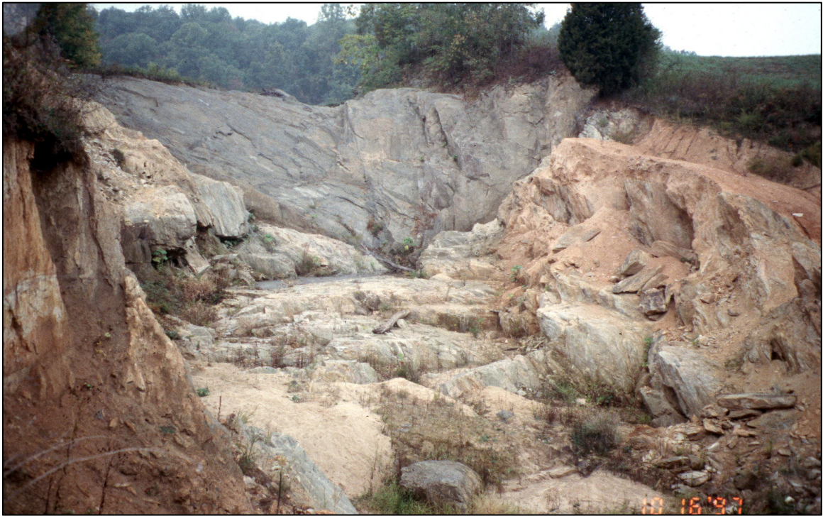
Figure 7. Photos of White Oak Dam auxiliary spillway looking downstream (top) & upstream (bottom) after June 27, 1995 flood when 21 inches of rain fell in less than 18 hours.
