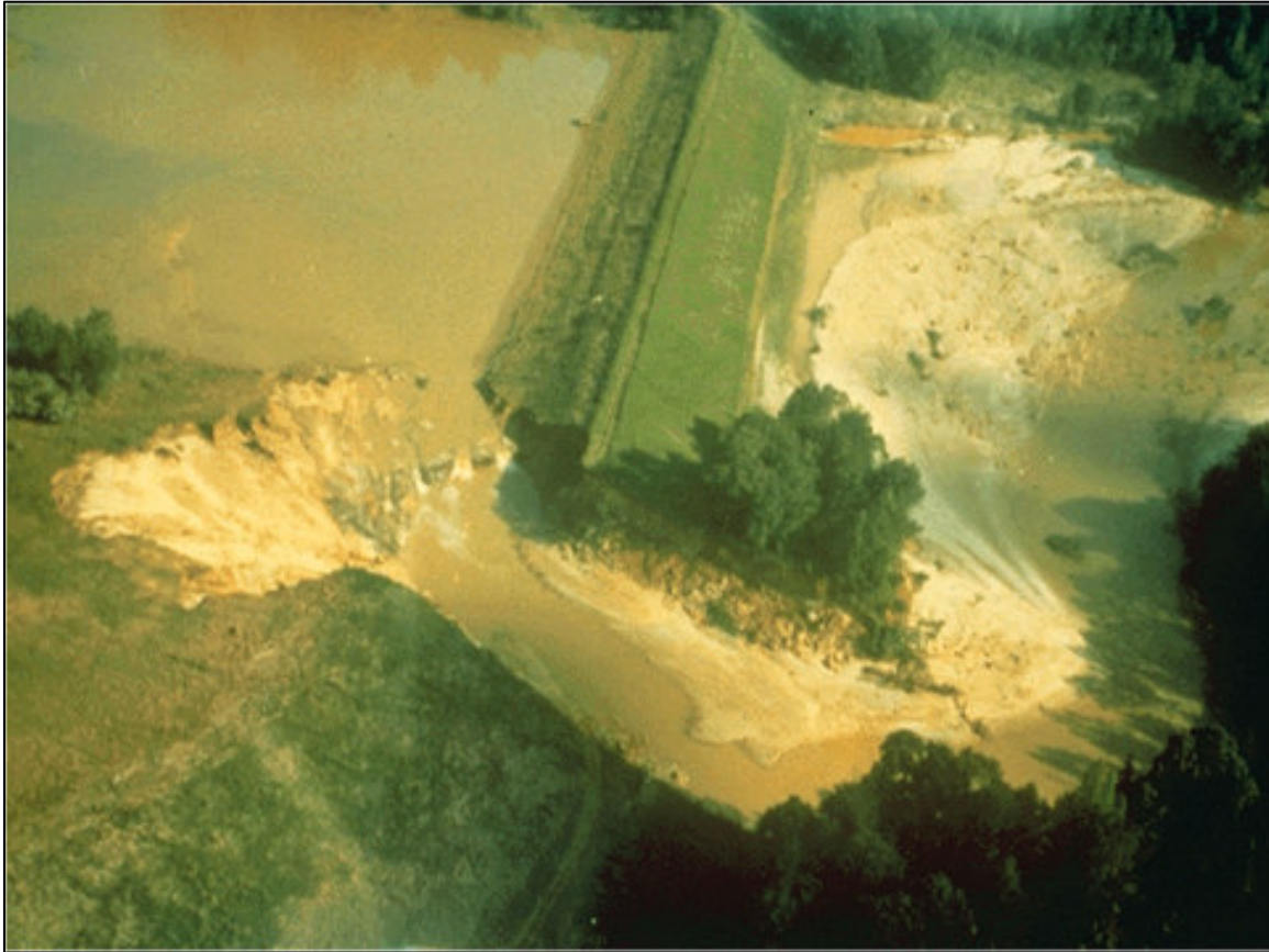
Figure 6. Black Creek Site 53 following breach of auxiliary spillway (Temple, 1989).
