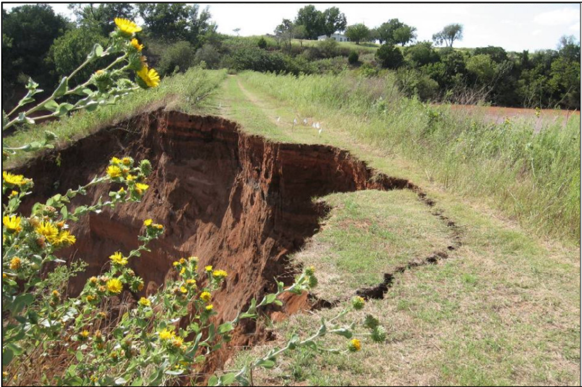
Figure 8. Photographs showing the flow path and erosion in the downstream slope of Sugar Creek Dam L-44 located in Caddo County, Oklahoma following Tropical Depression Erin on August 19, 2007.
