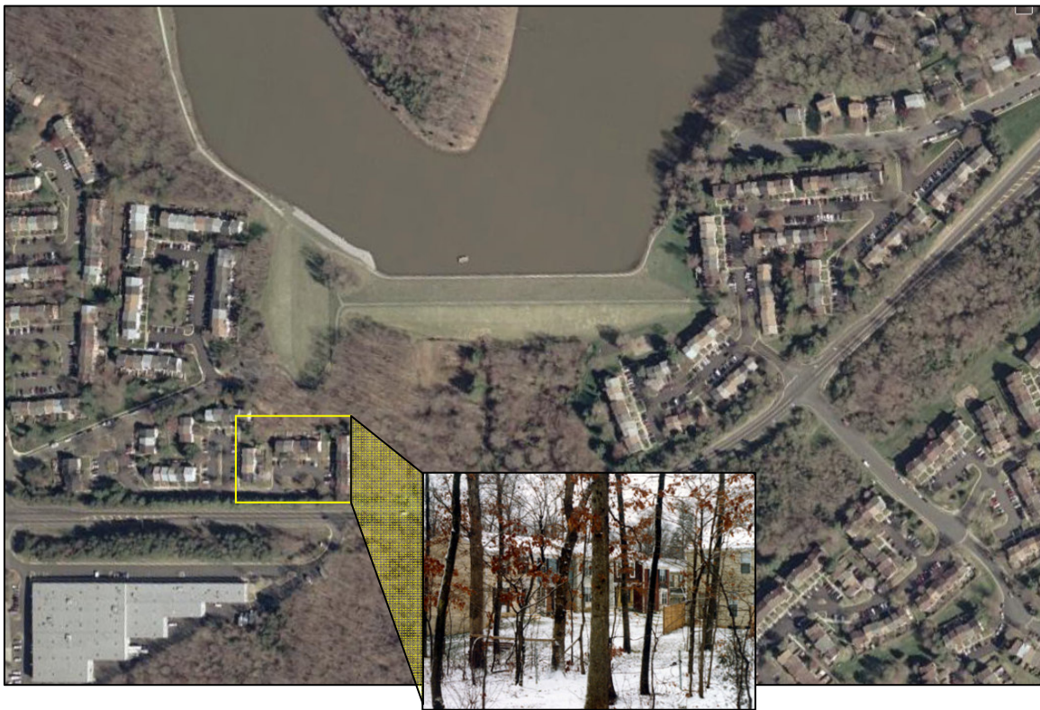
Figure 9. Aerial photos of Pohick Dam No. 4 showing intense urban development within watershed and immediately downstream of the dam and auxiliary spillway.
