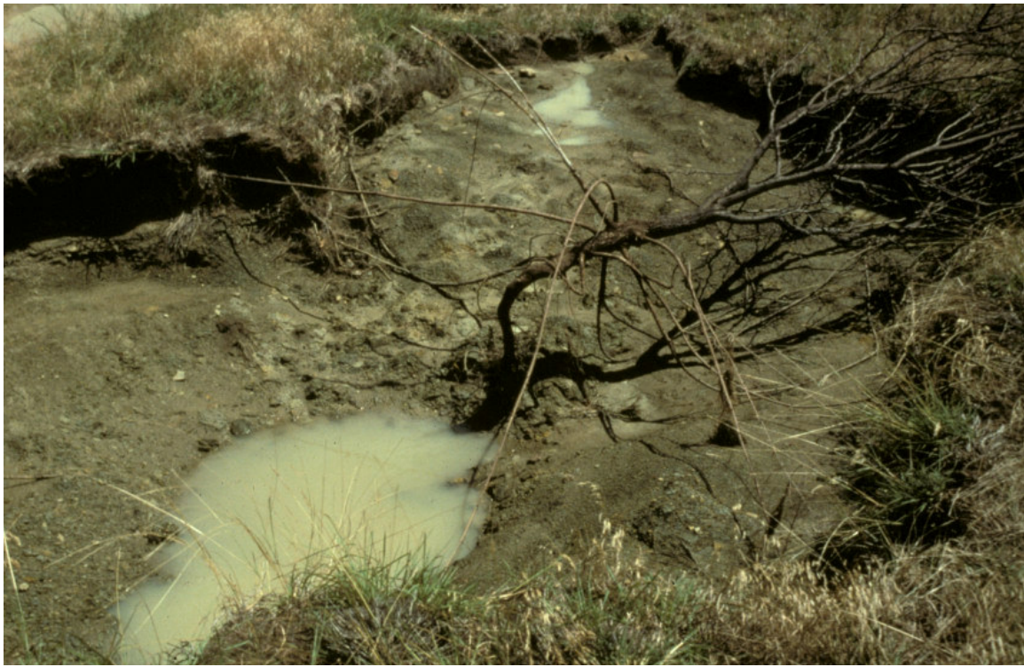
Figure 4. Example of a discontinuity (small tree) in an auxiliary spillway. Flow concentrates around the discontinuity causing higher stresses and local erosion of the grass cover.
