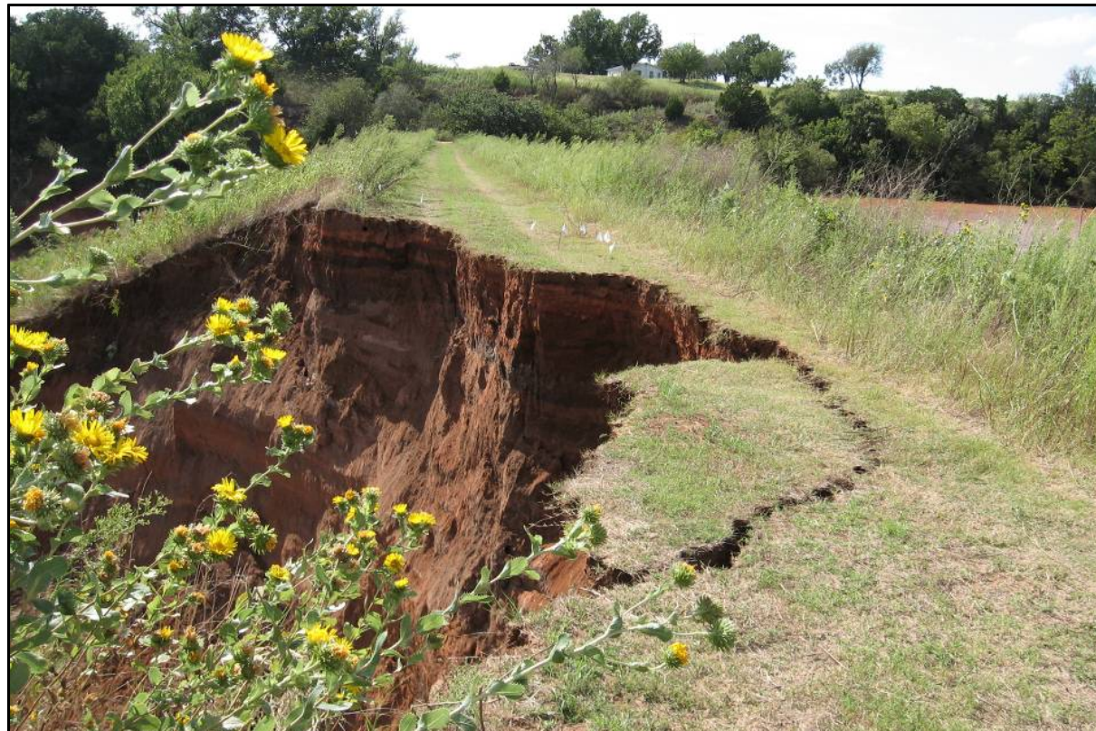
Figure 13. Photographs showing the flow path and erosion in the downstream slope of Sugar Creek Dam L-44 located in Caddo County, Oklahoma following Tropical Depression Erin on August 19, 2007.
