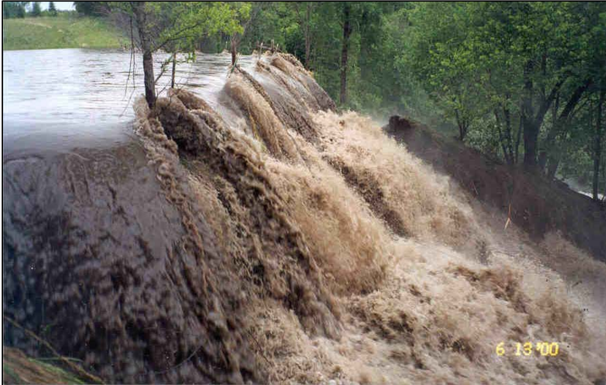
Figure 10. Headcut initiation at the outlet of the constructed portion of the auxiliary spillway
