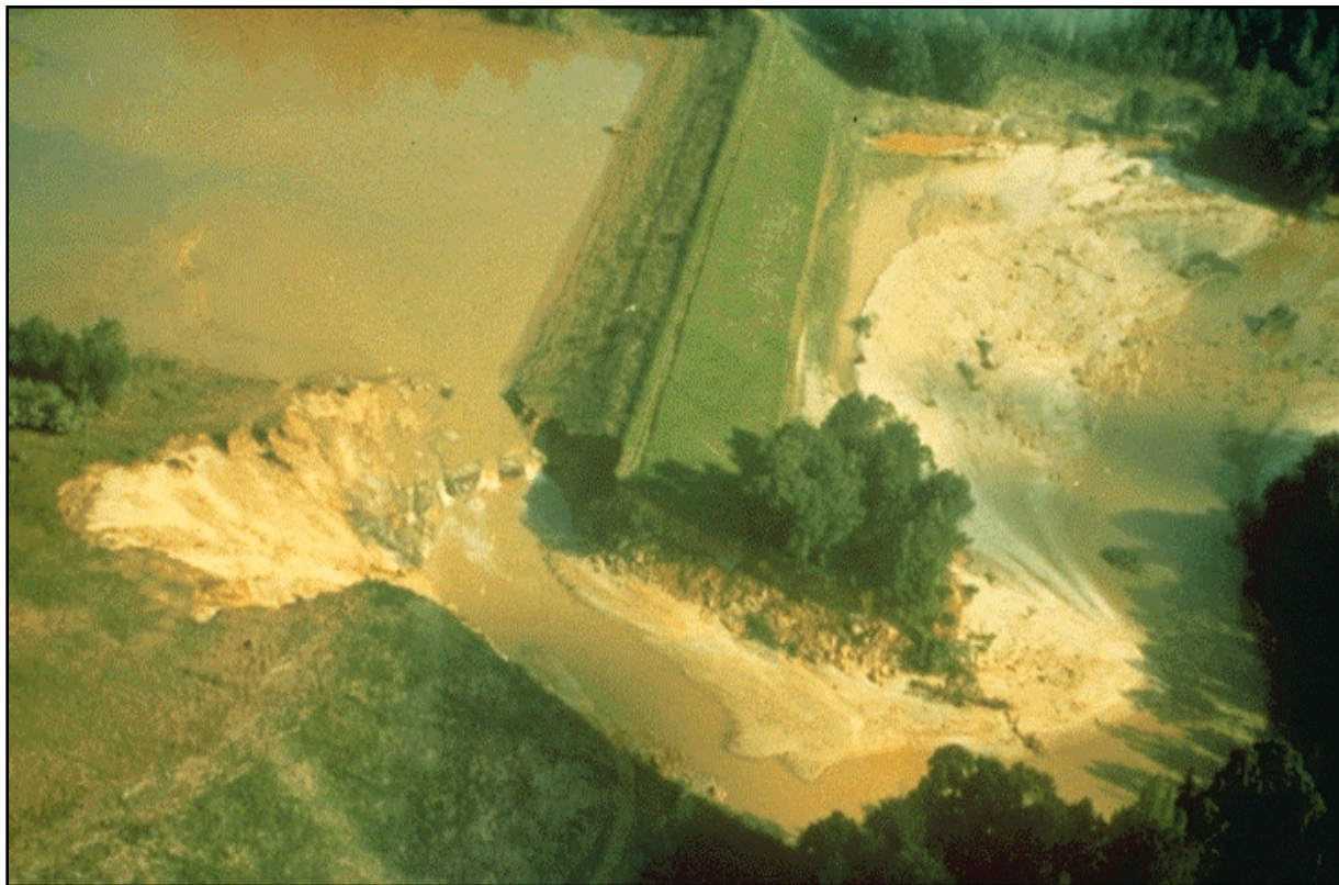
Figure 1. Failure of Black Creek Site 53 Auxiliary Spillway (Photo courtesy of Darrell Temple)
