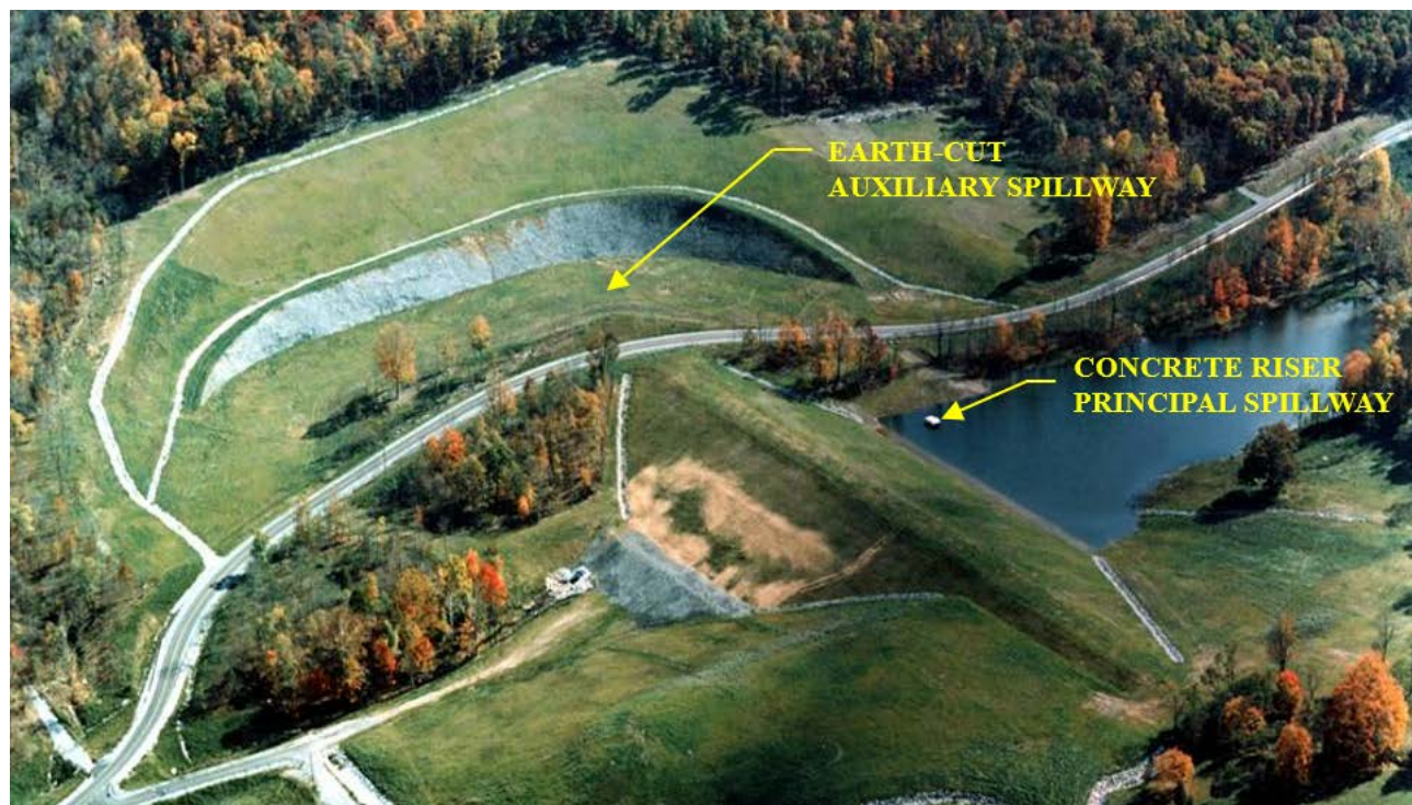
Figure 2. Typical NRCS Flood Control Dam with Auxiliary Spillway (Lost River Site 27, Hardy County, West Virginia)
