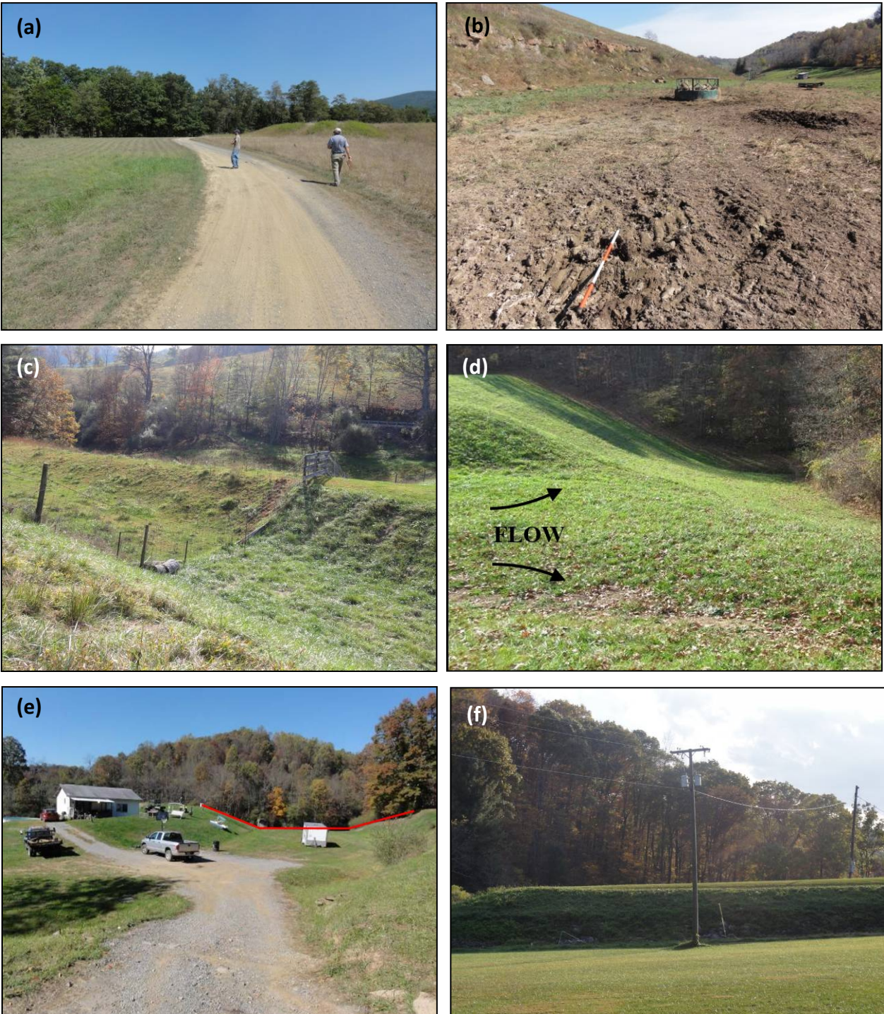
Figure 12. Photos Showing Typical Examples of Observed Deviations From Recommended Auxiliary Spillway Practice; (a) Dirt Road Parallel to Flow, (b) Sparse Grass Cover Due to Livestock, (c) Fence Across Spillway, (d) Spillway Exit Channel Along Toe of Dam, (e) Road Across Spillway and Obstructions In Spillway, (f) Utility Pole In Spillway.
