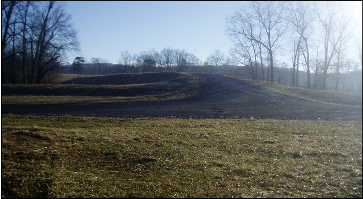
Figure 11. Ramp to Top of Dam across Auxiliary Spillway Control Section
