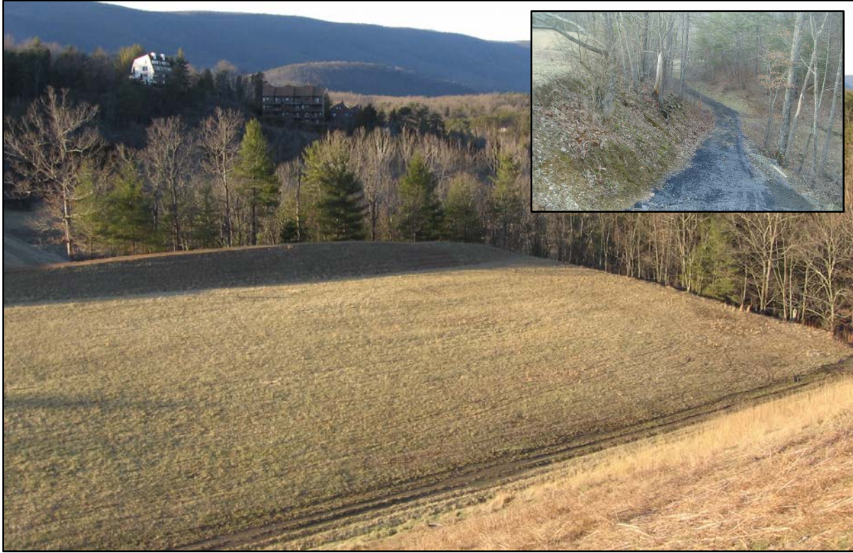
Figure 9. Well maintained auxiliary spillway with steep drop (road cut) beyond constructed section
