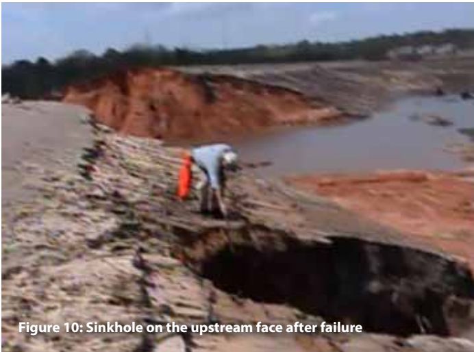
Figure 12: Dam breach
