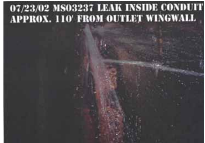
Figure 4: Leakage into the conduit
