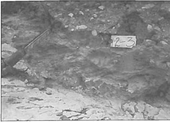
FIGURE 10. A clay layer 5 to 20 cm thick along the failure surface at location 12-3, near the east side of the slide.
