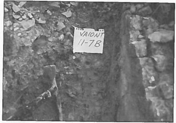
FIGURE 16. A clay layer, at location 11-7B, 10 cm thick lying between bedrock to the right and slide debris to the left. The clay is protected by a cascade structure, but is associated with the nearby failure surface.
