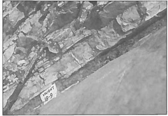
FIGURE 12. Clay interbed 5 cm thick along the failure surface at location 18-9. Other thin clay interbeds up to 0.5 cm thick lie in the rock mass.
