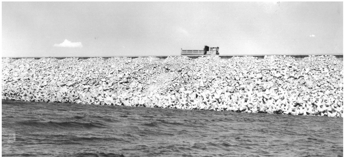
Figure 11. Newly Installed Kingsley Dam Erosion Protection Following 1972 Windstorm Repairs [10].
