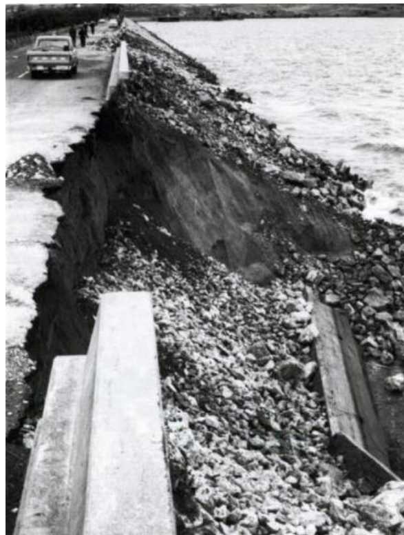
Figure 5. 1972 Windstorm Damage to Kingsley Dam [5]. Note the collapse of the concrete parapet wall.
