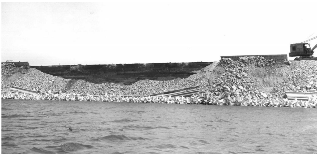
Figure 7. 1972 Windstorm Damage to Kingsley Dam [10]. Note collapsed parapet wall and emergency placement of hexapods at waterline.
