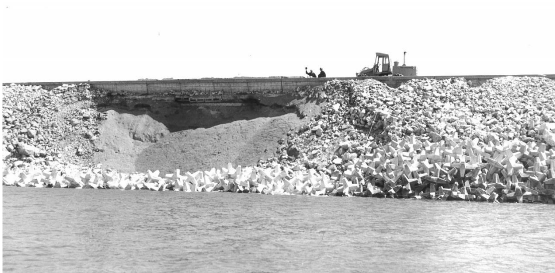
Figure 6. 1972 Windstorm Damage to Kingsley Dam [10]. Note the emergency placement of hexapods at the waterline.
