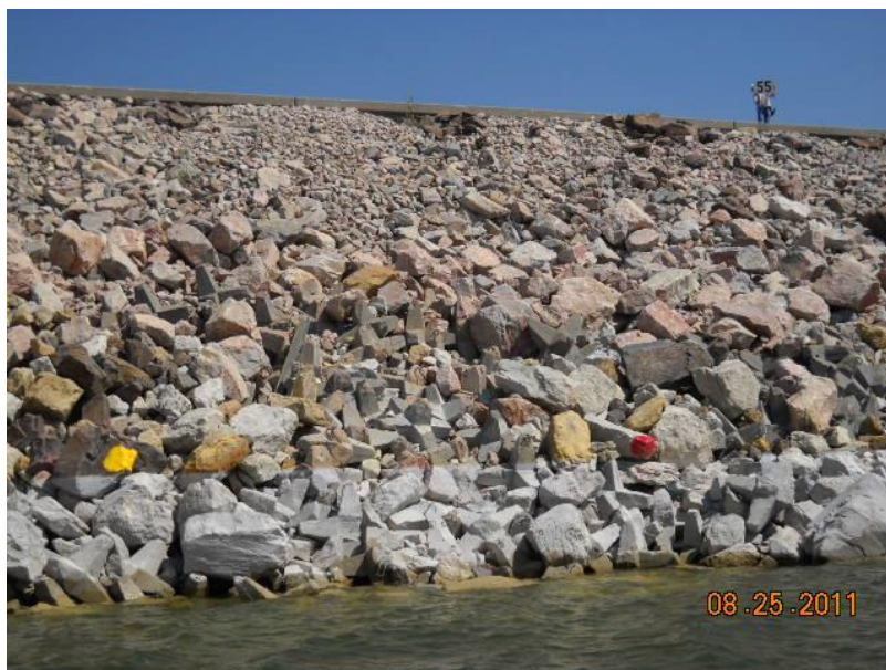
Figure 12. Paint Marks on Kingsley Dam Riprap for Monitoring Movement [12].
