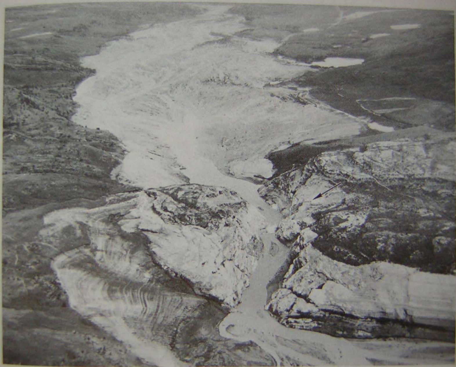
FIGURE 27.—Remains of Swift Dam looking downstream from the reservoir area. Arrow points to a part of the right end of the upstream face of the dam.
