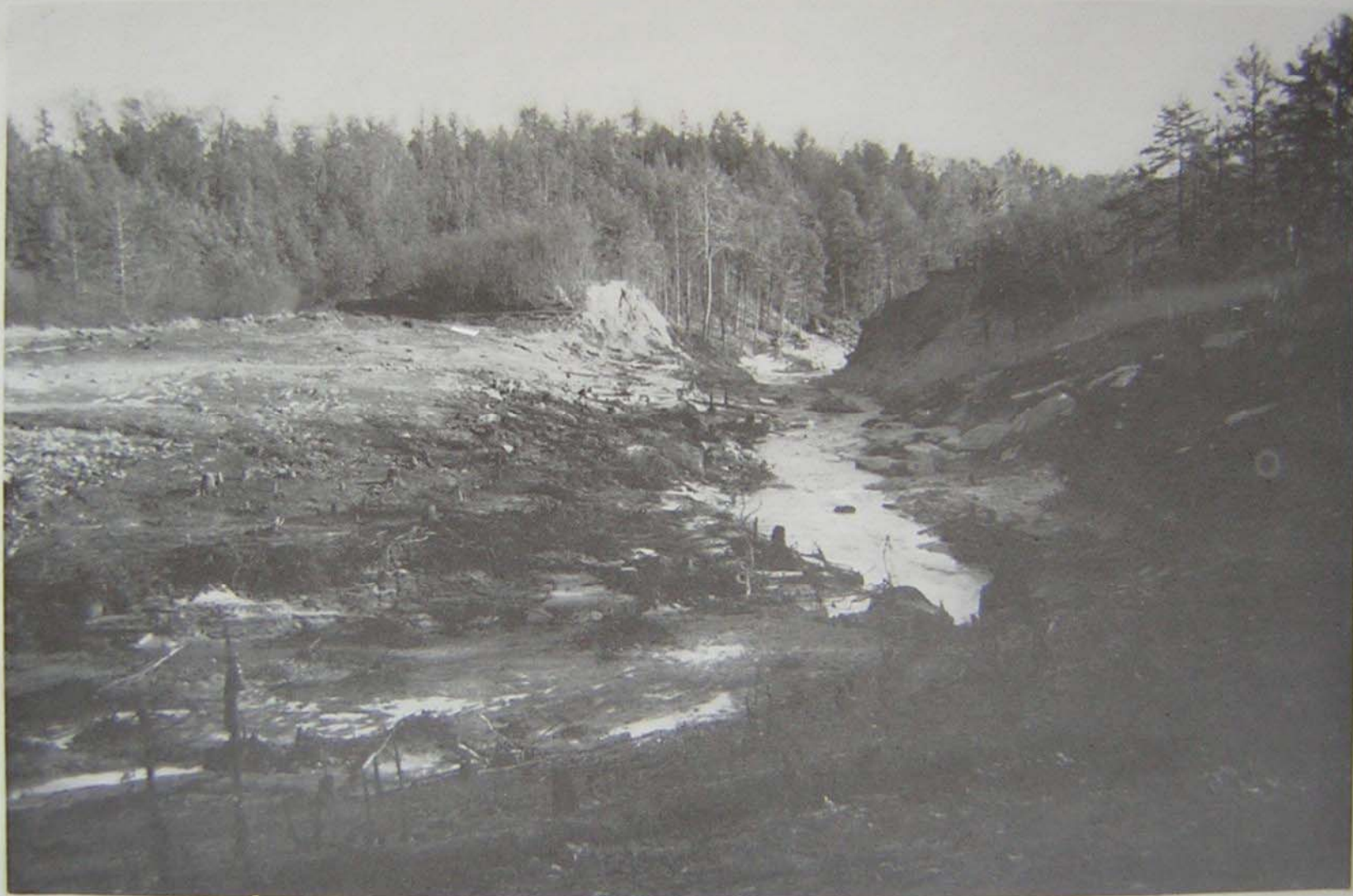
FIGURE 2. — Lakebed and remains of Kelly Barnes Dam. (View downstream)
