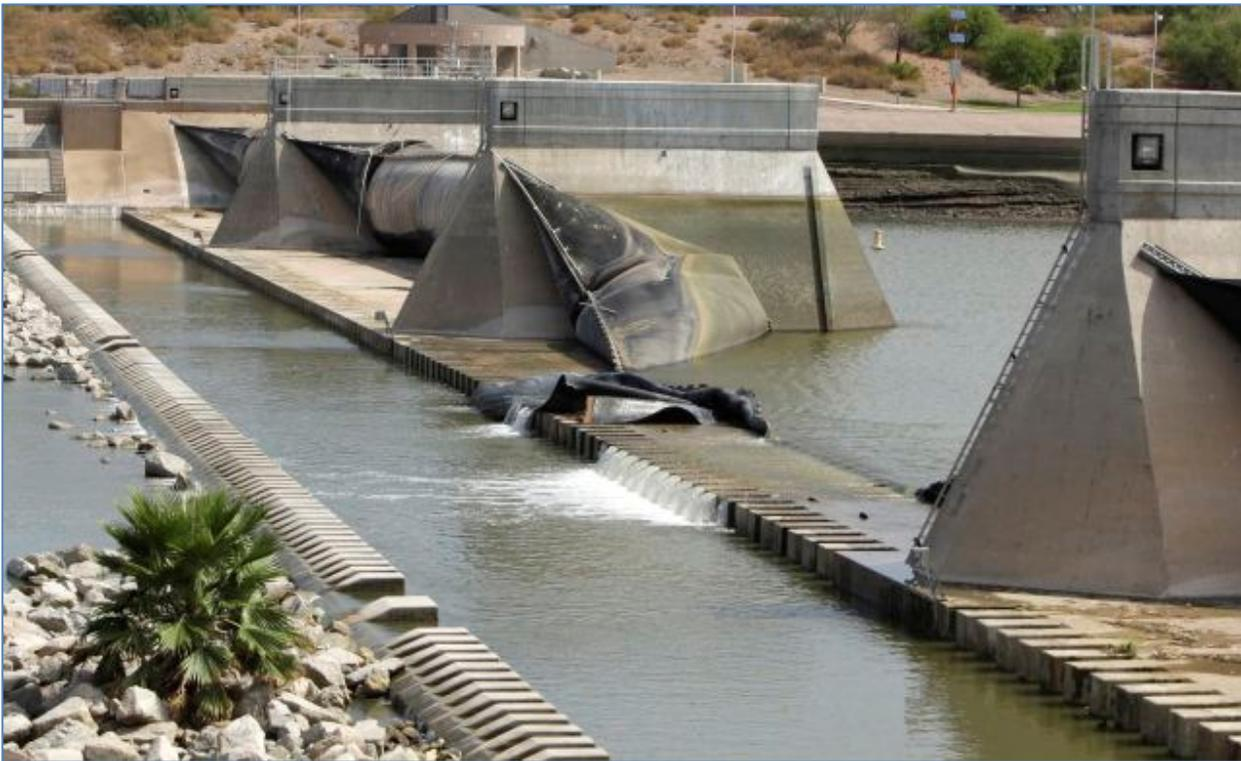
Figure 1. Photo of Failed 16-foot-High Rubber Dam at Tempe Town Lake, July 21, 2010.
