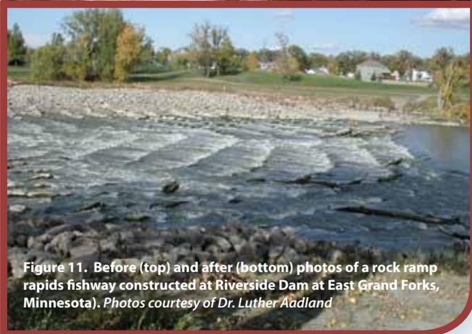
**Figure 11. Before (top) and after (bottom) photos of a rock ramp rapids fishway constructed at Riverside Dam at East Grand Forks, Minnesota).** Photos courtesy of Dr. Luther Aadland
