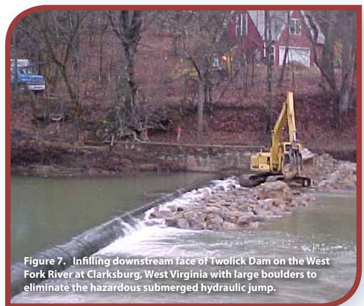
Figure 7. Infilling downstream face of Twolick Dam on the West Fork River at Clarksburg, West Virginia with large boulders to eliminate the hazardous submerged hydraulic jump.
