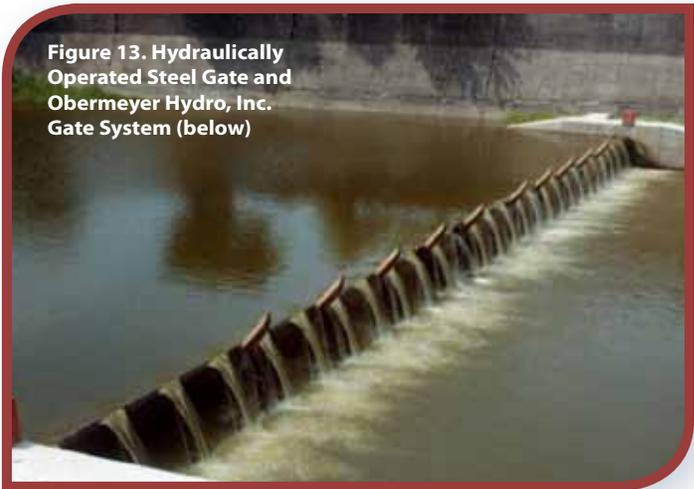
**Figure 13. Hydraulically Operated Steel Gate and Obermeyer Hydro, Inc. Gate System (below)**
