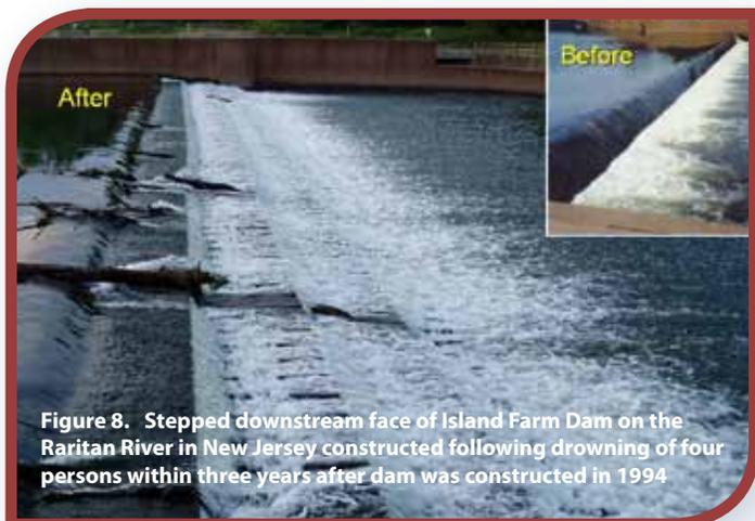
**Figure 8. Stepped downstream face of Island Farm Dam on the Raritan River in New Jersey constructed following drowning of four persons within three years after dam was constructed in 1994**
