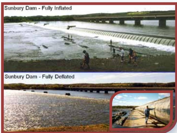
**Figure 9. Bridgestone Inflatable Dam on Susquehanna River at Sunbury, Pennsylvania, with no drowning incidents since it was constructed in 1969, despite intense recreation activity.**
