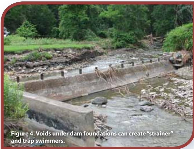
Figure 4. Voids under dam foundations can create “strainer” and trap swimmers.
