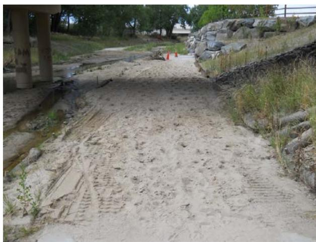
**Photograph 10-2.** Sediment frequently accumulates under crossings. Frequently inundated paths collect sediment and are maintenance-intensive.
