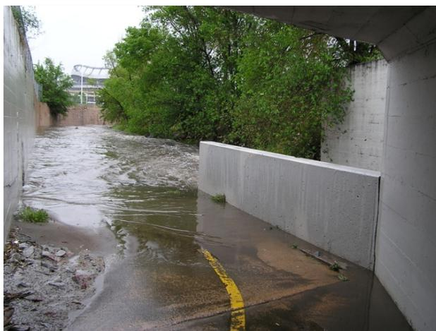
**Photograph 10-1.** Frequently inundated channels pose a high threat to public safety, especially in a walled channel where water can rise rapidly and egress is limited.
