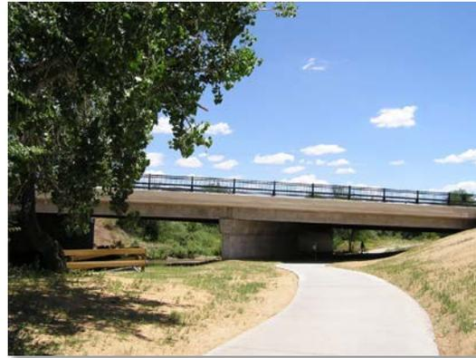
**Photograph 10-14.** This bridge offers safe passage, providing the user with a view of potentially rising water and the path beyond the structure. Additionally, the slope from the path to the roadway offers the user a passable route to higher ground in case of flash flooding.
