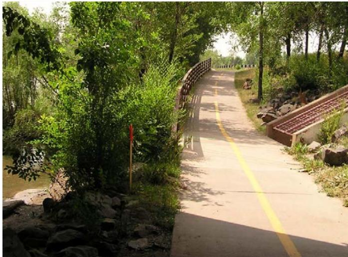
**Photograph 10-10.** Along this section of the South Platte River, the combination of a steep longitudinal slope, a cross drainage structure, and a steep slope from the path to the water warranted both a safety rail and striping.
