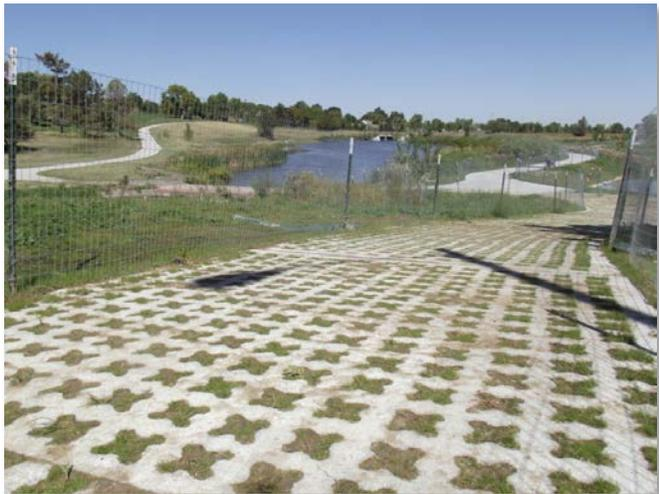
**Photograph 10-26.** Reinforced grass pavement shortly after construction.
