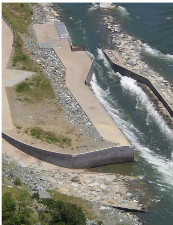
**Photograph 10-33.** The intake works on the American River near Auburn, California relies on a submerged self-cleaning fine screen. The screen is located in the invert of a boatable channel. This design eliminates intake apparatus that can be hazardous to recreationists, screens for fish and solids, and has proven to require relatively little maintenance. Photo courtesy of Placer County Water Agency.
