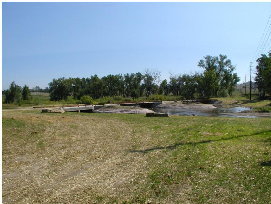
**Photograph 10-20.** This Cherry Creek crossing was split into three segments to accommodate the long span. Curb rails were used and the path was kept low to minimize impediment to flood flows. Photo Courtesy Muller Engineering.
