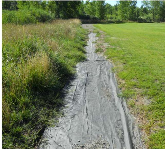
**Photograph 10-27.** Geotextile is all that is left of this crusher fines trail that washed out on Goldsmith Gulch.
