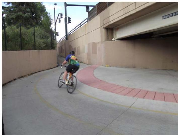
**Photograph 10-13.** Understanding the popularity of the Cherry Creek path, designers worked to make the underpass at University safe for bicyclists and pedestrians while working within the limitations of the existing site. Land was purchased to create a suitable turning radius at this 90 degree bend. This provides bicyclists with additional time to react to the unexpected.
