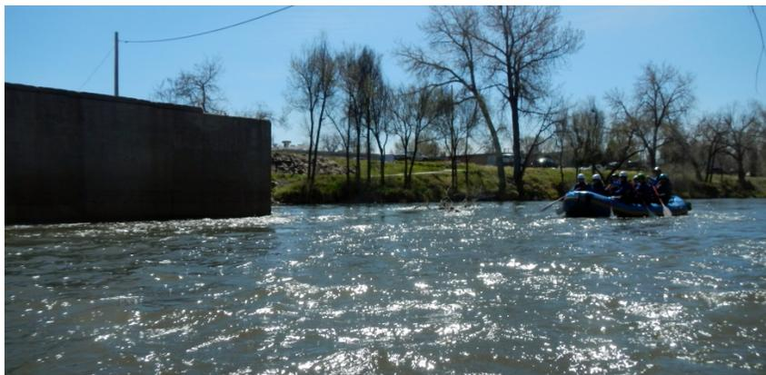
**Photograph 10-39.** The “pier nose extensions” on this bridge reduce the accumulation of debris and thereby improve safety for in-river users. Photo courtesy of McLaughlin Whitewater Design Group.
