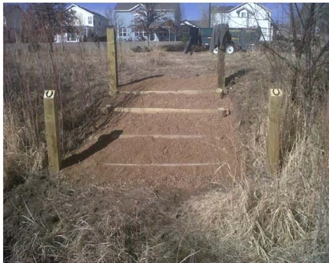
**Photograph 10-24.** Timber steps filled with roadbase are constructed to provide traction approaching a water crossing. Photo courtesy Arapahoe Park and Recreation District.
