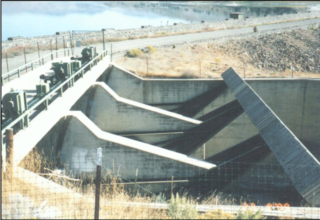
*Photograph No. 1.—Radial gates as installed on the right embankment.*
