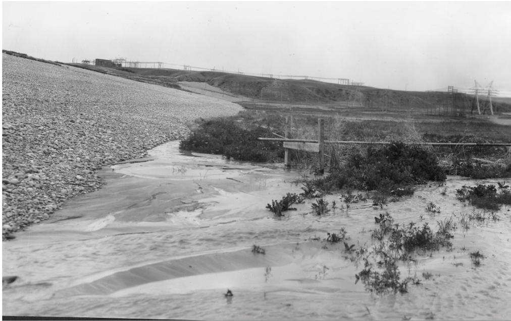
Figure 9. Sand boils at toe with reservoir partially filled.
