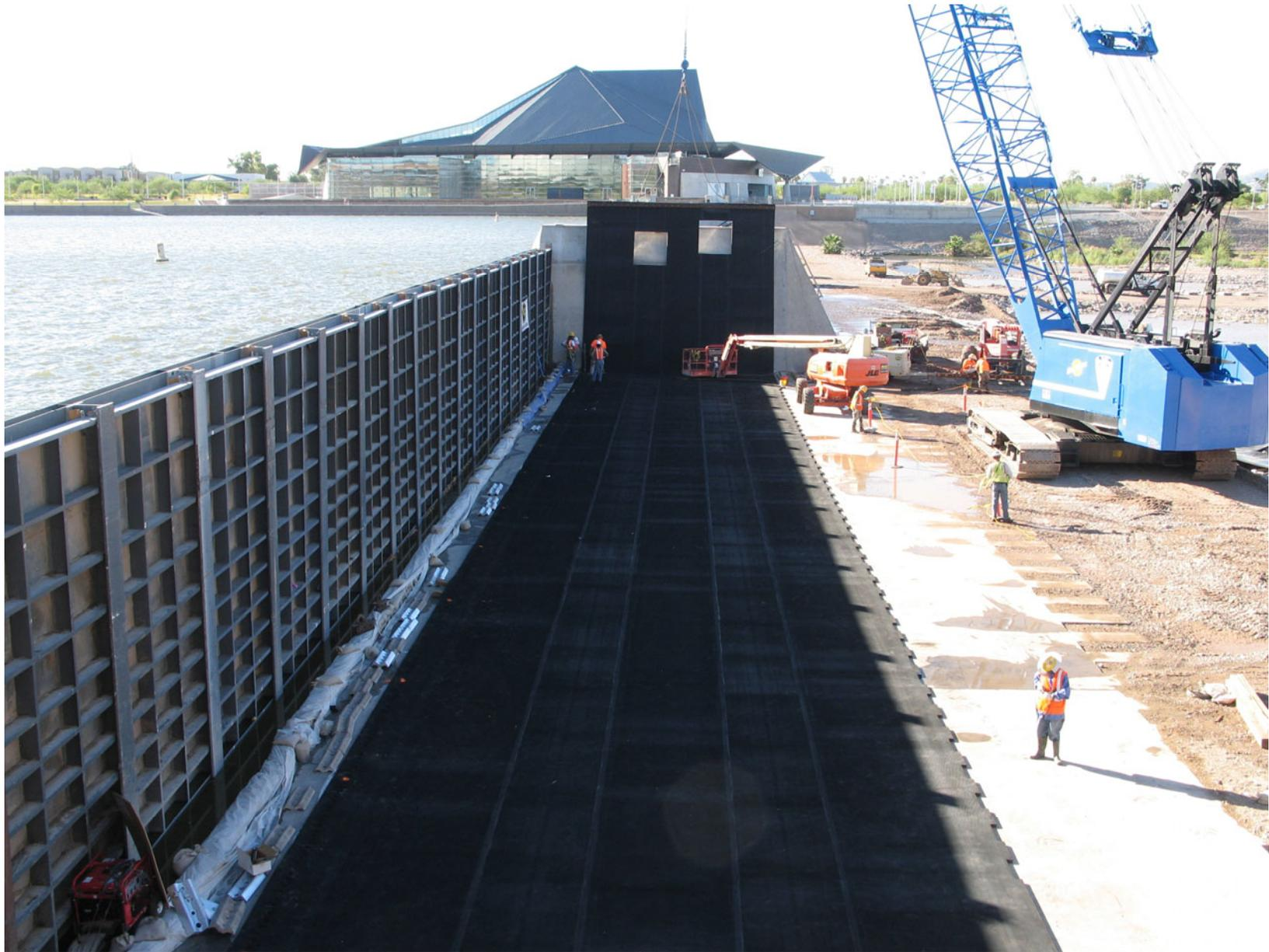
**Figure 3.** Installation of the fourth rubber bladder at Tempe Town Lake Dam with the steel coffer dam in place and the lake filled.
