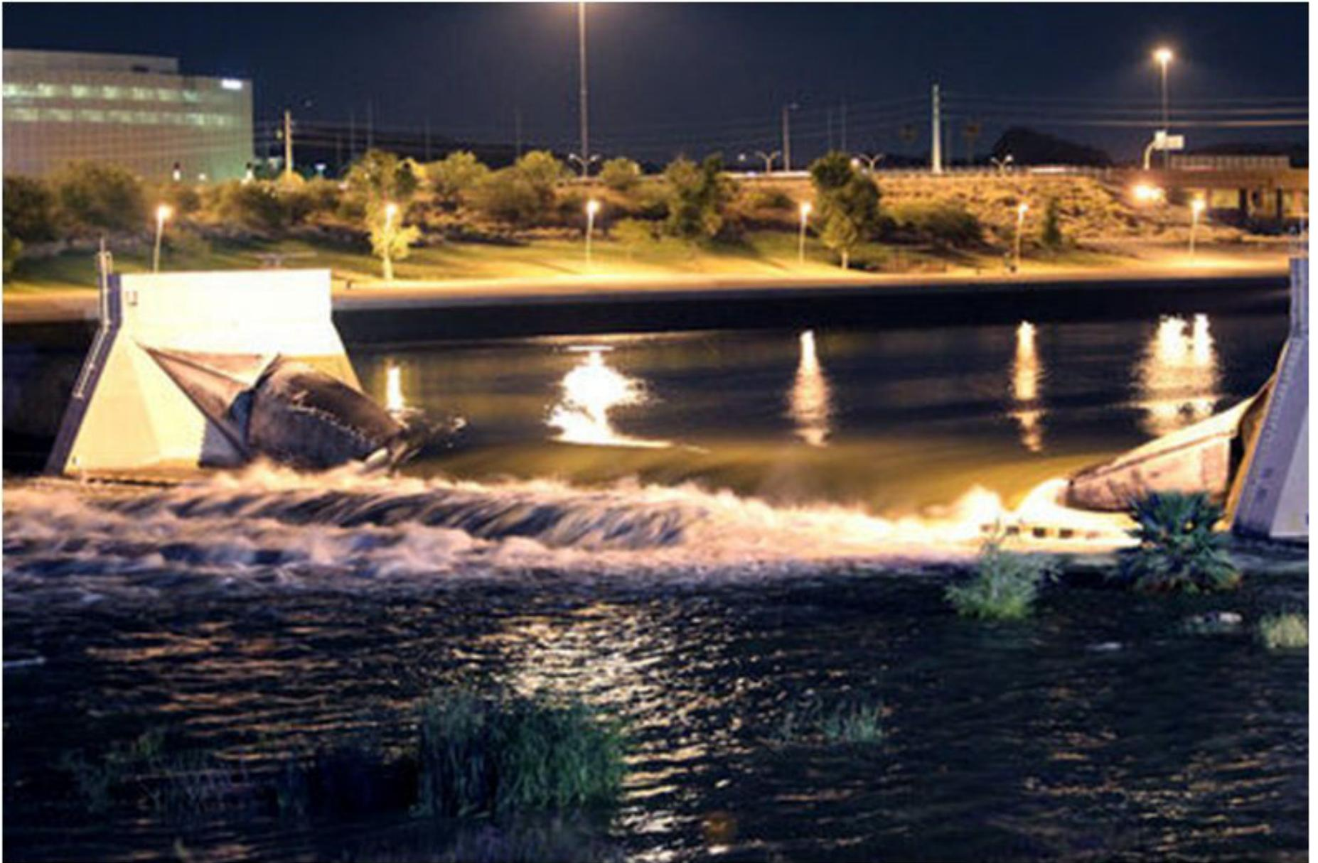
**Figure 2.** Rubber bladder failure at Tempe Town Lake Dam on 20 July 2010.
