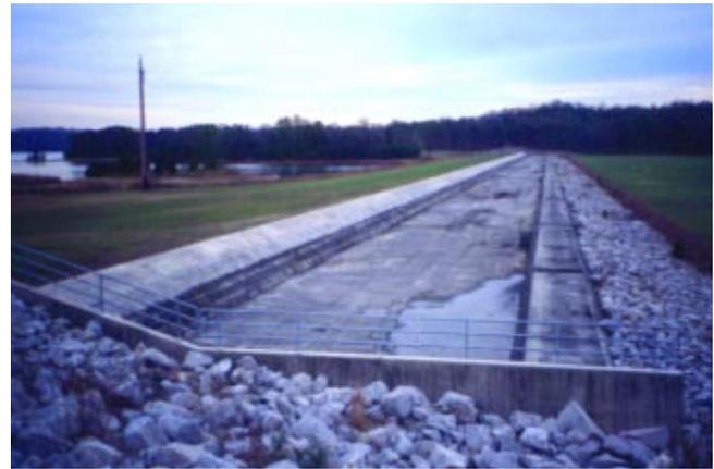
**Figure 6.21b. Completed ogee crest weir (Tellico Dam, Tennessee).**
