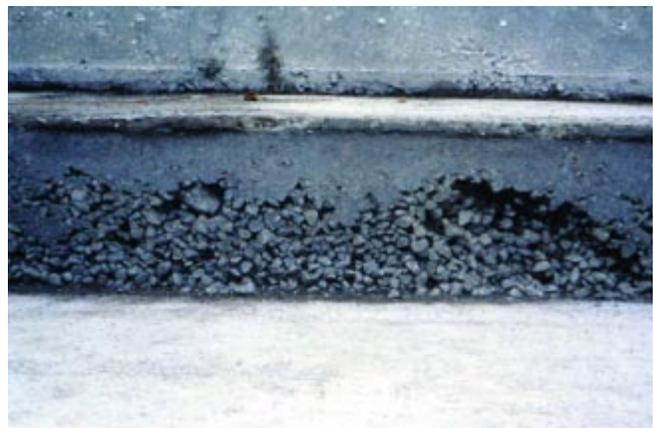
Figure 9.14. Example of “poor” appearance of RCC placed against a vertical form.
