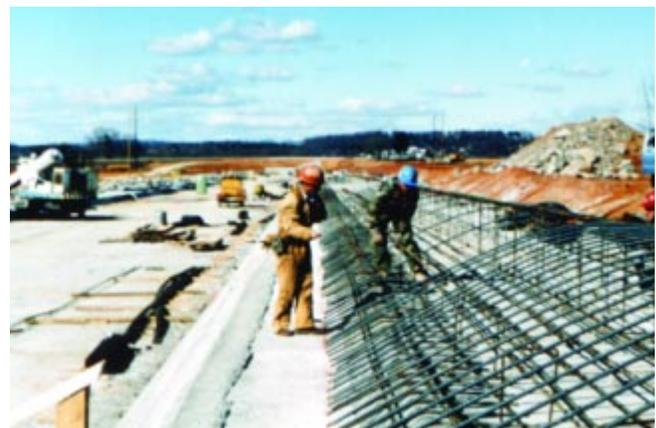
Figure 6.15. Installing reinforcement steel for modified ogee crest weir (Tellico Dam, Tennessee).
