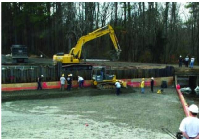
**Figure 6.27. Steel sheet pile for downstream cut-off wall (McKinney Lake, North Carolina).**
