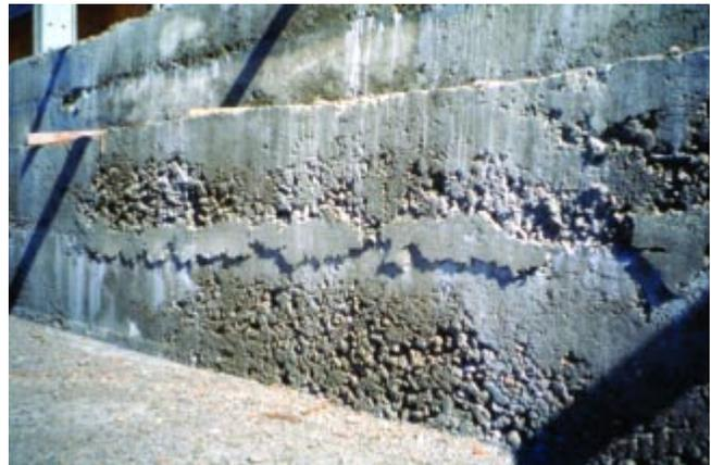
Figure 9.13. Example of “fair” appearance of RCC placed against a vertical form.
