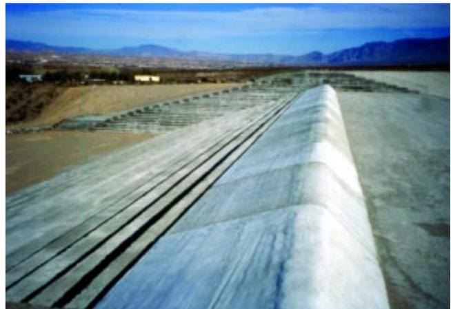
Figure 6.19. Sloping ogee crest weir constructed with conventional concrete (Windmill Wash, Nevada).
