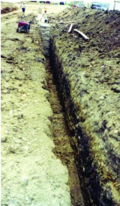
**Figure 6.26. Overtopping spillway — upstream cut-off wall during concrete placement.**
