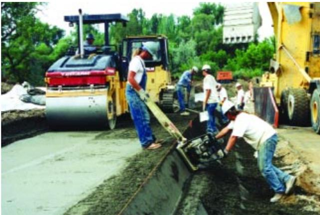
**Figure 9.9. Compacting downstream RCC slope (note string line for alignment control).**
