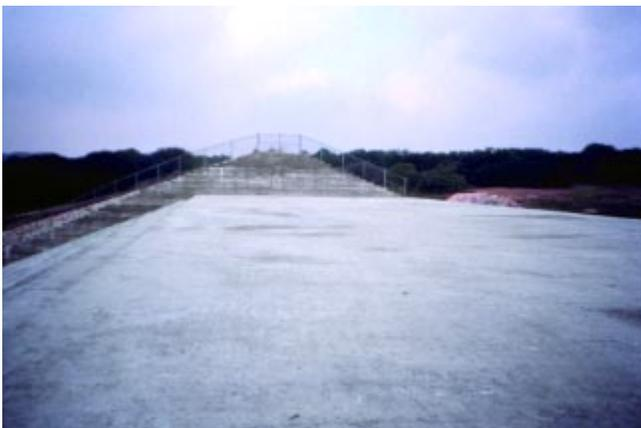
Figure 6.14. Broad crest weir construction of RCC (Saklado Dam No. 10, Texas).
