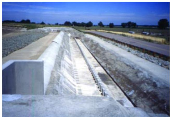
Figure 6.20a. Modified ogee crest weir (Coal Ridge, Colorado).
