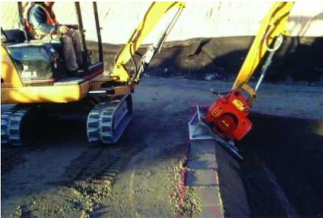
**Figure 9.10. Compacting downstream RCC face with track hoe mounted hydra-plate compactor.**
