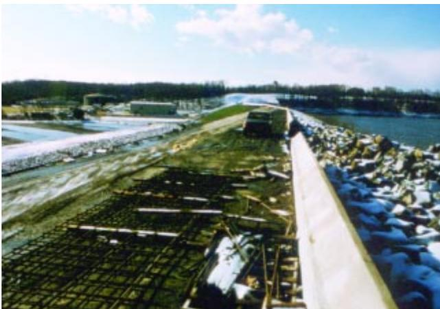
Figure 6.17. Sharp crest weir wall under construction (Smith Lake Dam, Virginia).
