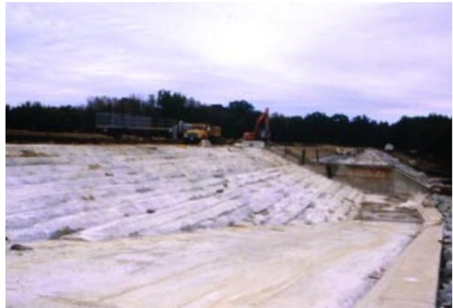
**Figure 6.7. Unformed RCC chute with compacted RCC (Fawell Dam, Illinois).**
