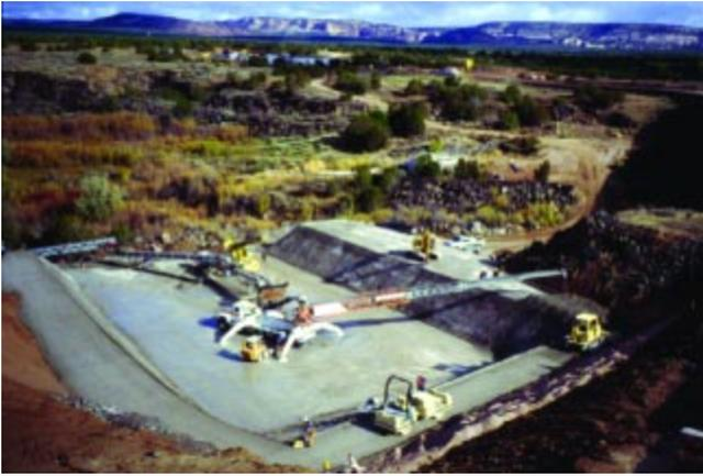
**Figure 9.6.** RCC delivery using conveyors and mobile super swinger (Black Rock Dam, New Mexico).
