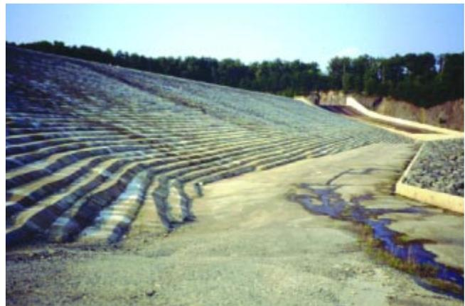
**Figure 6.8. Unformed RCC chute with compacted RCC (Smith Lake Dam, Virginia).**
