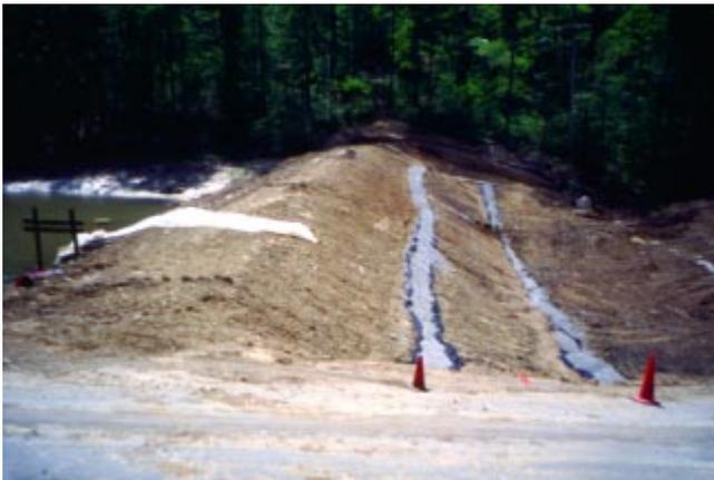
Figure 6.32. Trench drain construction prior to RCC placement (McBride Dam, Ohio).
