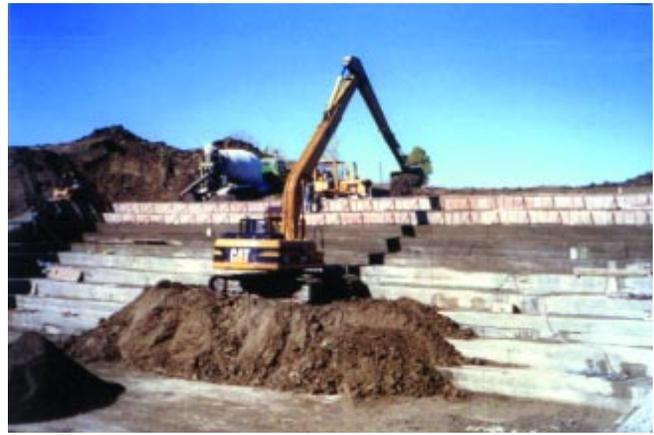
**Figure 9.4. RCC delivery with a long stick track hoe (Hayes Dam, South Dakota).**
