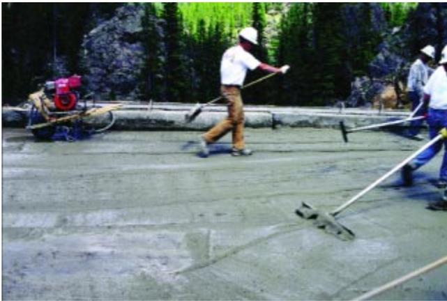
Figure 9.20. Bedding mortar placement.
