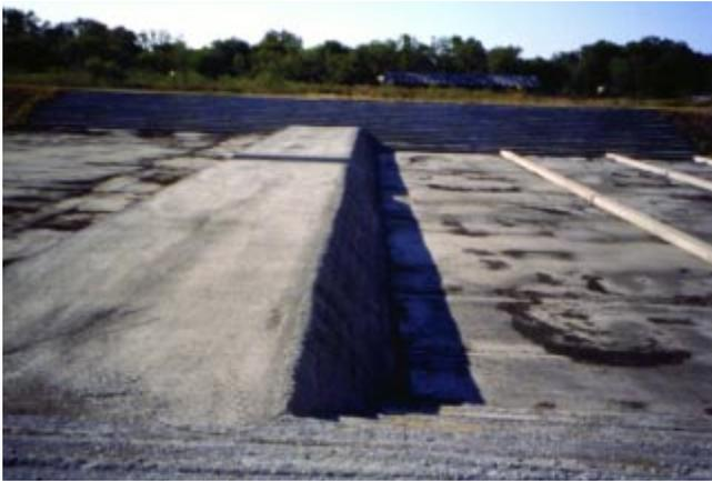
**Figure 2.2. In-stream drop structure (Cooks Slough, Texas).**
