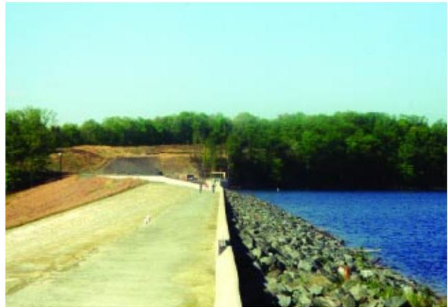
Figure 6.18. Sharp crest weir and with completed RCC overtopping section (Smith Lake Dam, Virginia).
