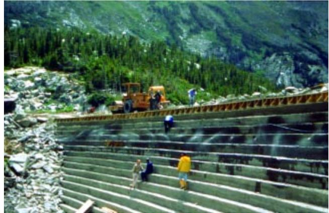
Figure 6.10. Formed RCC chute (Goose Lake, Colorado).
