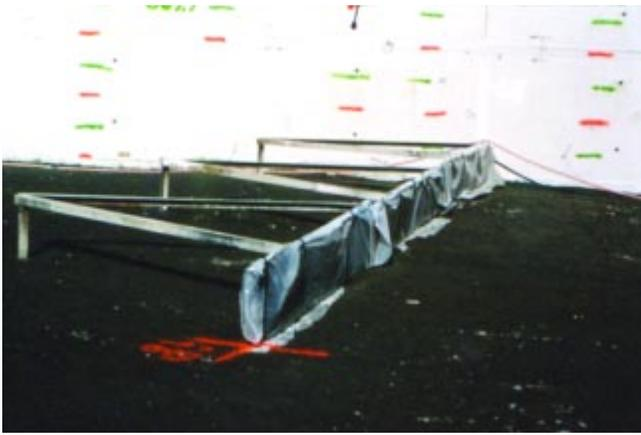
**Figure 9.17. Control joint form using plastic sheeting.**
