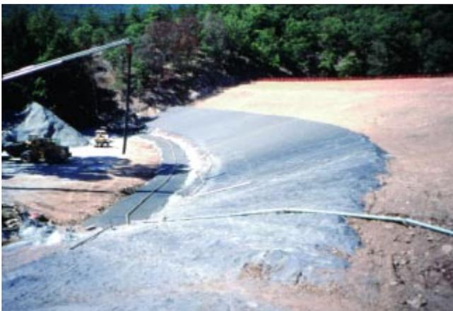
Figure 6.33. Blanket drain construction prior to RCC placement (Douthat Dam, Virginia).
