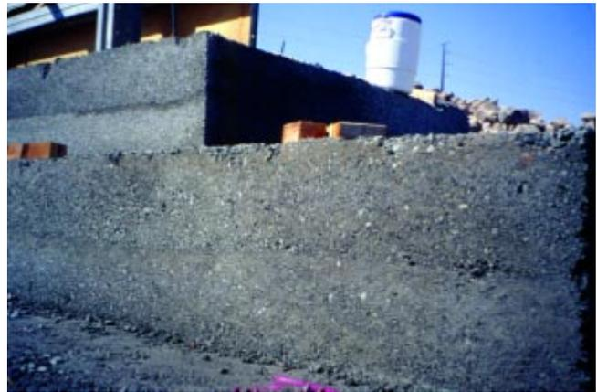
Figure 9.12. Example of “good” appearance of RCC placed against a vertical form.
