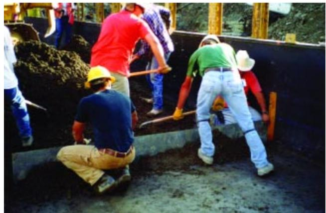
Figure 9.16. Control joint plate placed during RCC placing.
