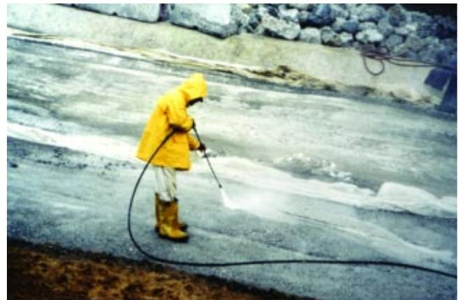
**Figure 9.18. Cold joint preparation.**
