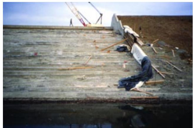
Figure 6.42. Conventional concrete training wall being constructed on completed RCC (Leyden Dam, Colorado).
