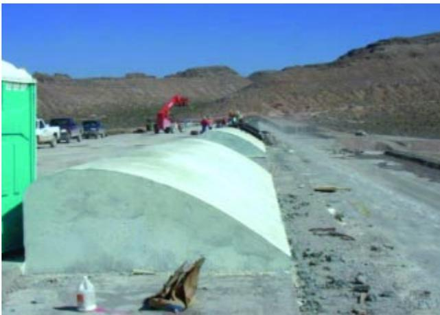
**Figure 6.21a. Modified ogee crest weir constructed of unreinforced concrete placed in segments (Blue Diamond, Nevada).**
