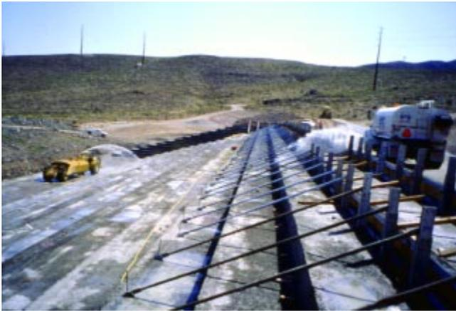
**Figure 6.12. Formed RCC chute, 2 foot high steps (Anthem No. 2, Nevada).**
