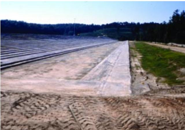
Figure 6.24. Stilling basin constructed of RCC (Lake Tholocco Dam, Alabama).
