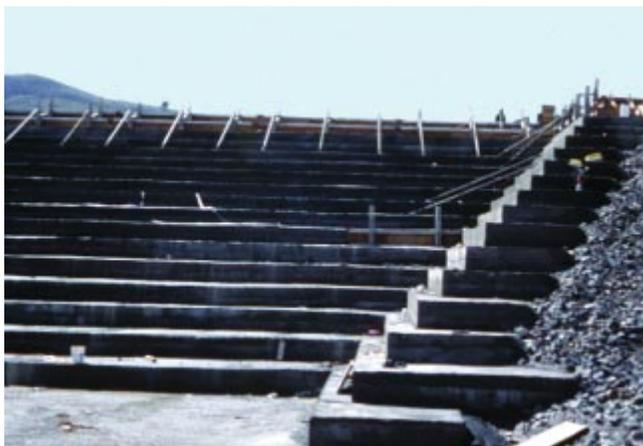
Figure 6.37. RCC training walls constructed using formed sloping RCC wall (Anthem No. 2, Nevada).
