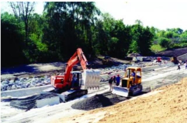
**Figure 9.3. RCC delivery with a track hoe (Fawell Dam, Illinois).**
