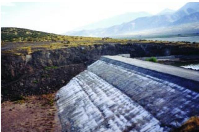
**Figure 6.6. Uncompacted, unformed RCC downstream face (Mona Dam, Utah).**
