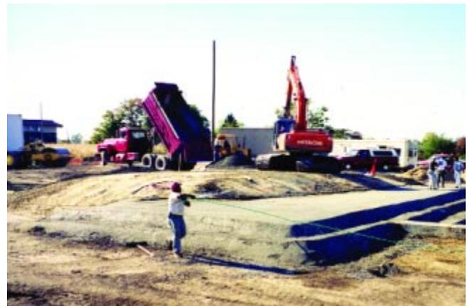
Figure 9.21. RCC transition area construction.
