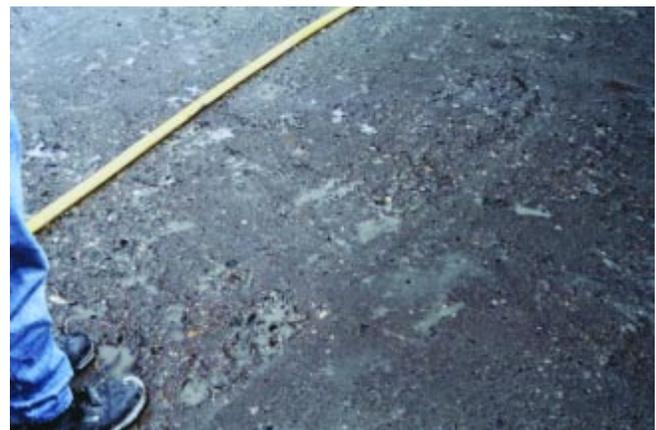
**Figure 9.19. Example of well prepared RCC cold joint surface.**
