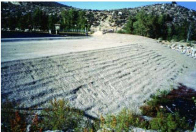
**Figure 6.5. Uncompacted, unformed RCC downstream face (Bishop Creek Dam No. 2, California).**
