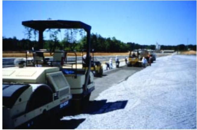
**Figure 9.7.** RCC spreading and compaction (Lake Tholocco Dam, Alabama).
