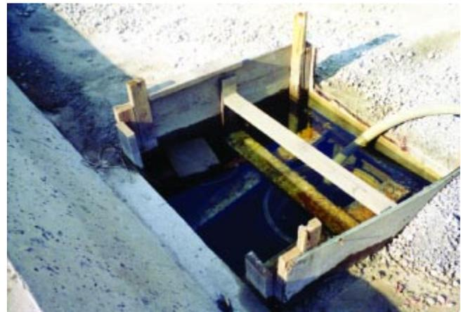
**Figure 9.1. Dewatering sump adjacent to downstream cut-off wall in stilling basin runout apron.**
