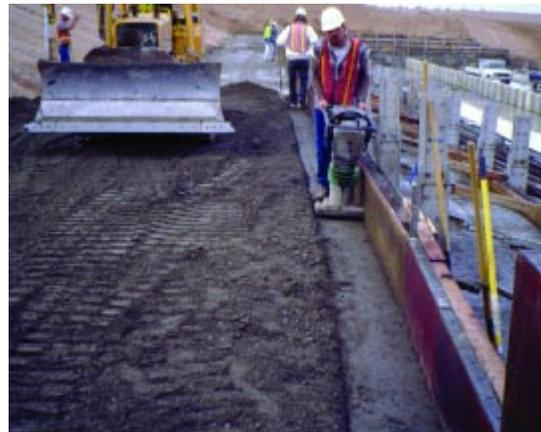
**Figure 9.8.** Hand compaction of RCC adjacent to step form.
