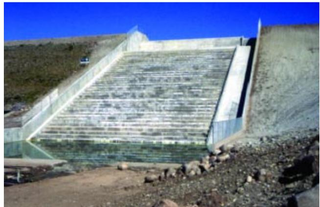
Figure 6.11. Formed RCC chute (Big Beaver Dam, Colorado).
