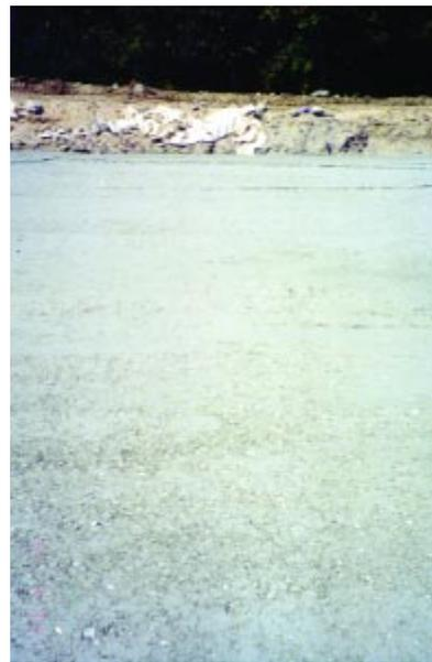
Figure 9.11. Appearance of a “good” RCC finish surface.
