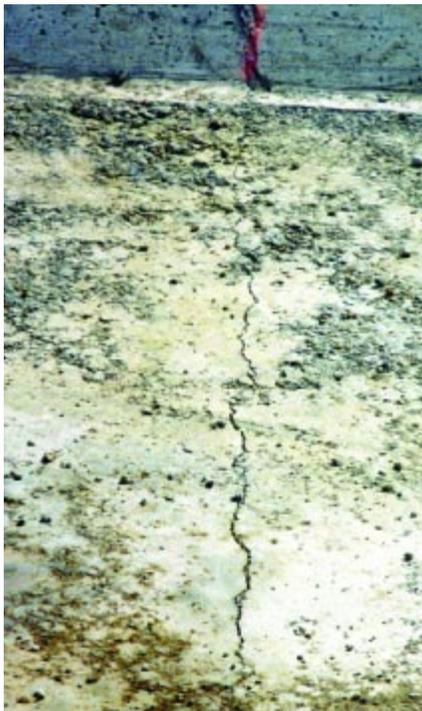
Figure 6.29. Naturally occurring shrinkage crack in RCC.
