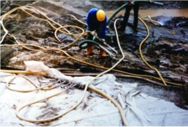
**Figure 9.2.** Foundation preparation and cleaning using a vacuum device.
