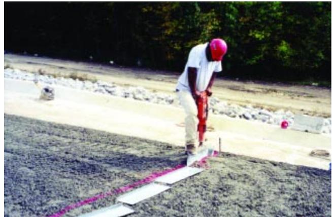
Figure 9.15. Installation of control joint plate.
