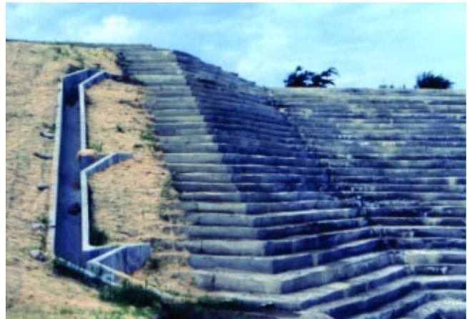
Figure 6.35. Concrete drain outlet structure (South Prong Dam, Texas).
