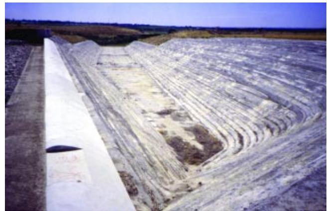
**Figure 2.3. RCC side channel spillway (Cold Springs Spillway, Oregon).**
