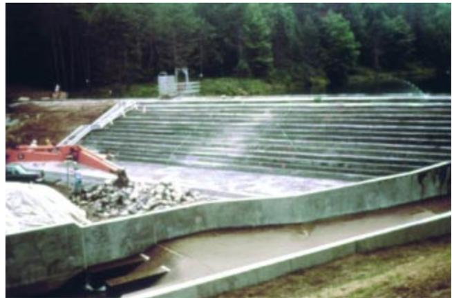
Figure 6.43a. RCC spillway before soil cover is placed (Philipsburg Dam 3, Pennsylvania).
