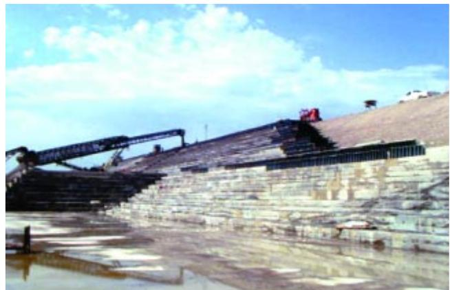
**Figure 9.5. RCC delivery using conveyor system (Blue Diamond Dam, Nevada).**
