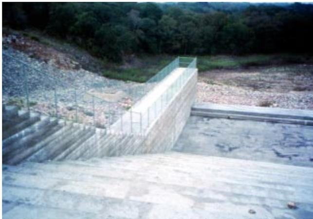
Figure 6.36. RCC training wall constructed using vertical forms (Salado No. 10, Texas).
