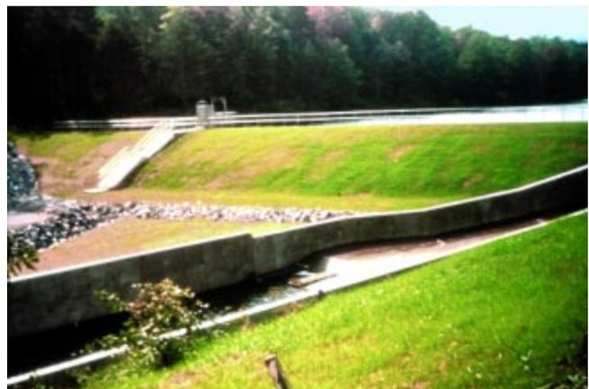
Figure 6.43b. RCC spillway after soil cover is placed (Philipsburg Dam 3, Pennsylvania).
