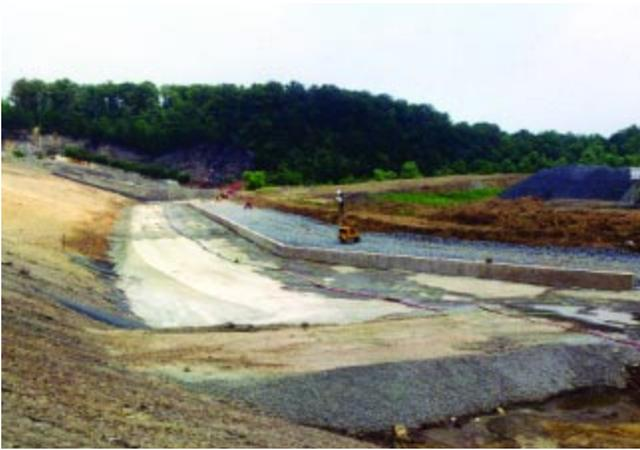
Figure 6.23. Run-out apron, end sill and riprap transition section under construction (Smith Lake Dam, Virginia).
