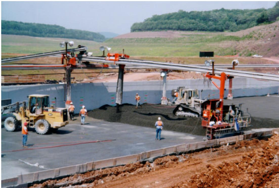
Figure 6-2. Conveyor system with mobile side discharge belt
