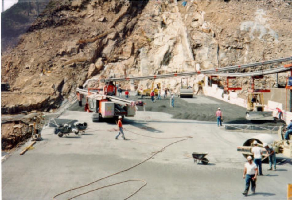
Figure 6-1. Conveyor system with self-propelled crawler-placer
