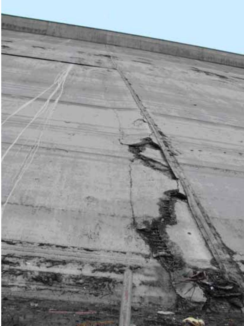
Figure 9. Face slab joint 23/24 near maximum section (from Chen).
