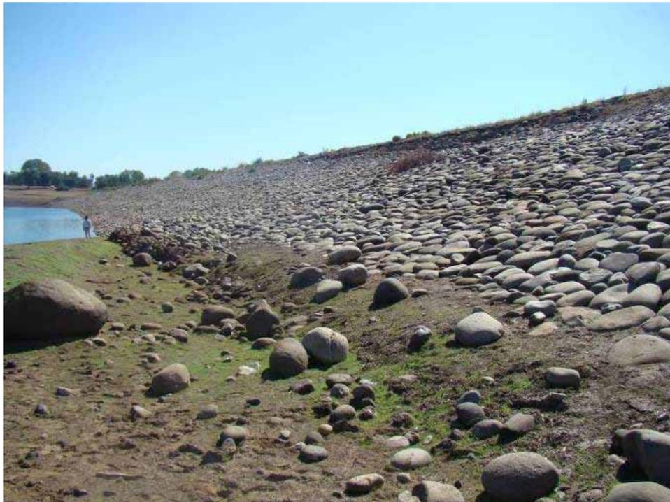
Figure 8. Slough B located right of the highest part of the embankment (from Bray et al., 2010).
