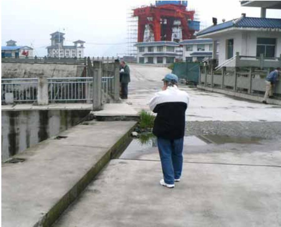
Figure 7. Embankment settlement at spillway wall (Babbitt).
