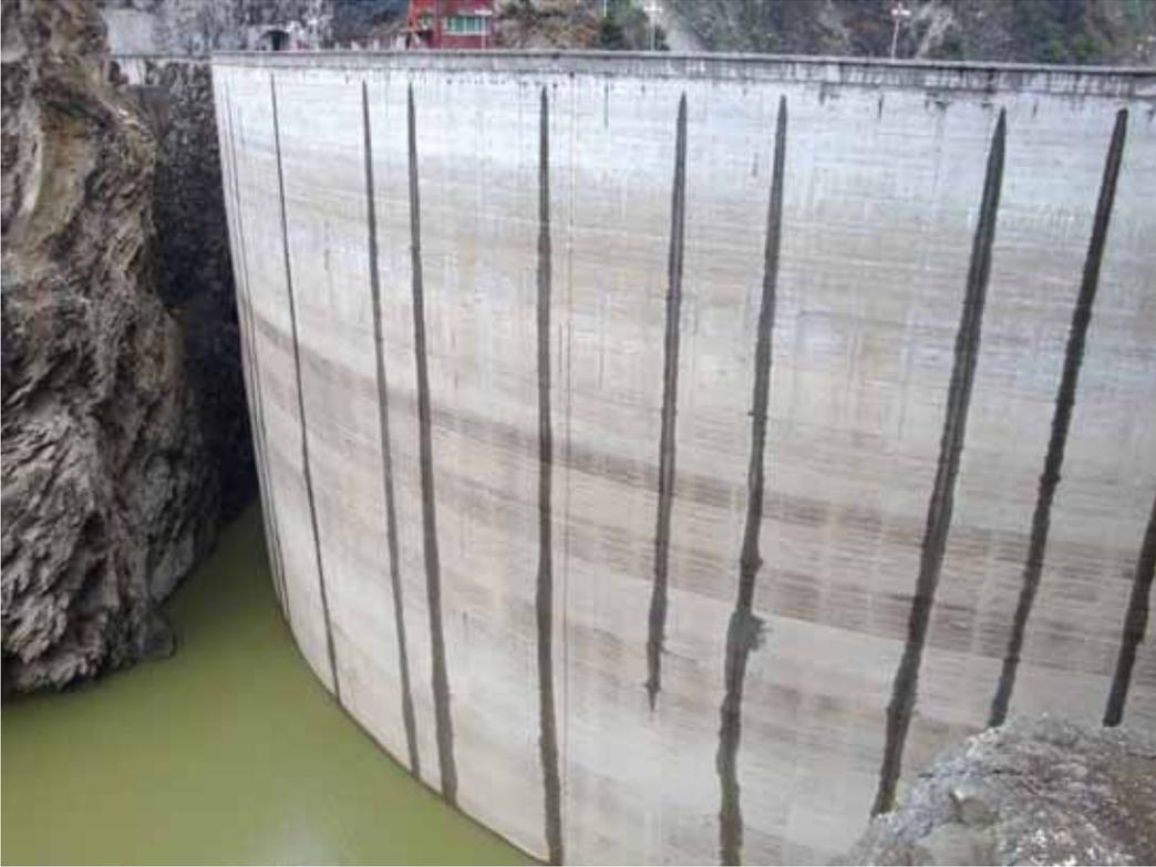
Figure 1. Shapai Dam from upstream after the earthquake (Babbitt).
