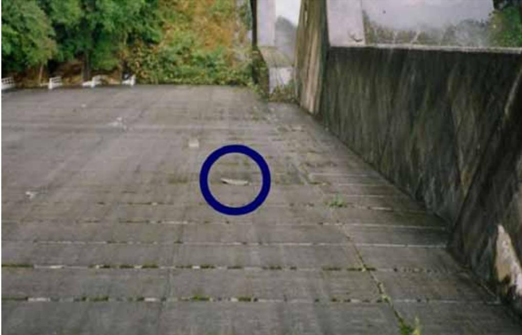
Figure 11. Concrete spill on the downstream face of Sugesawa Dam (from Yamaguchi et al., 2002).
