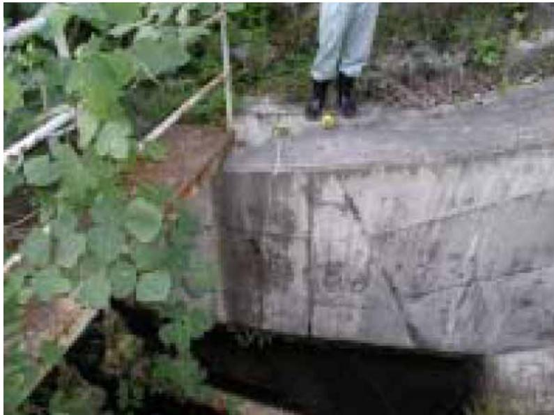
Figure 14. Cracking of the spillway channel wall of Uh Dam (from Takasu et al., 2000).
