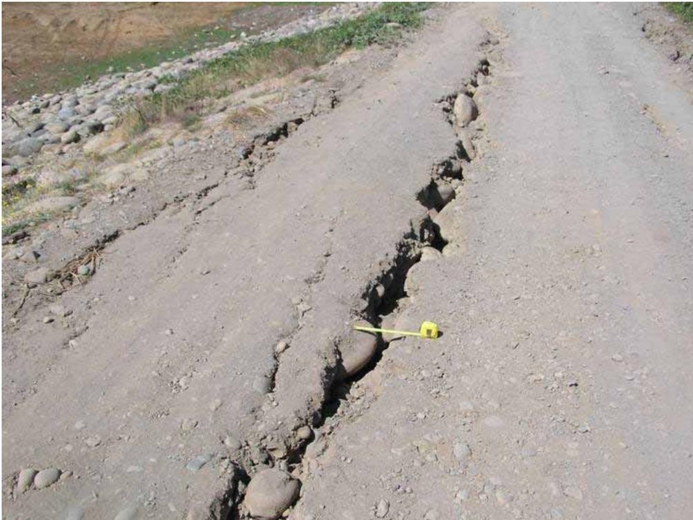
Figure 14. Cracking in crest of Saddle Dam (from Bray et al., 2010).
