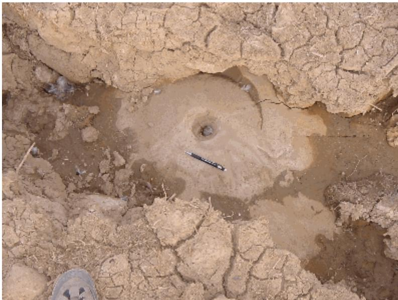
Figure 4. Sand boil observed in the reservoir near the upstream toe of Chang Dam (from GEER, 2001)
