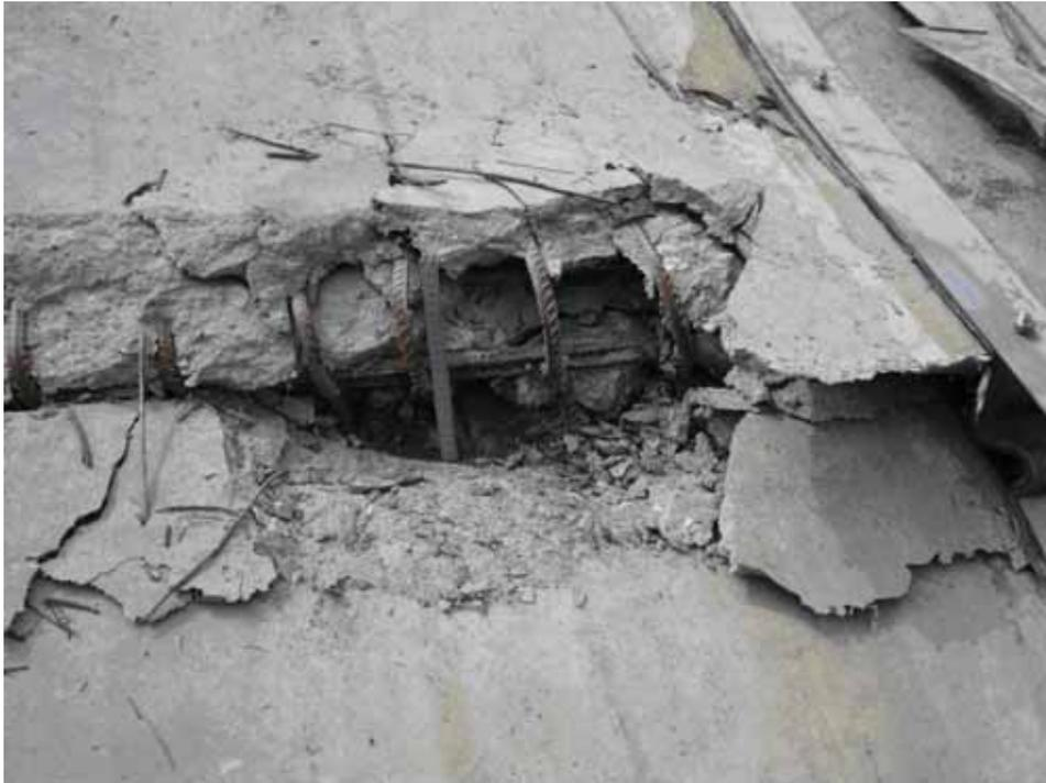
Figure 11. Highest horizontal construction joint detail (from Chen).
