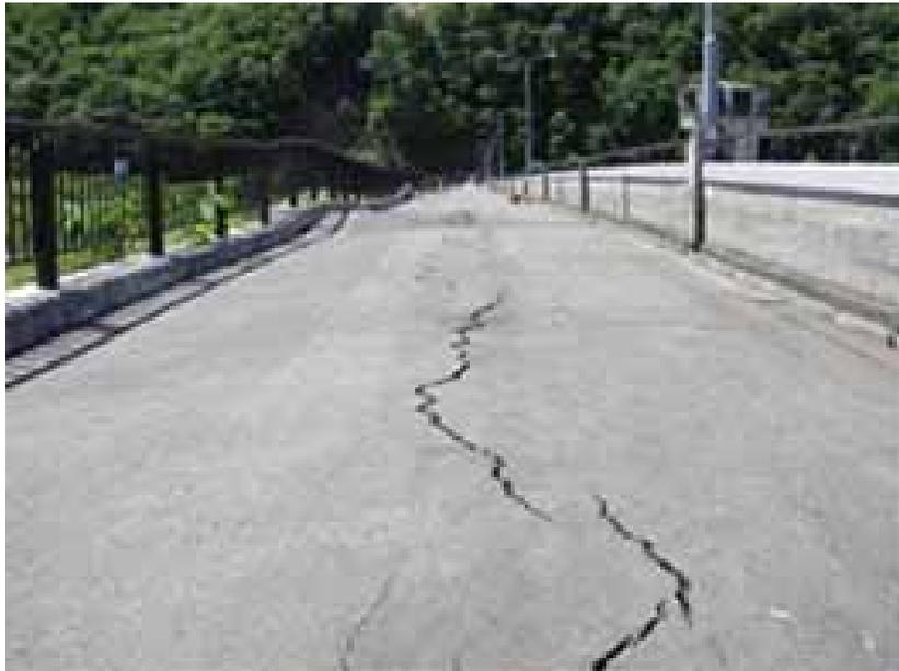
Figure 5. Dam crest – note waves in pavement (from Yamaguchi 2010).
