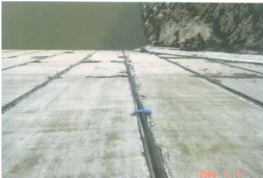
Figure 8. Face slab joint 5/6 near left abutment (from Wen).
