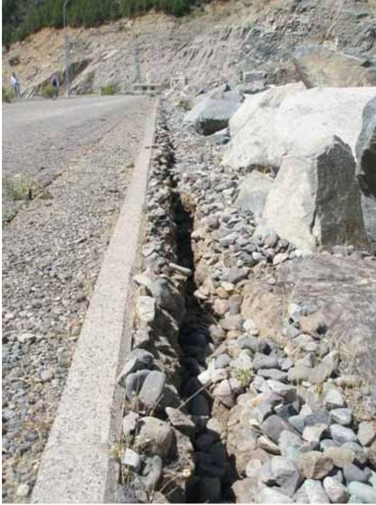
Figure 3. Longitudinal cracking on upstream side of crest (from Noguera, 2010)
