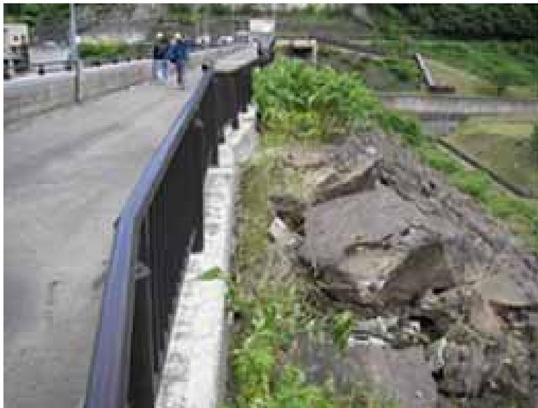
Figure 7. Displaced rock on downstream slope (from Yamaguchi, 2010).
