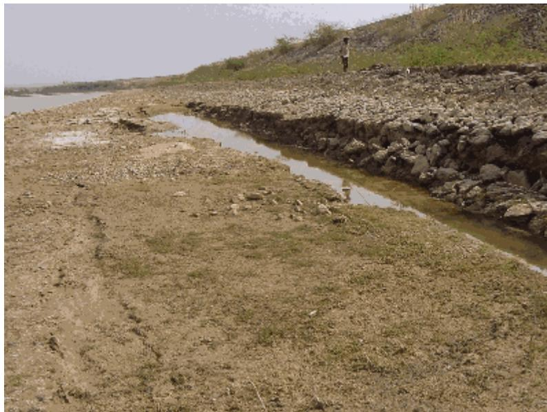
Figure 6. Lateral spreading occurred near the upstream Toe of Tapar Dam (from GEER, 2001).
