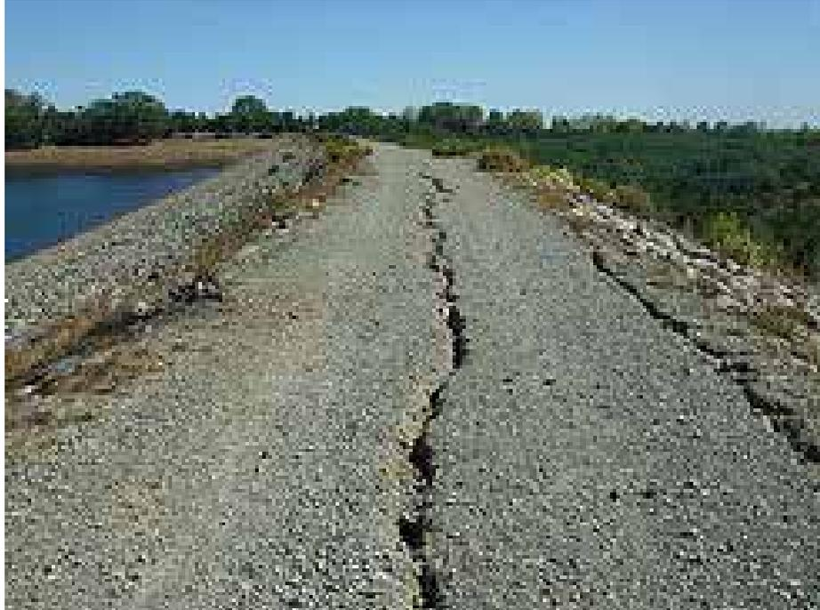
Figure 11. Crest cracking (from Bray et al., 2010).
