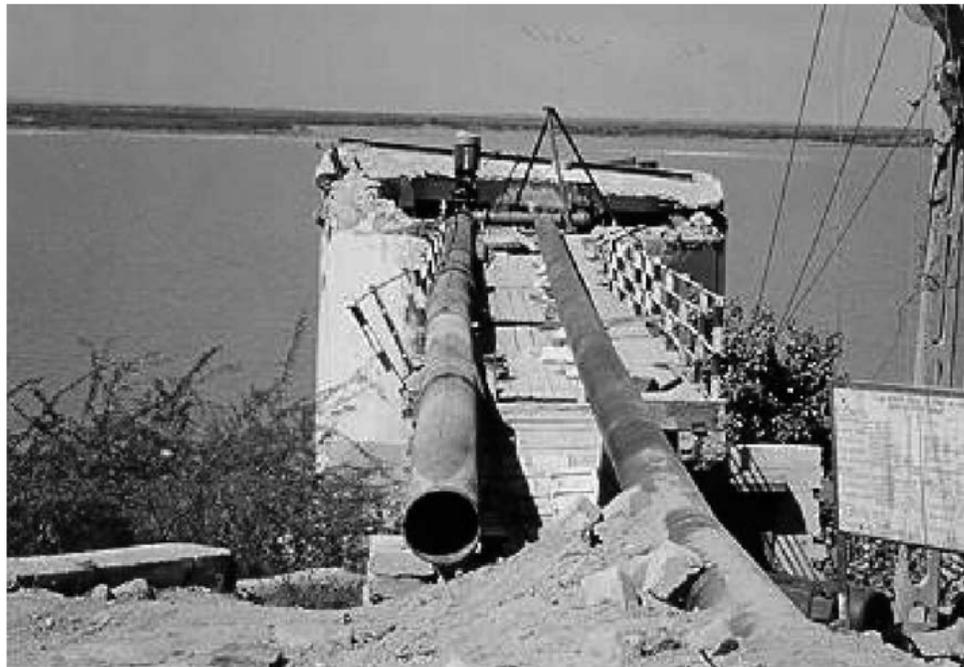
Figure 8. Damaged intake tower at Tapar Dam (from Krinitzsky and Hynes 2002).
