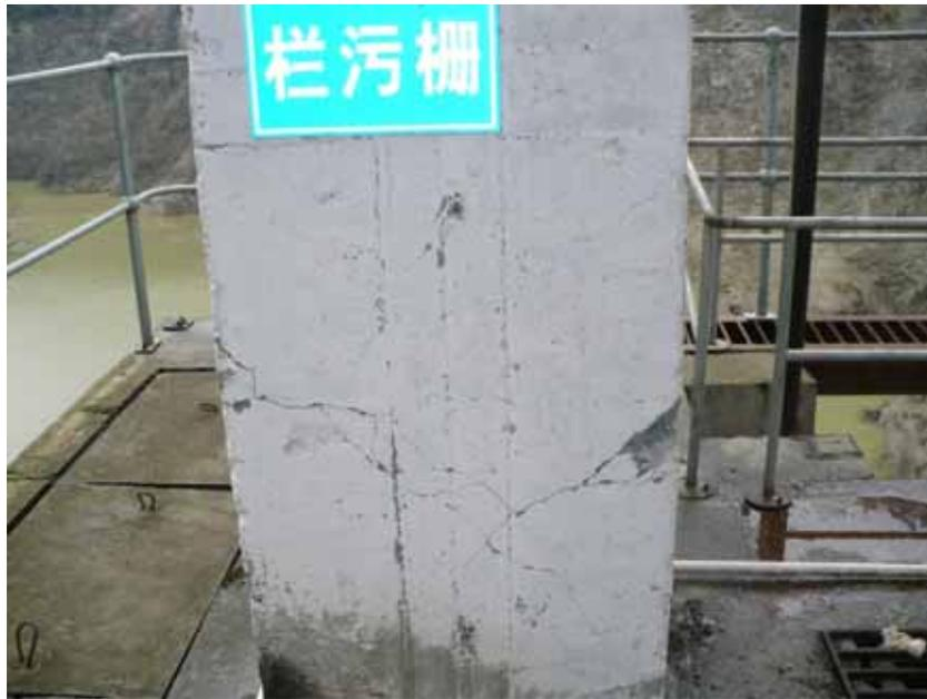
Figure 4. Cracking on gate hoist structure (Babbitt).
