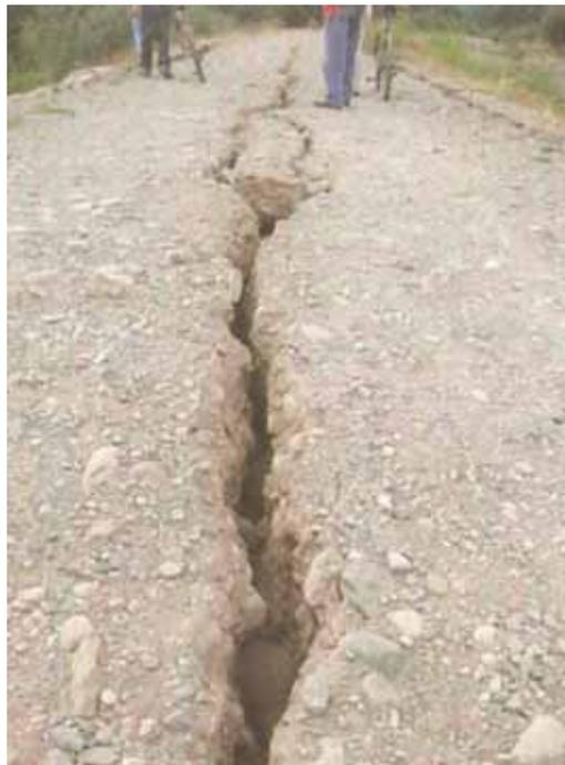
Figure 12. Crest cracking near right end of embankment (from Bray et al., 2010).
