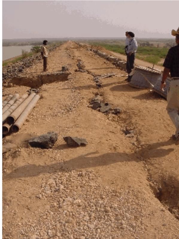
Figure 7. Longitudinal cracks occurred along crest of Tapar Dam. Excavation showed the cracks extended to a depth of 3 meters (from GEER, 2001).
