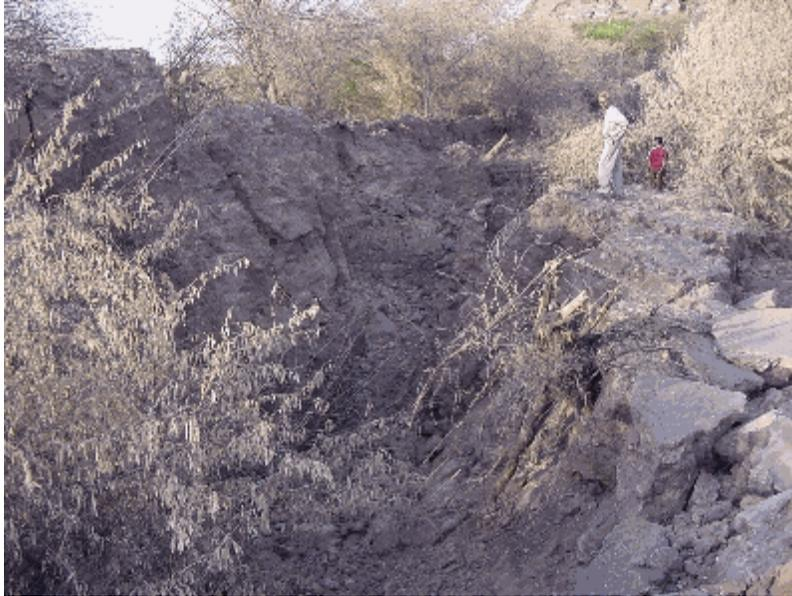
Figure 3. A large longitudinal crack, approximately 10 meters deep, was observed near crest of Chang Dam (from GEER 2001).
