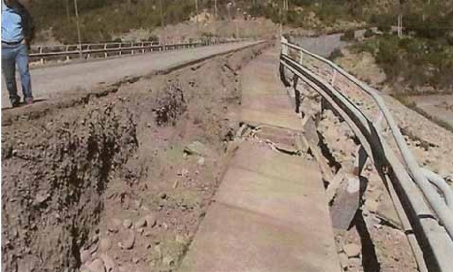
Figure 3. Displaced electrical conduit on downstream edge of crest (from Noguera 2010).
