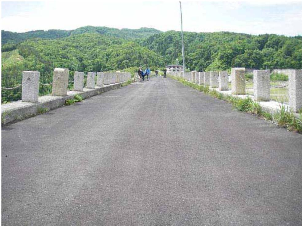
Figure 4. Dam crest showing tilting and fallen monuments (from Yamaguchi et al., 2008).
