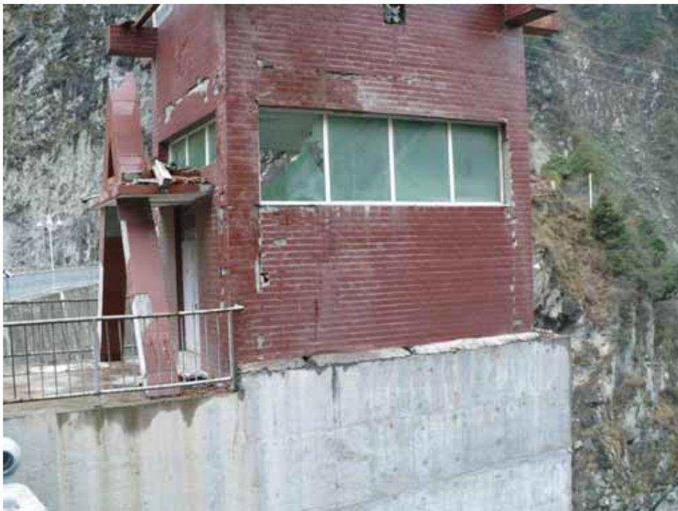
Figure 5. Damaged elevator shaft building (Babbitt).
