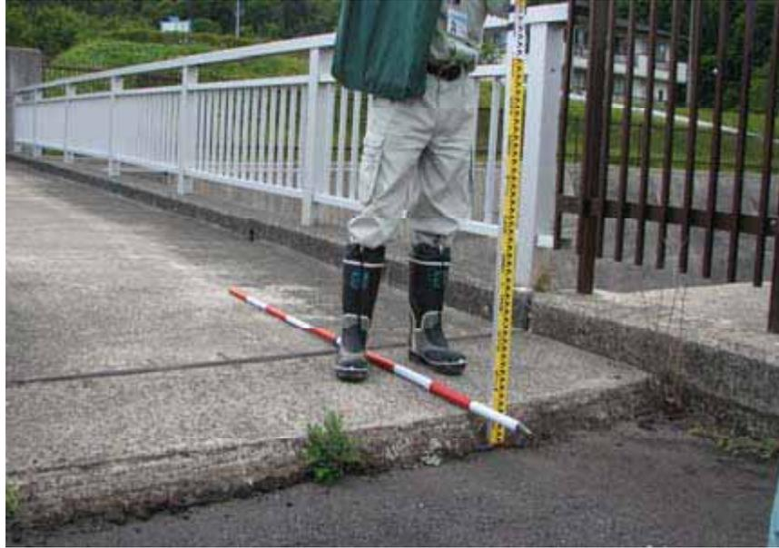
Figure 5. 10 cm of embankment settlement at the spillway (from Tani, et al., 2008).
