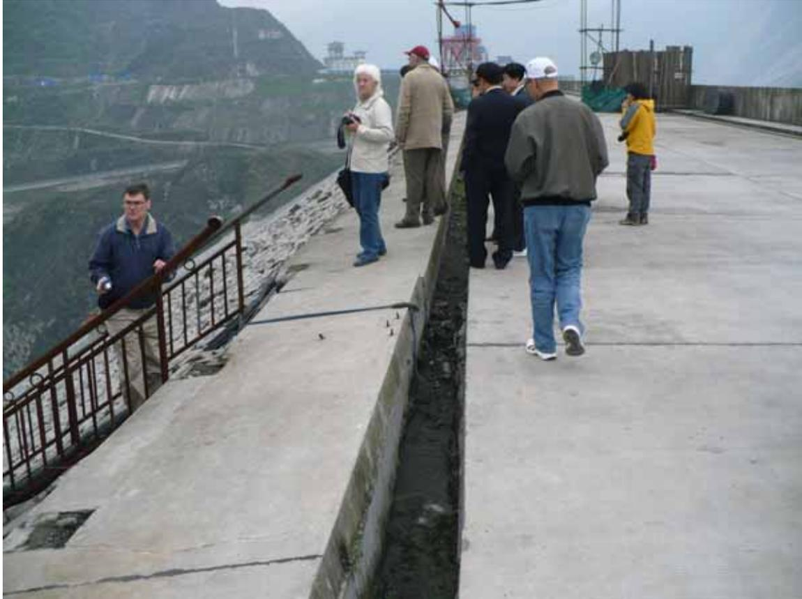
Figure 5. Gap at downstream edge of crest (Babbitt).
