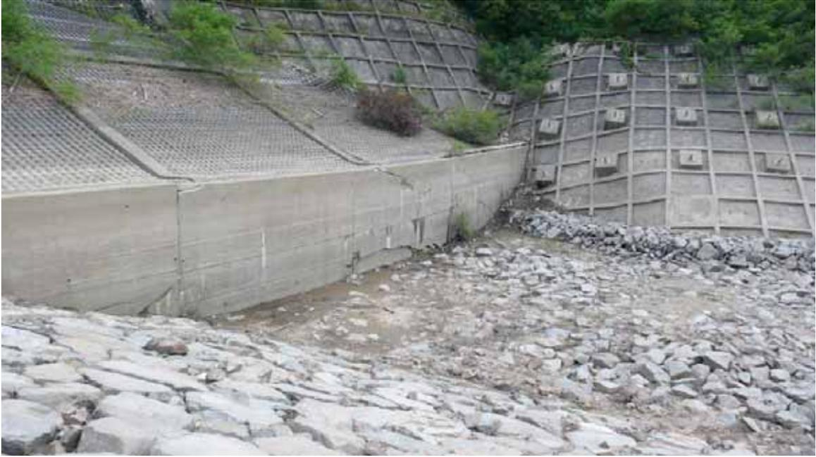
Figure 7. Cracking of spillway retaining wall structure (from Kayen et al., 2008).
