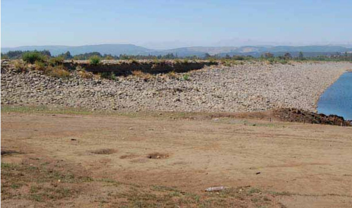
Figure 3. Slough A — near left abutment scarp at dam crest and bulge in lower right of photo (from Bray et al., 2010).
