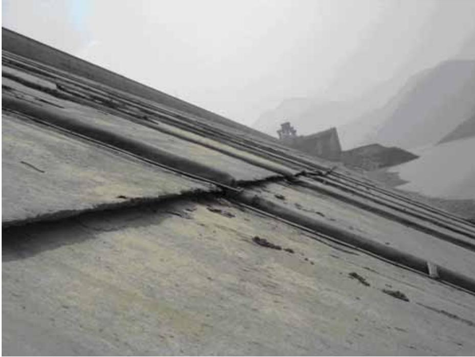
Figure 10. Highest horizontal construction joint (from Chen).
