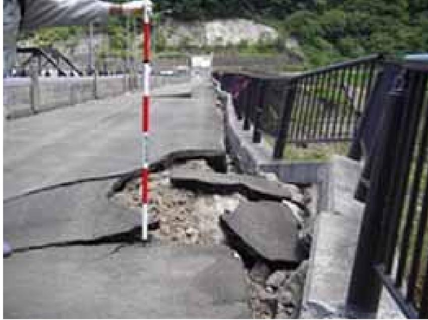
Figure 6. Deformation at downstream edge of crest. (from Yamaguchi, 2010).
