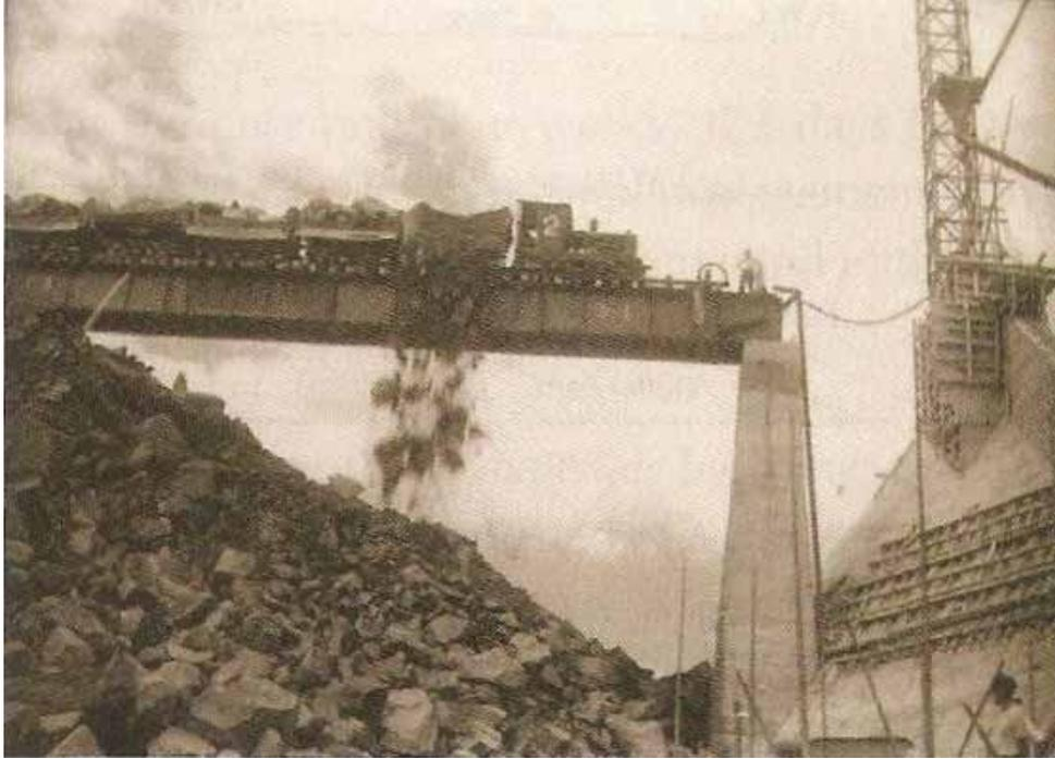
Figure 4. Rockfill construction – note pier and spillway wall (from JCOLD 2009).
