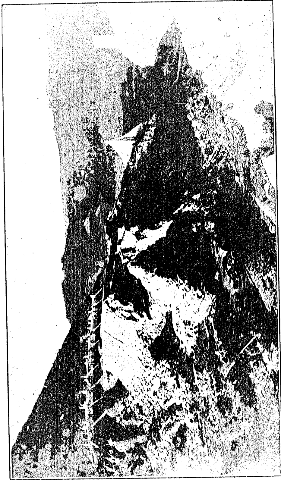
MAMMOTH DAM. Upstream view of North end of dam after failure, showing location of temporary spillway.
