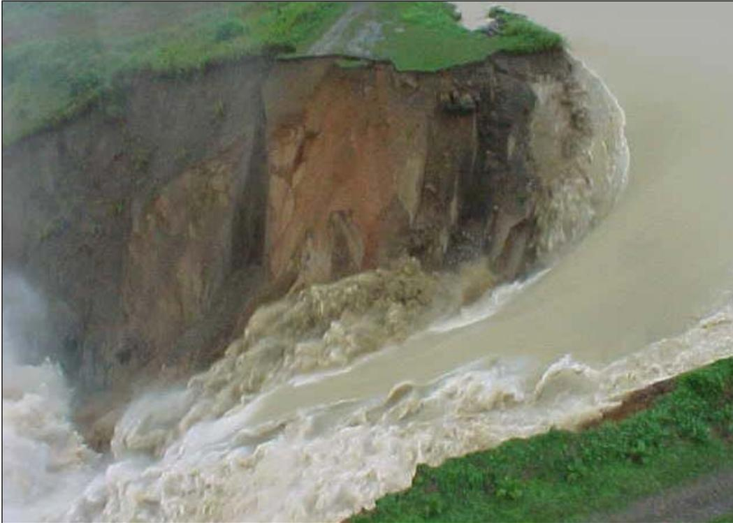
Figure F-2-11.—Headcutting progressed to reservoir.
