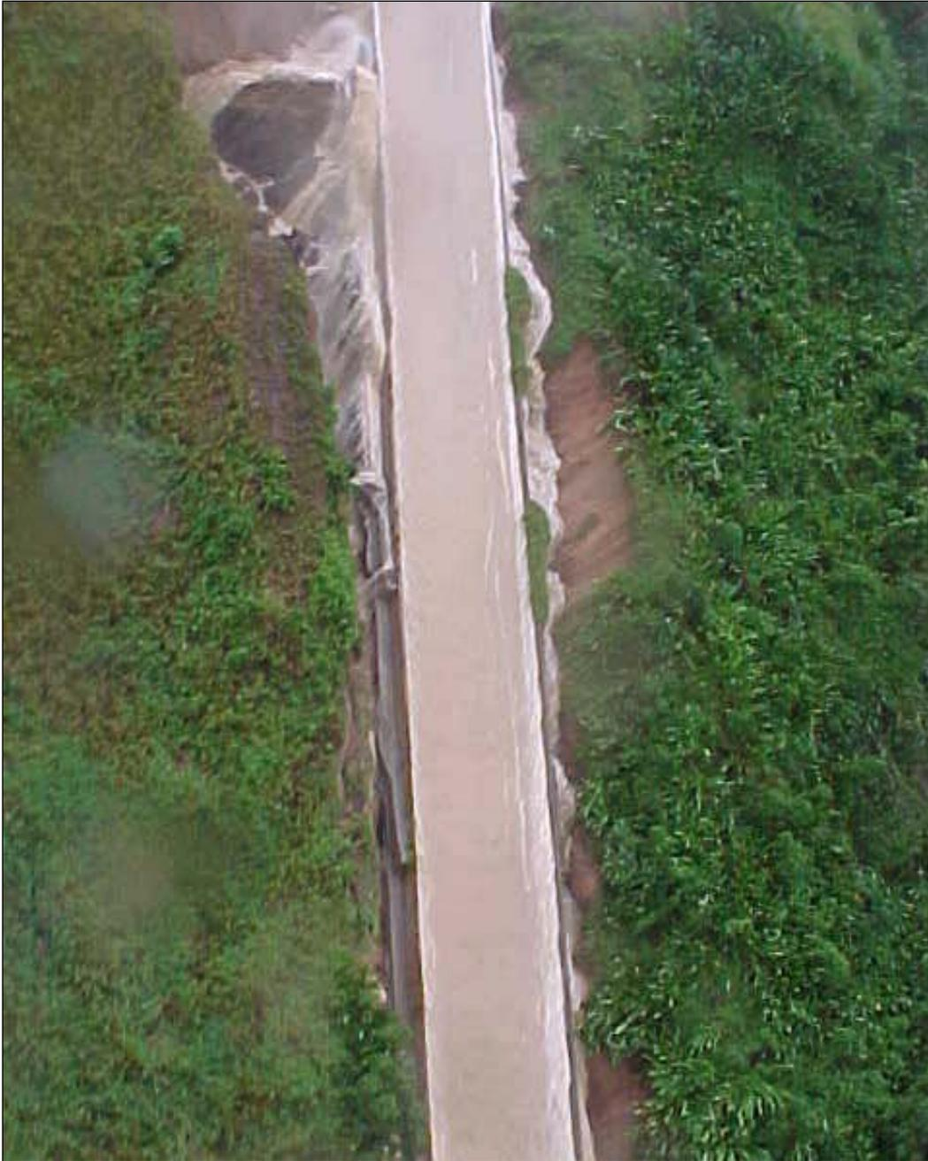
Figure F-2-10.—Overtopping of upstream chute walls.
