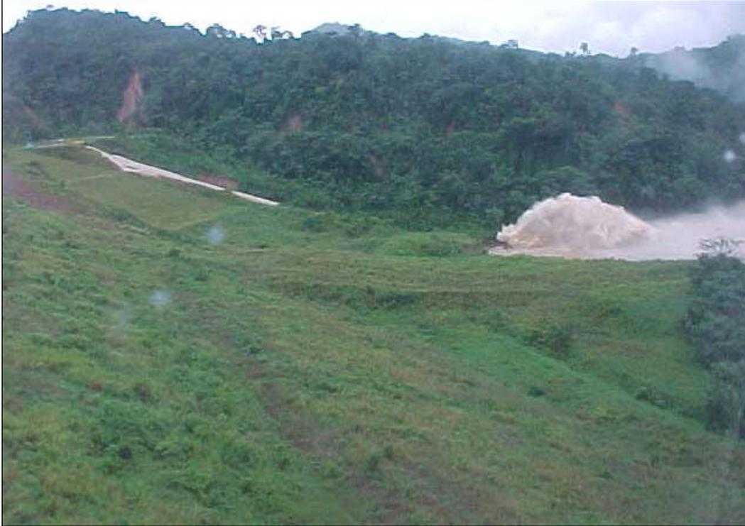
Figure F-2-8.—Sweepout of spillway stilling basin.
