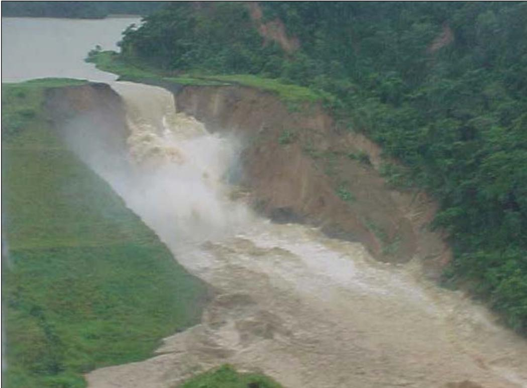
Figure F-2-12.—Breach formation nearing completion.
