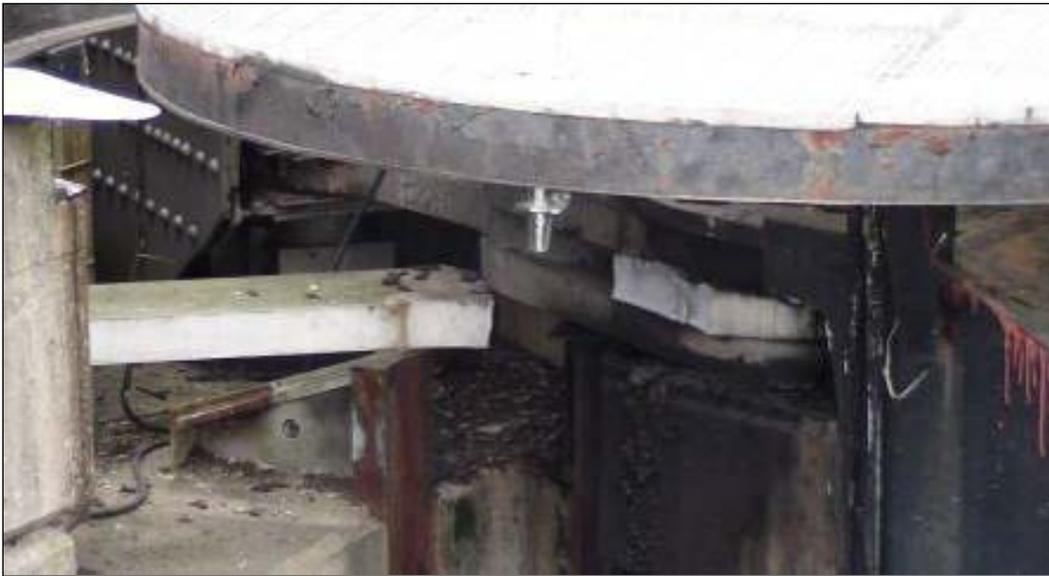
**Figure G-2-14.—Failed Anchor Arm, Greenup Lock and Dam (USACE 2010a).**
