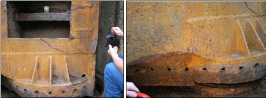
**Figure G-2-10.—Cracking in main chamber miter gates, Greenup Lock and Dam (USACE 2010a).**
