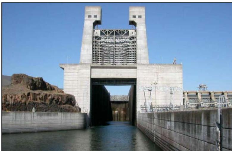
Figure G-2-7.—Overhead vertical lift gate.
