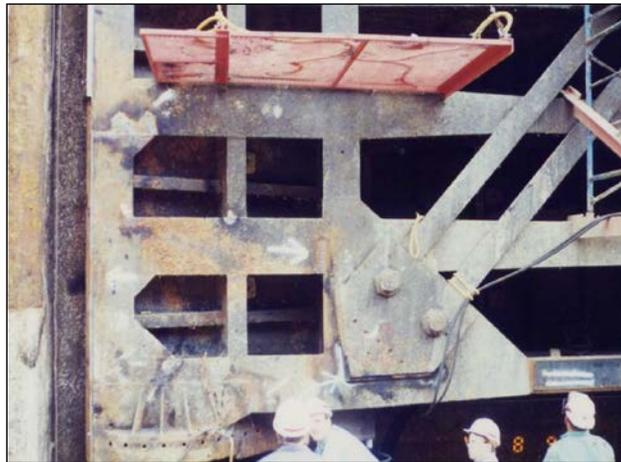
**Figure G-2-13.—Fatigue cracking in girder flange at diagonal anchor plate, Markland Lock and Dam (USACE 2010b).**
