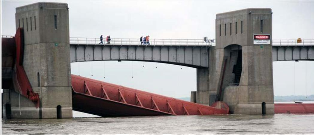
Figure G-2-18.—Damaged roller gate, Mississippi River Lock and Dam 25 (USACE 2011).
