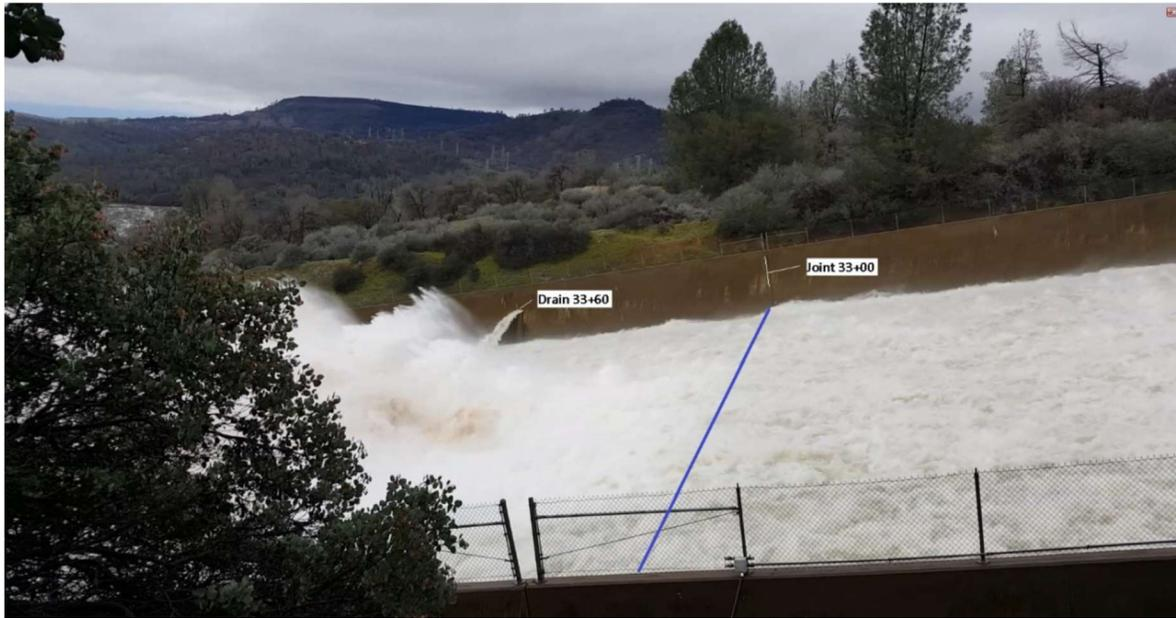
**Fig. 2.3.2 Water Splashing against Offset Downstream from Sta. 33+00**
