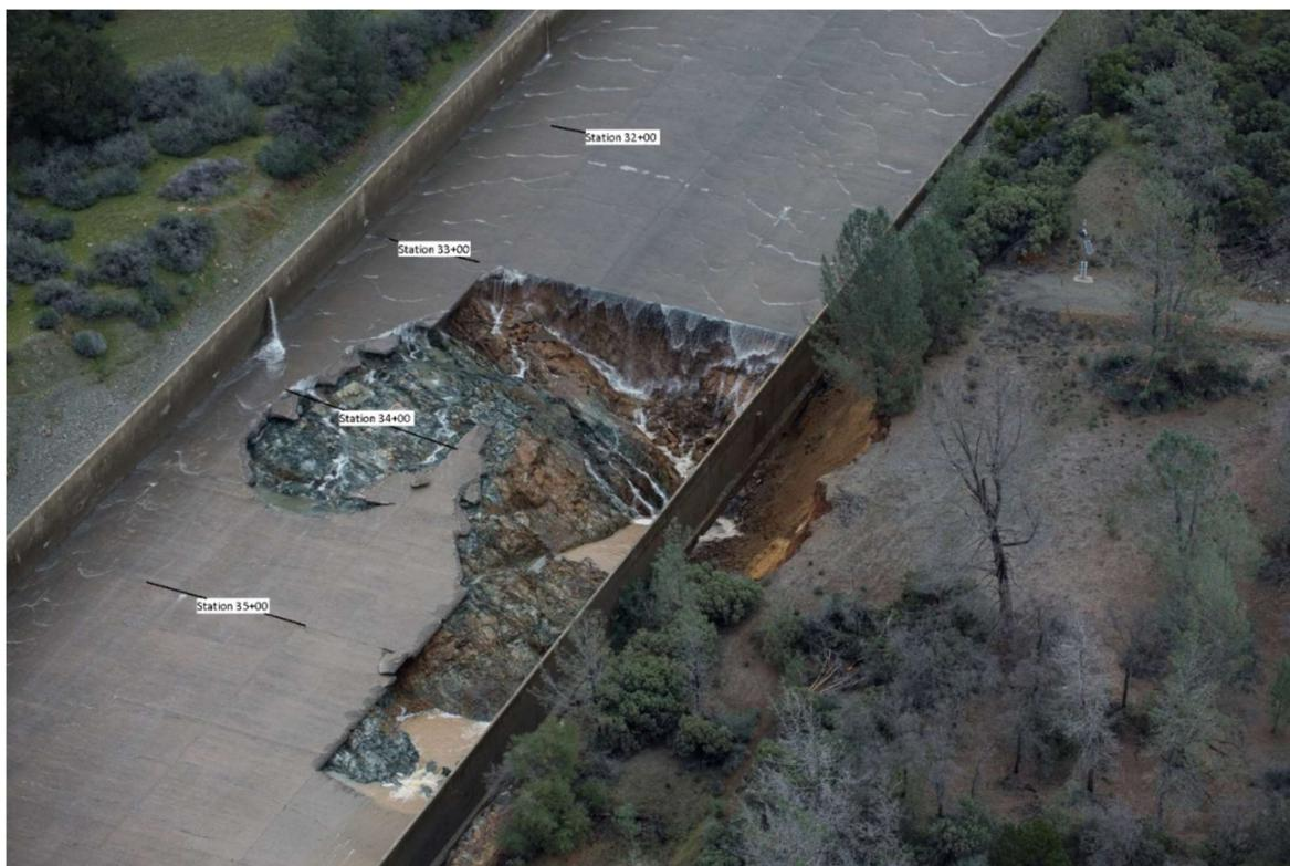
**Fig. 2.3.3 Initial Erosion Visible on February 8, 2017**
