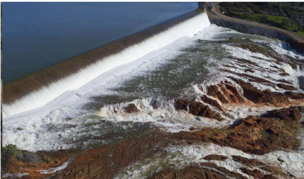
Figure 4-10: Emergency spillway head cutting on February 12 (from DWR)
