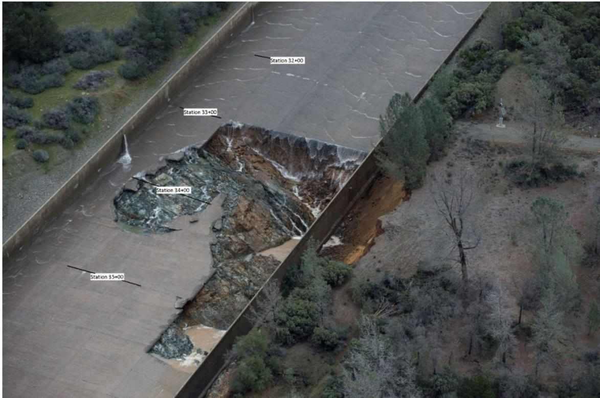
**Fig. 2.2.3 Initial Erosion Visible on February 8, 2017.**
