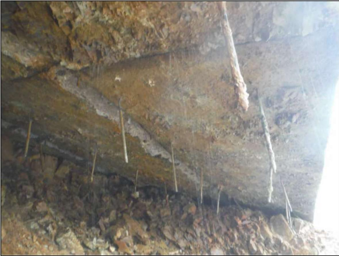
**Figure A-19: Anchor bars on the underside of the slab upstream of Sta. 33+00 (on right edge). Note the smooth underside of the chute slab that was to have been placed on a rock foundation which would have been expected to be irregular. (Photo DSCF9788)**
