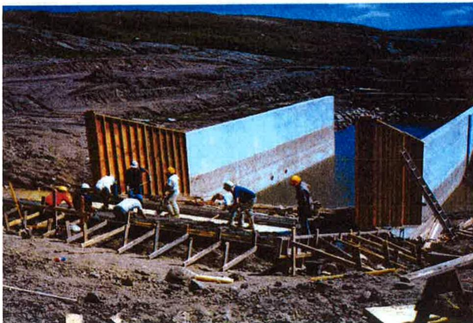
2. Looking downstream and to the left at formwork for the Segment D slab. Note the concrete forms that temporarily enclose the drain system will be subsequently removed and lack of backfill to provide lateral confinement of the drain system.
