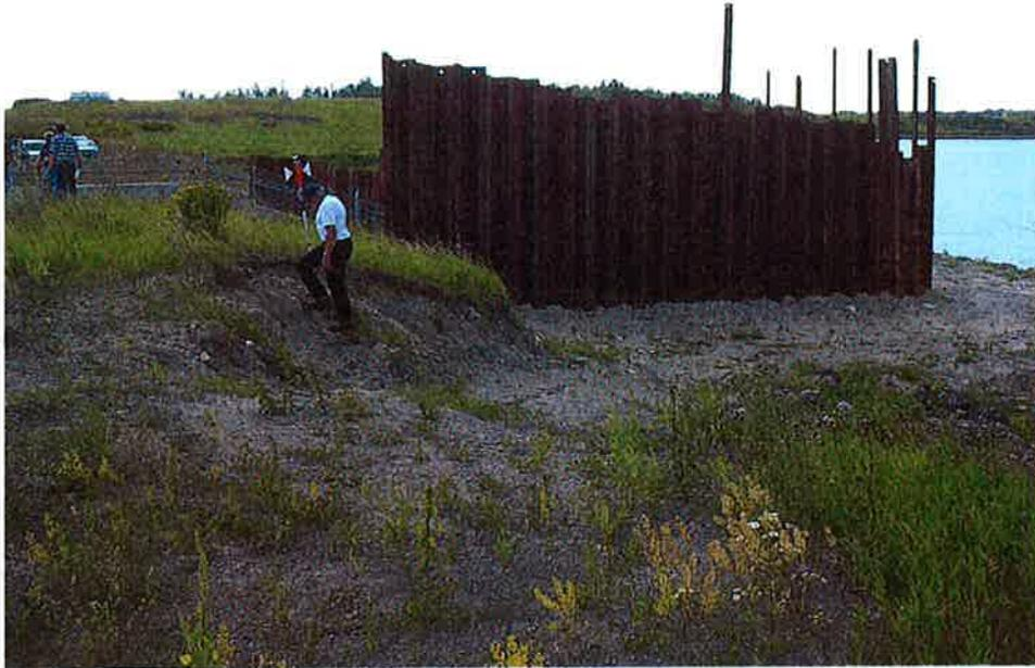
1. Looking right along crest at the temporary berm and sheetpile protection for the drop inlet structure.
