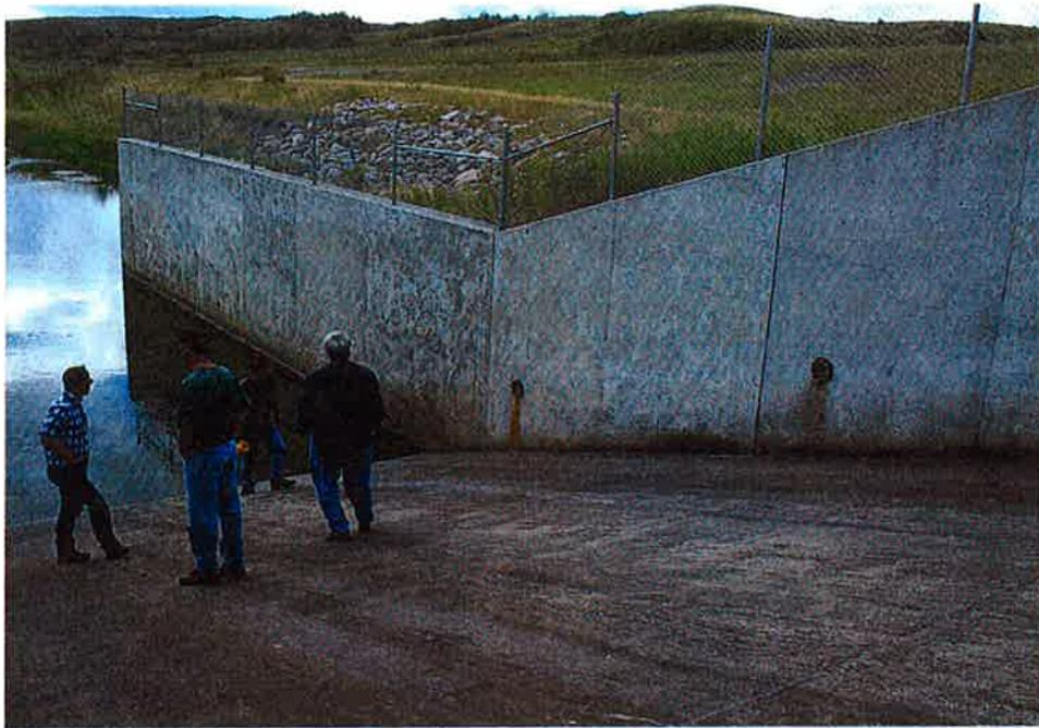
5. Looking downstream and to the right at spillway chute and right wall. Spillway underdrain outlets for Segment E and D are visible, whereas the outlet for Segment C is beneath the tailwater in the stilling basin.
