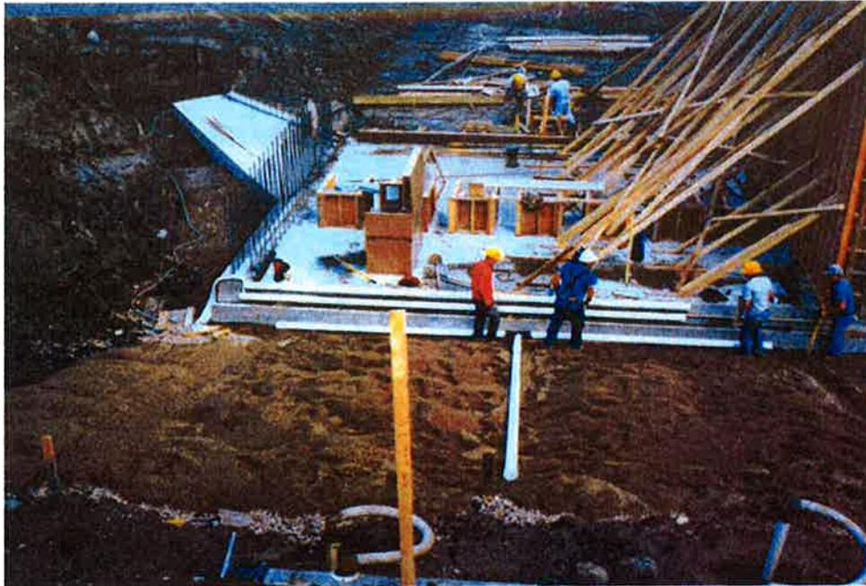
1. Looking downstream at construction of underdrain for Segment B. Note lack of lateral confinement of fine drainfill material. Note 1-1/2-inch-minus gravel used for subgrade stabilization beneath fine drainfill.
