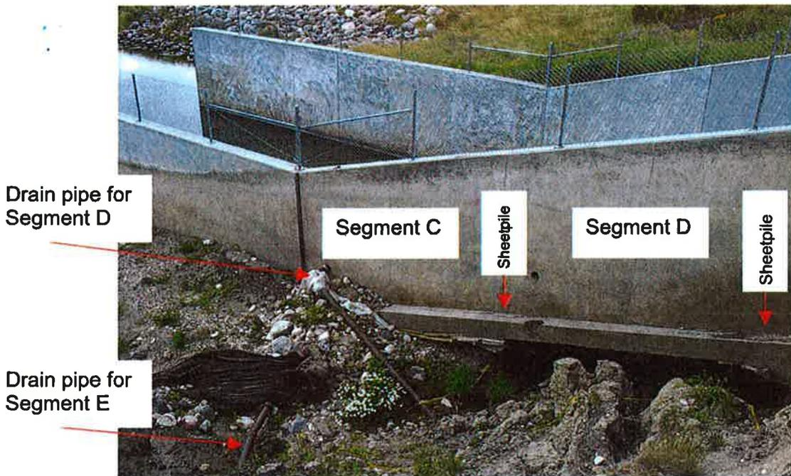
8. Looking downstream and to the right at left wall of chute and void beneath structure. Note the displaced ductile iron pipe drain pipes. Note black geotextile that envelops a gravel drain installed to control seepage during construction.
