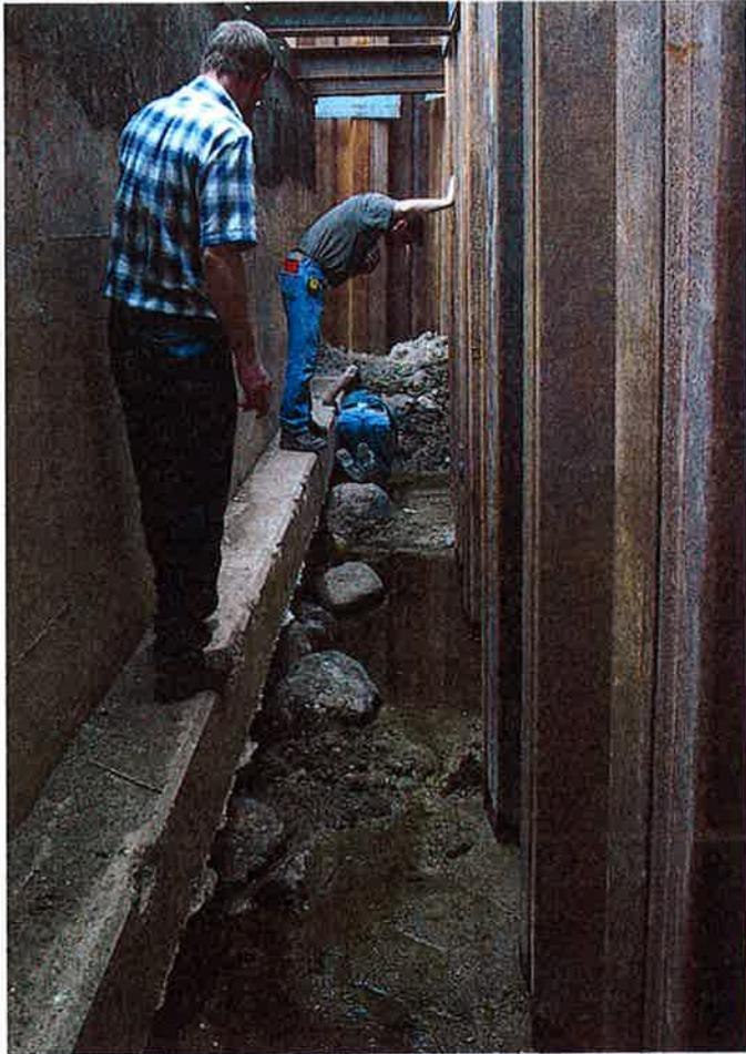
3. Looking right along upstream footing of principal spillway intake structure. Note up to 2-foot-deep void beneath slab. Note riprap that has fallen under slab. All remaining backfill and riprap was removed for installation of emergency sheetpile cofferdam.
