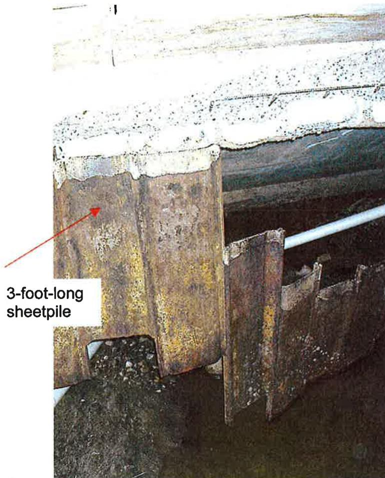
10. Looking downstream and right at sheetpiles for Segment D/E joint. Note undermined sheetpiles have fallen down from broken slab embedment. Note short sheetpile (only 3-foot long) versus 4-foot length specified. Note displaced PVC drain pipe beneath Segment D.
