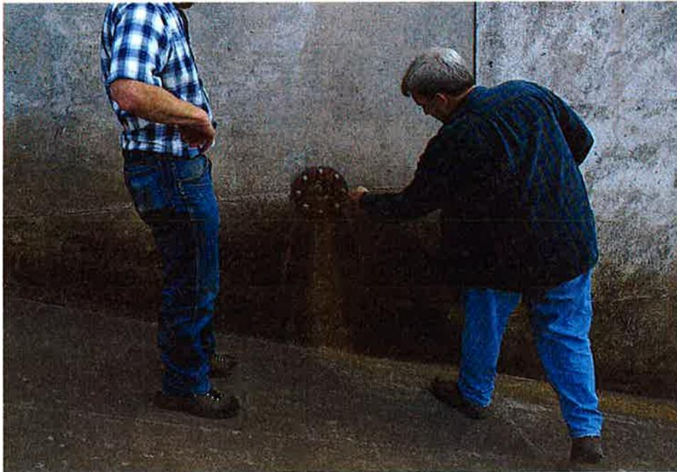
6. Looking to the left in the spillway chute at the outlet for spillway underdrain Segment E. Note the increased concrete staining that has occurred at this location compared to the outlets in Photos 5 and 7.
