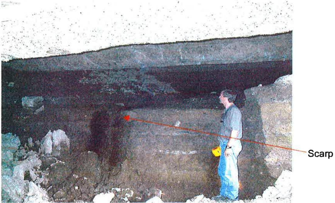
7. Erosion under Segment F. Note 5-foot-high scarp likely resulting from headcutting. Embankment fill is exposed in scarp.
