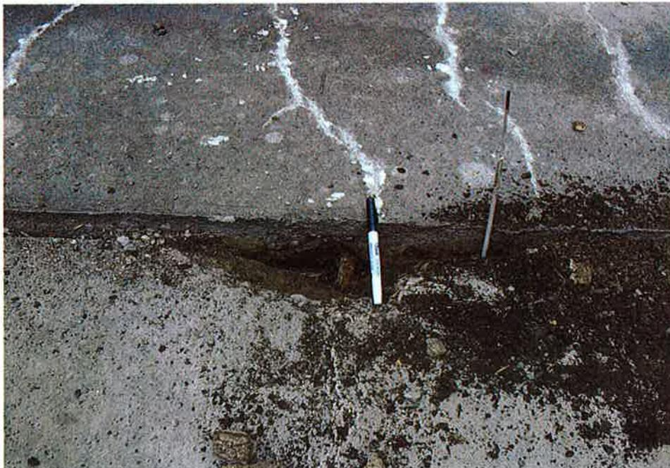
15. Close-up view of slab joint K/L. The waterstop visible to left of dowel is no longer embedded on upstream edge.
