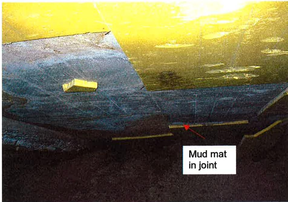
9. View of underside of slab Segment E and rigid insulation board. Two layers of 2-inch-thick insulation were installed during construction. Note concrete mud mat in joints between insulation panels.
