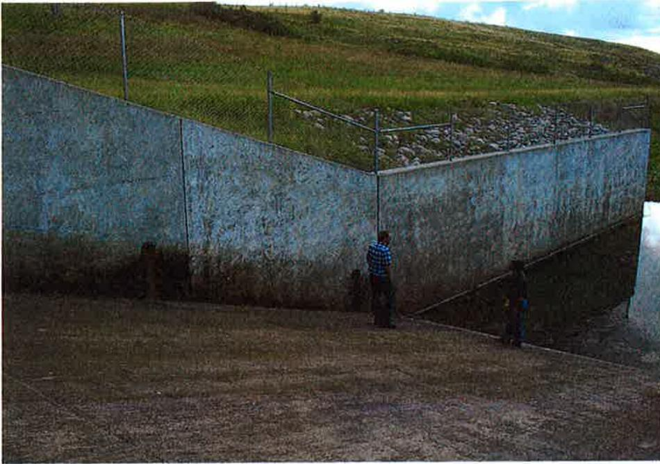
7. Looking downstream and to the left at spillway chute and left wall. Spillway underdrain outlets for Segments E and D are visible, whereas the outlet for Segment C is beneath the tailwater in the stilling basin. Note increased concrete staining at the outlet for Segment E. See close-up Photo 6.
