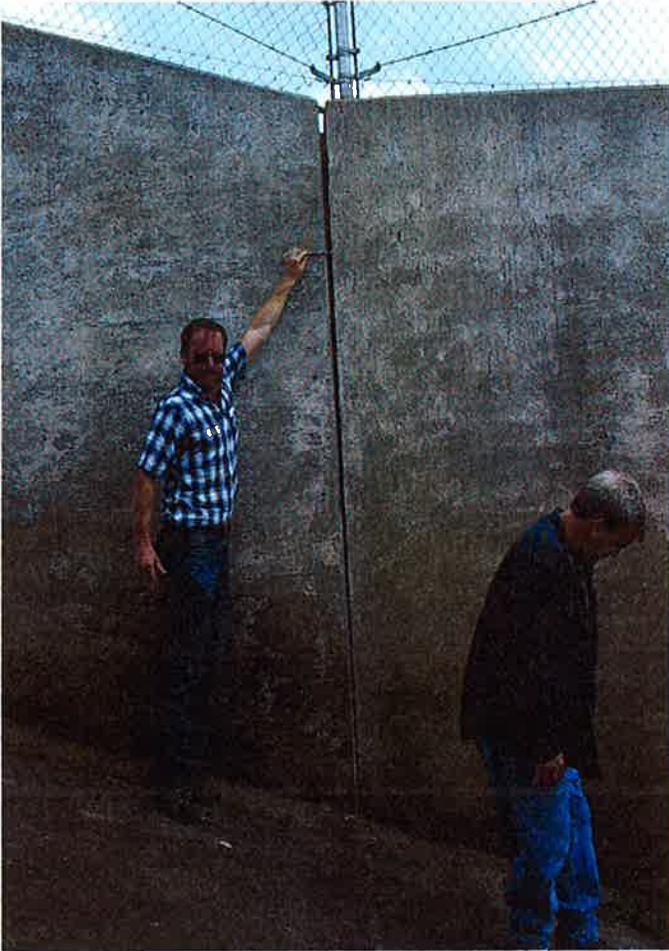
**17. Joint displacement between Segments B and C on left wall of principal spillway.**
