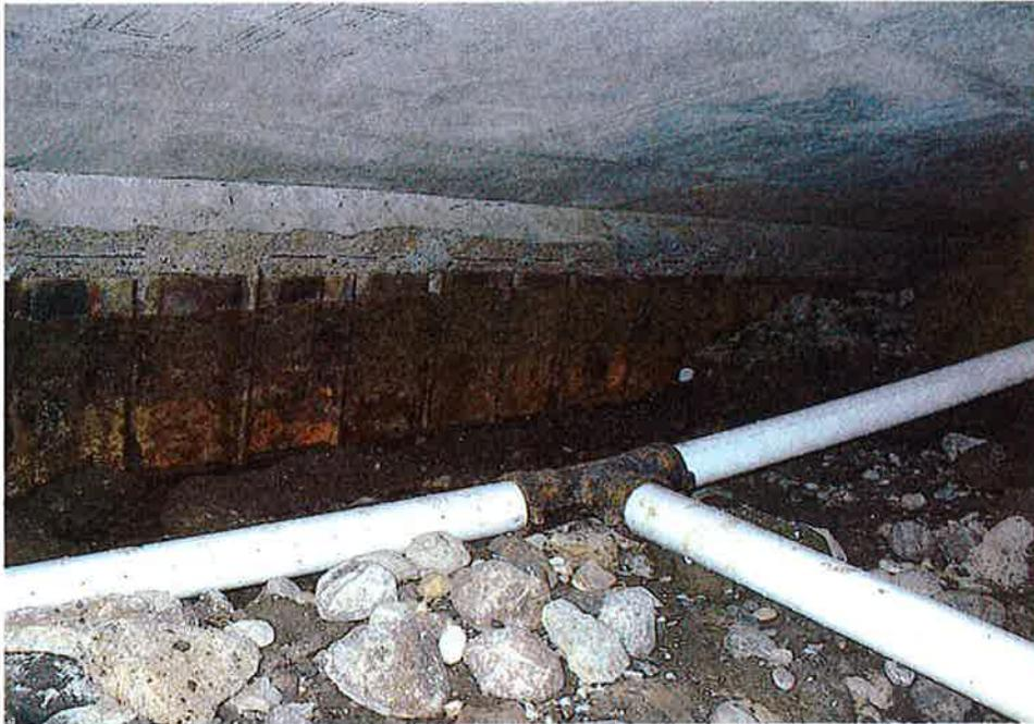
11. Looking downstream and to the right at sheetpiles for Segment C/D. Note 4-inch-diameter underdrain lying in foreground.
