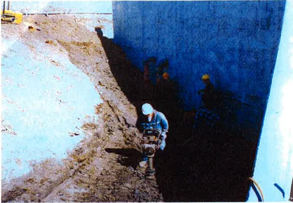
3. Backfill compaction using lightweight equipment adjacent to stilling basin Segment A. Photo looking upstream and to the left. Note exposed underdrain discharge pipes and insulating wrap.
