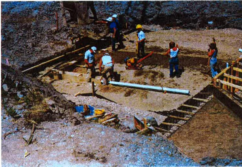
4. Placement of fine drainfill for Segment A stilling basin. Note the perforated drain pipe supported at grade before coarse drainfill is placed around the pipe using the guide forms. Note the fine drainfill is placed over 1-1/2-minus gravel foundation stabilization material and a non-woven geotextile that was installed to address wet subgrade conditions. Photo taken looking upstream and to the left.
