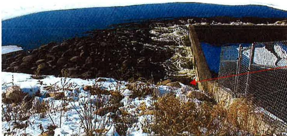
2. Photo taken March 30, 2003 during erosion failure. Looking upstream at right wall of drop inlet structure. Note water flowing over riprap berm and down along all sides of the drop inlet. Note location of large erosion hole on right side of structure. Photo provided by NDSWC.
