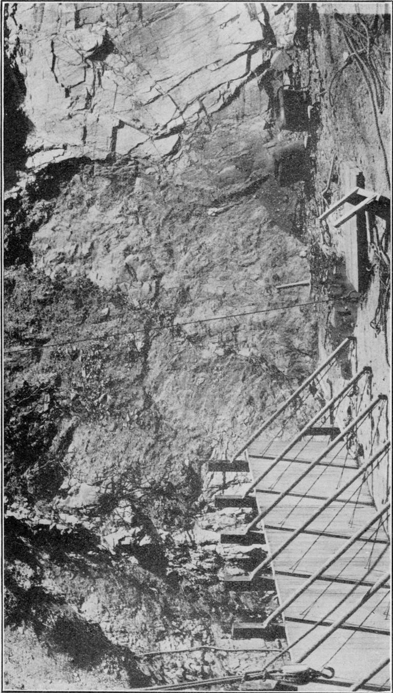
CONSTRUCTION VIEW SHOWING SHAPING OF EAST ABUTMENT AT UPSTREAM WALL.
