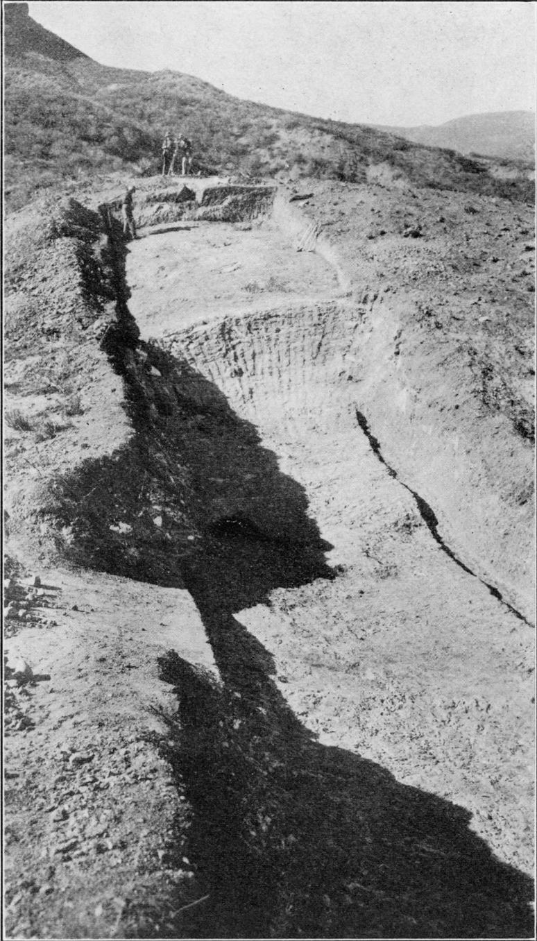
EXCAVATION FOR WING WALL SECTION.
