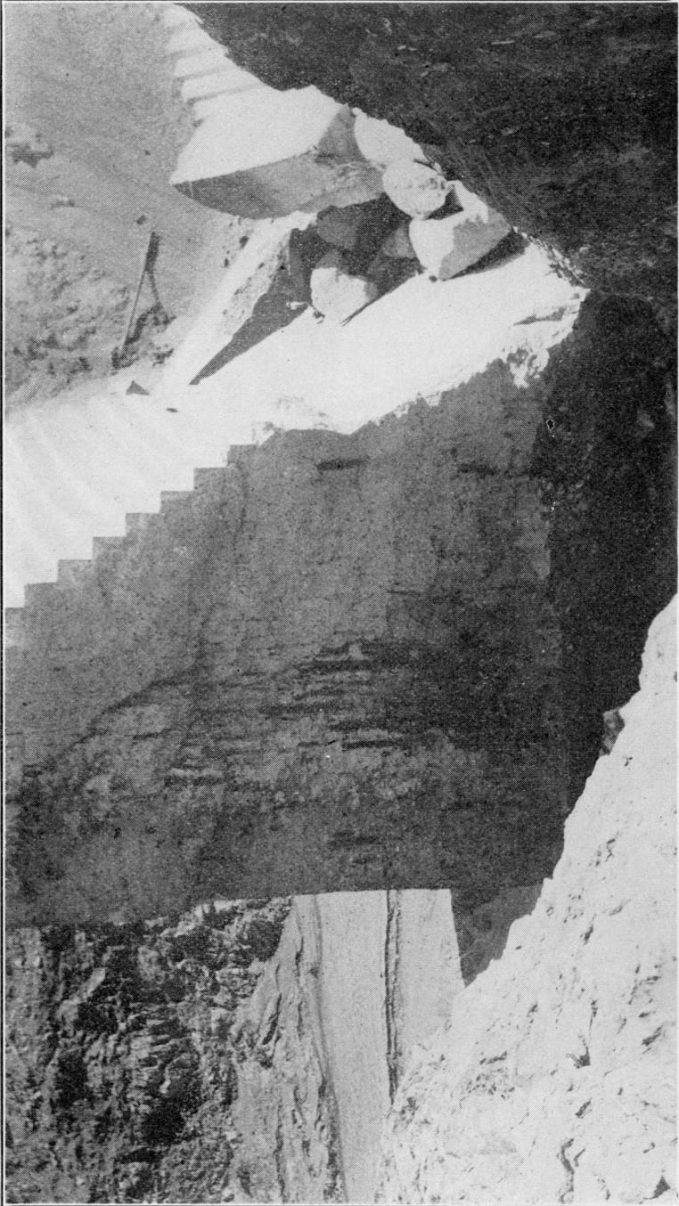
WEST FACE OF STANDING SECTION SHOWING CONTACT PLANE WITH FOUNDATION.
