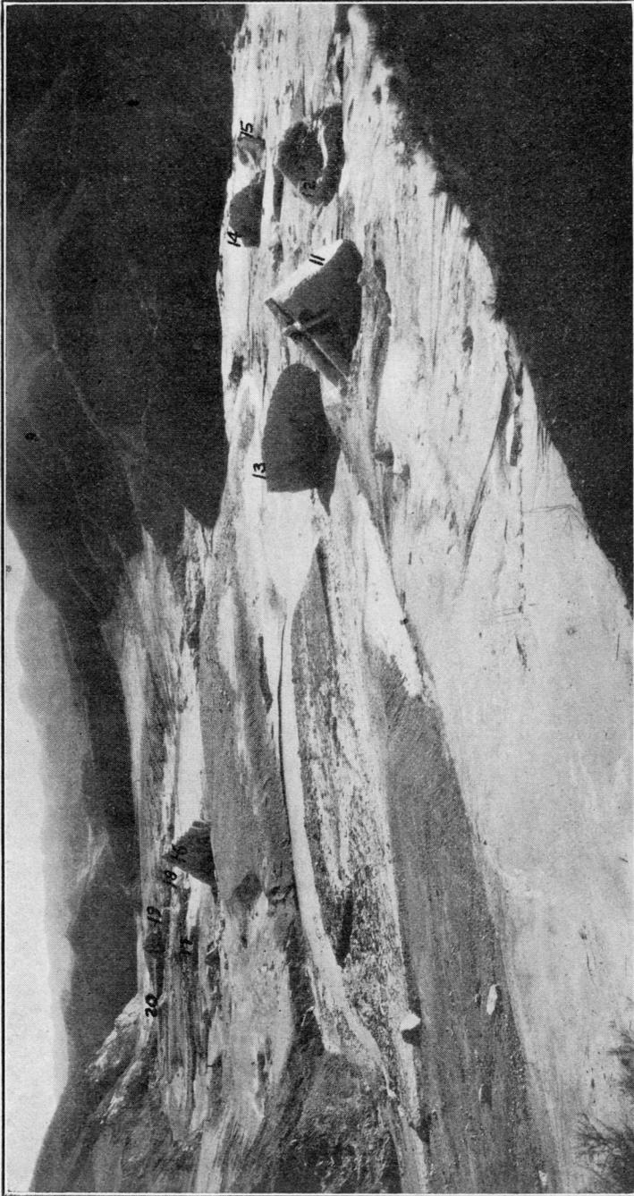
CONCRETE FRAGMENTS OF DAM DEPOSITED DOWNSTREAM BY FLOOD WAVE.
