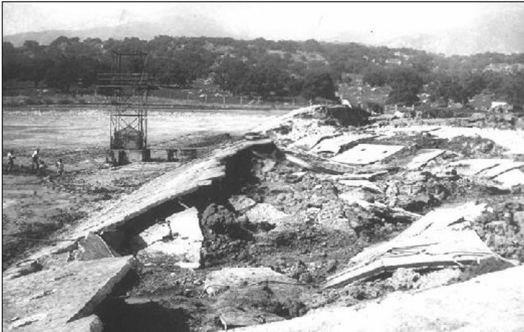
Figure D-8-3.—Sheffield Dam after 1925 earthquake (courtesy of National Information Service for Earthquake Engineering, University of California, Berkeley).
