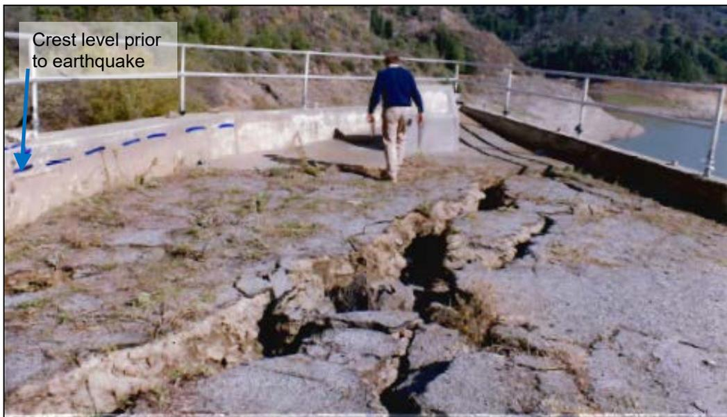
Figure D-8-4.—Settlement and cracking at Austrian Dam in area of spillway wing wall (courtesy of Sal Todaro).
