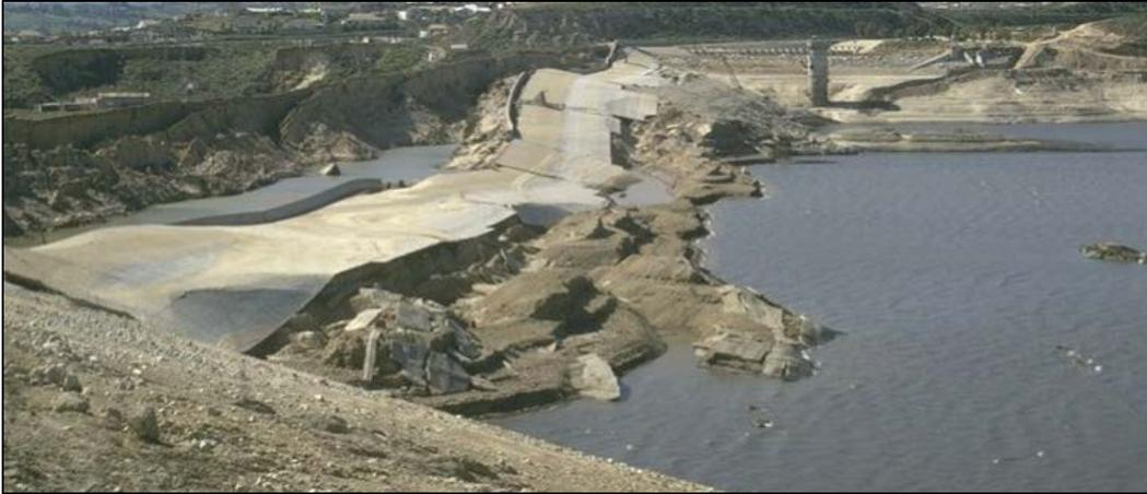
Figure D-8-1.—Lower San Fernando Dam after 1971 earthquake (courtesy of National Information Service for Earthquake Engineering, University of California, Berkeley, Karl Steinbrugge Collection).
