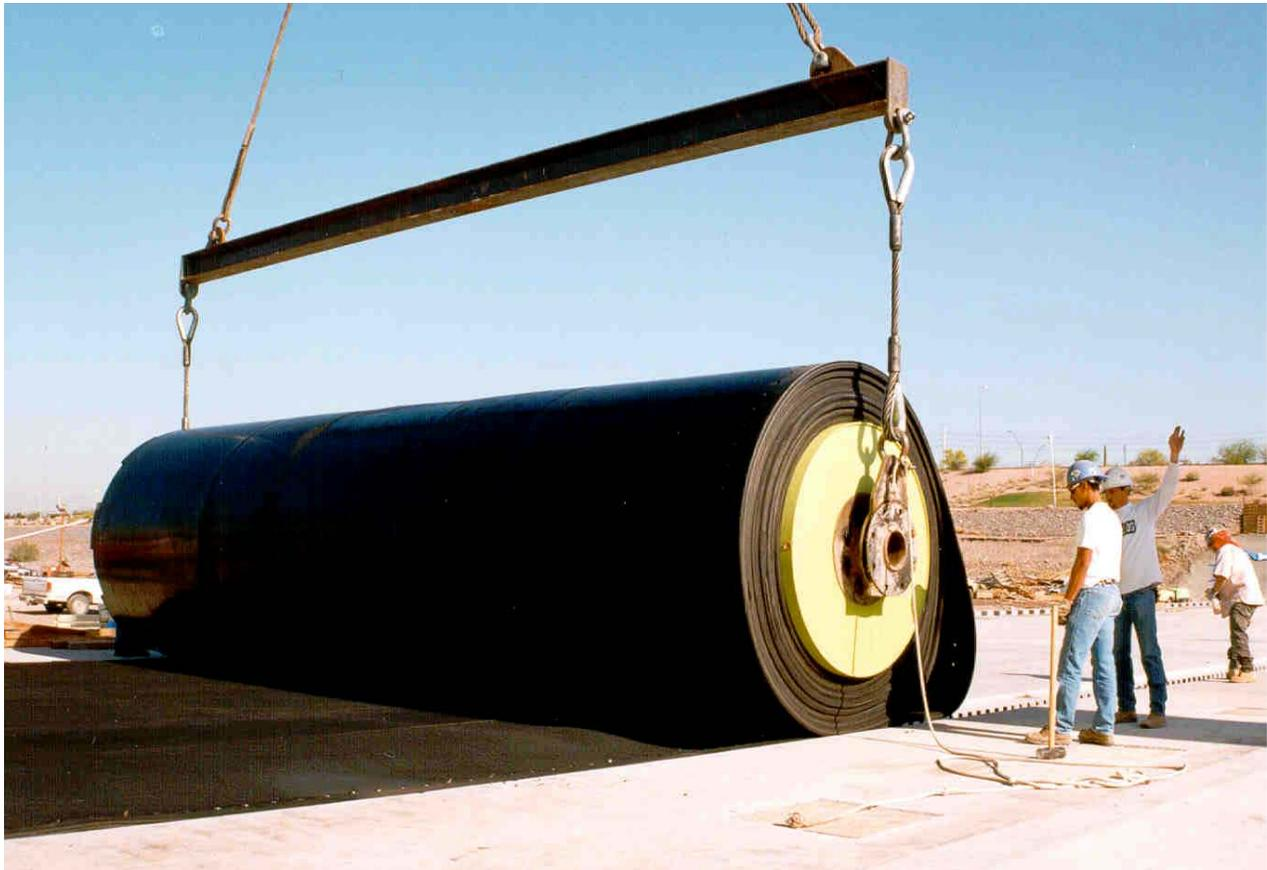
Figure 5. Rubber bladder being positioned on dam foundation
