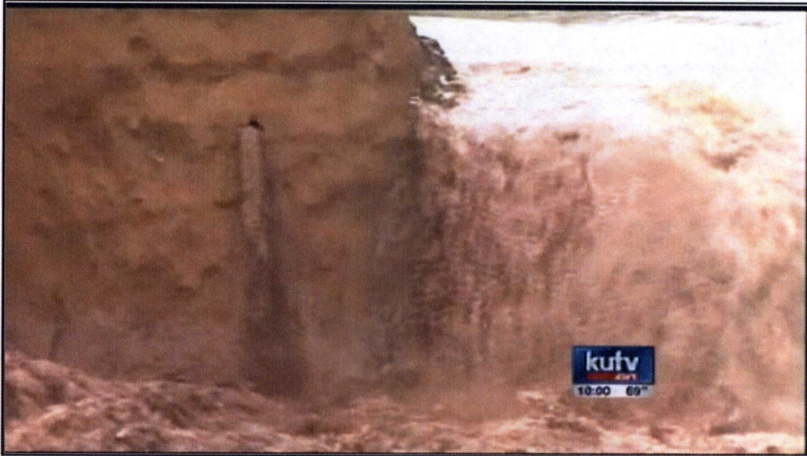
Photograph 7 – Concentrated flow through hole into breach
