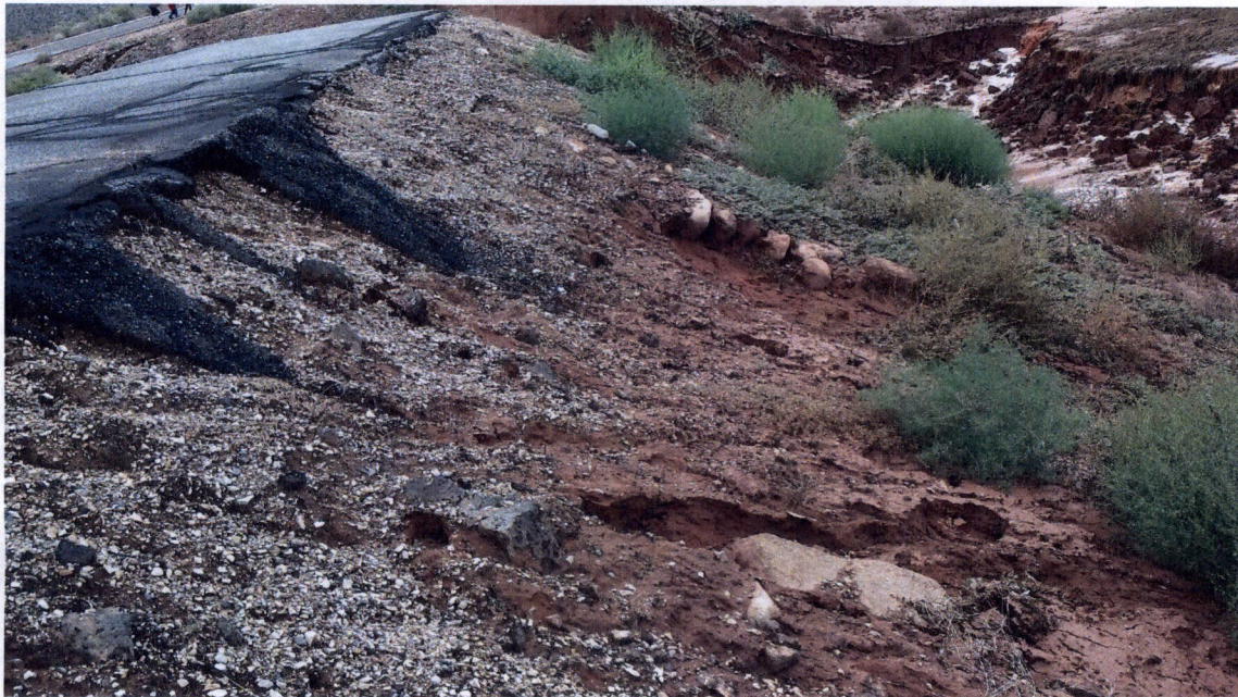
Photograph 8 – Post breach, rodent holes with gully from backflow
