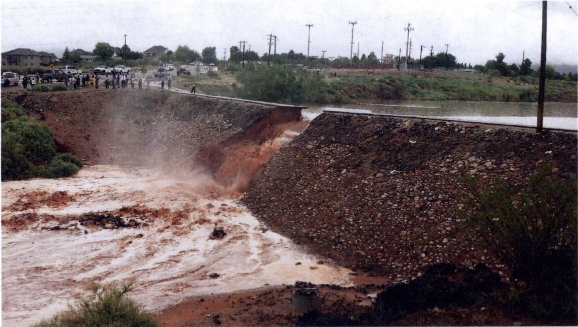
Photograph 3 – Failure progression
