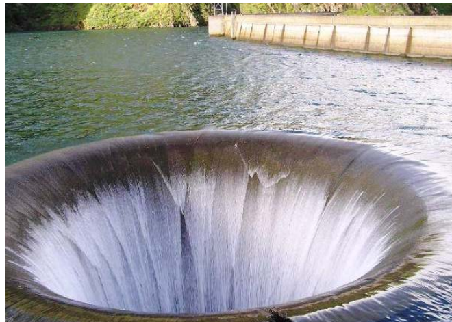
Photo 1: A glory hole is one type of drop inlet
