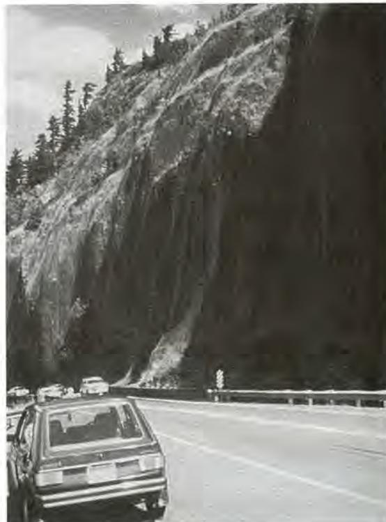
FIGURE 18-21 Wire mesh hung on vertical face to direct falling rock into ditch at toe of slope.
