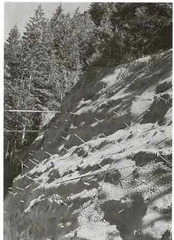
to be able to stand in a vertical cut of about 2 m without failure or excessive deformation. Thus, soil nailing is generally not cost-effective or practical in loose granular soils and very soft clays (Mitchell and Christopher 1990). A high groundwater table may also present construction difficulties.
