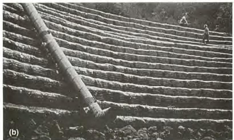
FIGURE 17-19 La Honda, California, landslide repair using geogrids: (a) under construction and (b) completed slope face.
