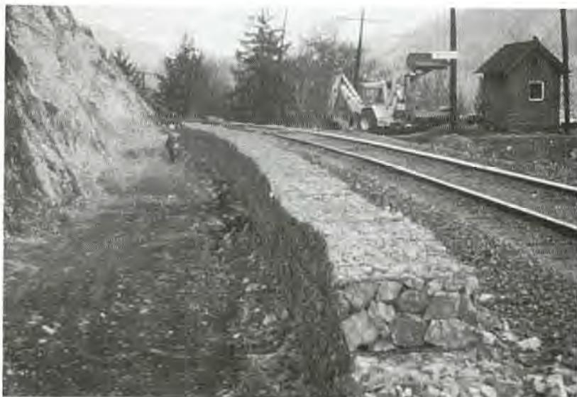
rubber tires (Figure 18-17). The capacity of a barrier of this type to stop rock falls depends on its mass in relation to the impact energy and on its capacity to deform without failing. The deformation may be both elastic deformation of the barrier components and shear displacement at the fabric layers or on the base.
