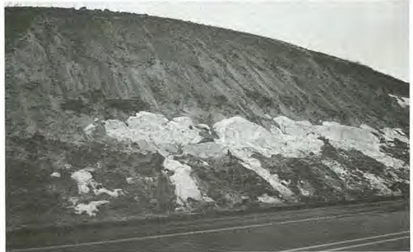
FIGURE 23-21 Failure of slope under melting snowdrifts on US-195 near Pullman, Washington.
