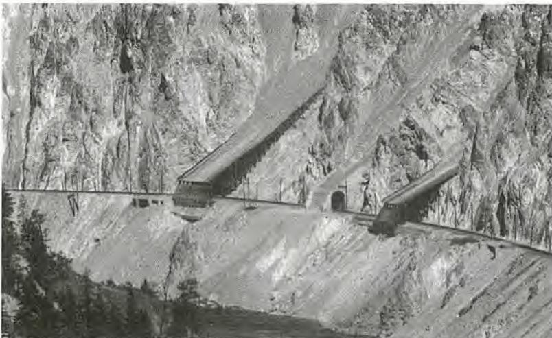
Alternatively, a lighter-weight crushable element, such as a cellular metal panel, may be used. The columns supporting the lower end of the roof are founded on rock-socketed piers that extend through the fill into sound rock. This type of foundation provides the required support with minimal settlement.
