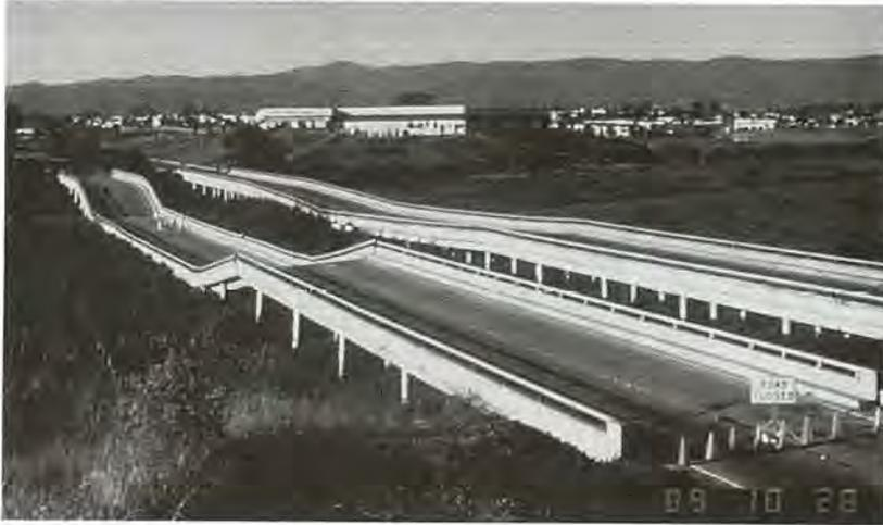
FIGURE 4-15 State Highway 1 bridge destroyed by strong shaking and liquefaction of river deposits at Struve Slough near Watsonville, California, during 1989 Loma Prieta earthquake (Plafker and Galloway 1989).
