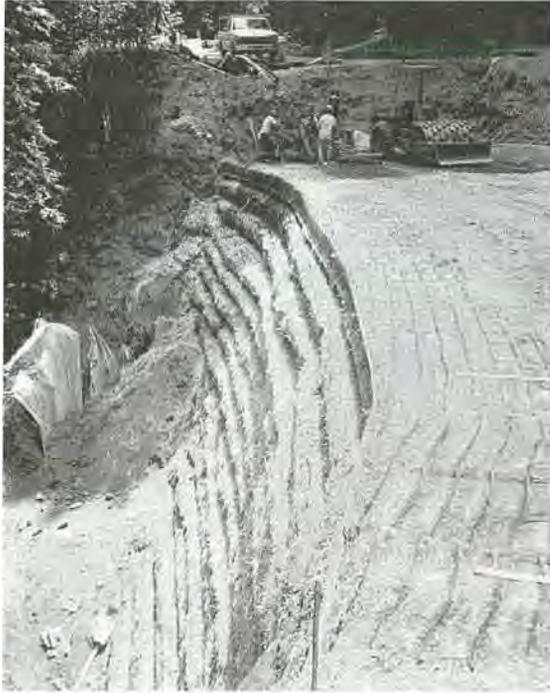
Caltrans project and other independent developments were the Hilfiker Welded Wire Wall (WWW), Hilfiker Reinforced Soil Embankment (RSE), VSL Retained Earth, and the Georgia Stabilized Embankment systems.
