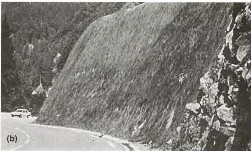
FIGURE 17-22 (above) Texsol: (a) wall under construction in French Alps; (b) 10-m-high Texsol slope with vegetation 1 year after construction.
