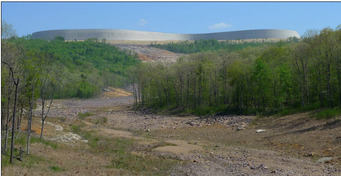
Fig. 21. – Overlooks within Johnson’s Shut-ins State Park provide excellent views of the scour path formed during the failure and rebuilt structure. This photograph shows the rebuilt RCC upper reservoir during the spring of 2010, just prior to the resumption of operations at the facility.
