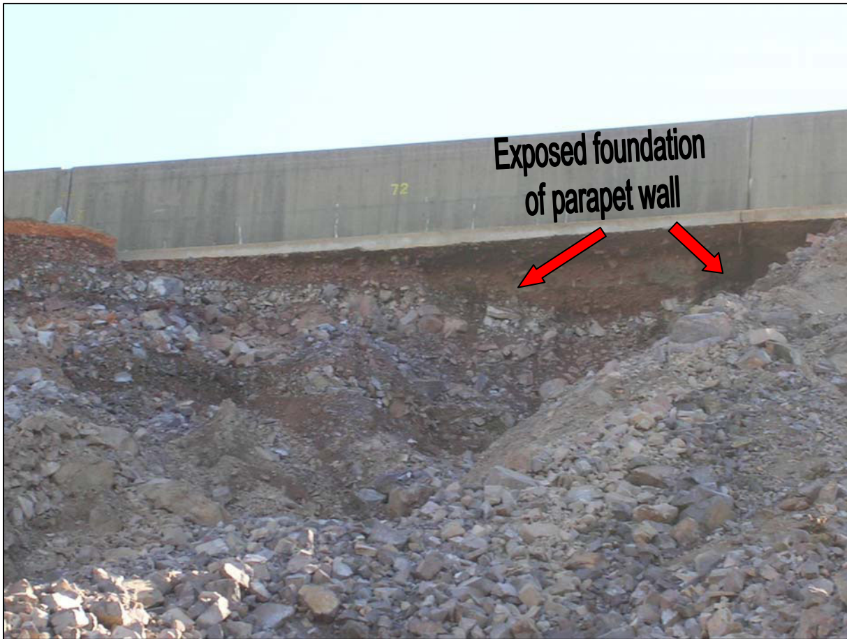
Fig. 7. – This photo taken below panels 71-72 show the deep plunge pool that developed and subsequent undercutting of the parapet wall. (Photo courtesy of David Hoffman).
