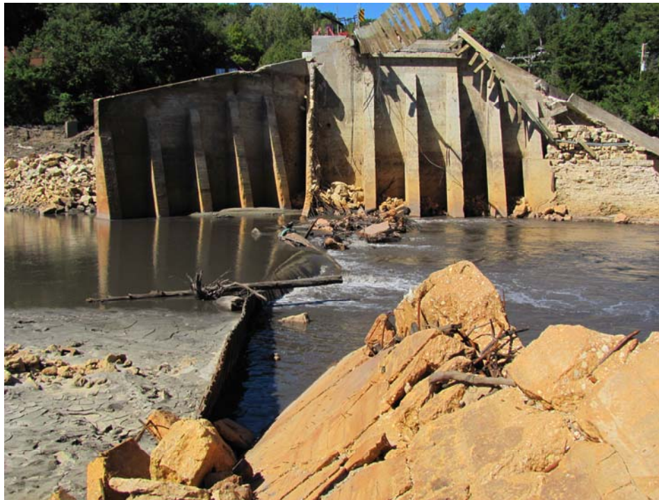
Figure 8. Remnants of sheet pile, core wall and spillway wingwalls. Source: Iowa DNR
