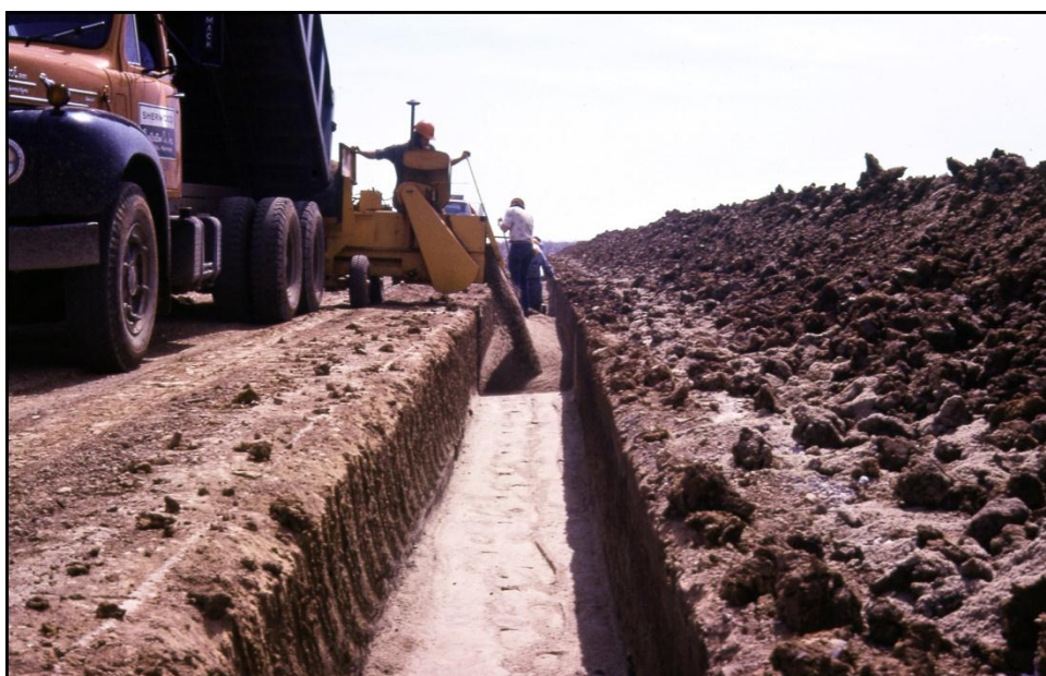
Figure 7-6. Trenching method – backfilling trench.
