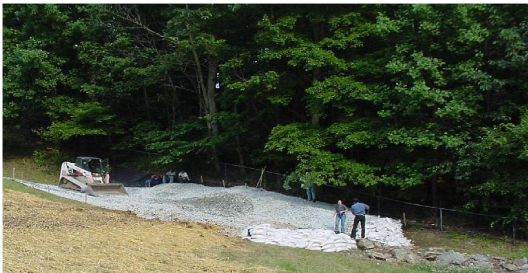
Figure L-26-2. Gravel drain being placed over seepage area.
