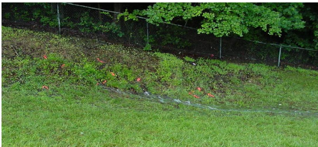
Figure L-26-1. Water discharging in the groin area downstream of an embankment during higher than normal reservoir storage. Seepage was through bedrock in the foundation that was not grouted. A gravel drainage layer was placed over the seepage to provide a controlled outlet. The seepage was not carrying fines, which would have been problematic to deal with because a fine filter would be required to block the fines but a coarse filter was required for capacity. In this case, the gravel layer provided a collector mechanism, with no filtering being required.
