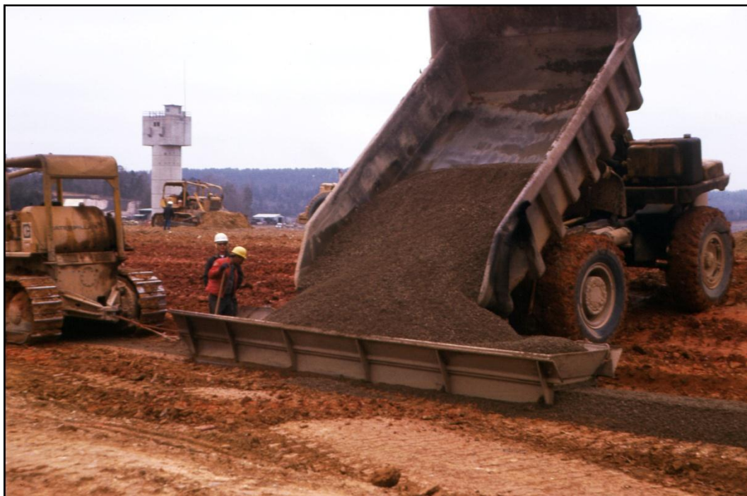
Figure 7-16. Dumping into spreader box.
