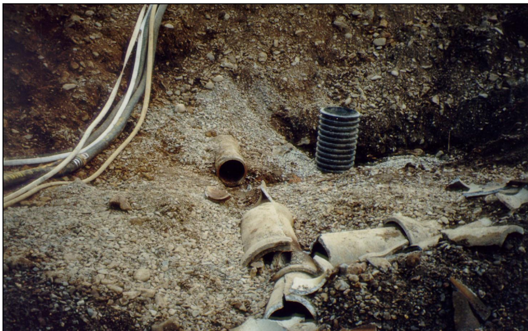
Figure 2-15. 1950s era concrete pipe used as a toe drain. Water enters the pipe through a gap left in the bell and spigot joints. A “Y” junction is shown with two laterals that connect to a trunk line shown on the right side of the photo. Since connectors were not manufactured for this configuration, intact pieces of pipe were broken and the pieces used to stack together, making a protective cap for the junction. This junction was exposed during excavation for a toe drain replacement.
