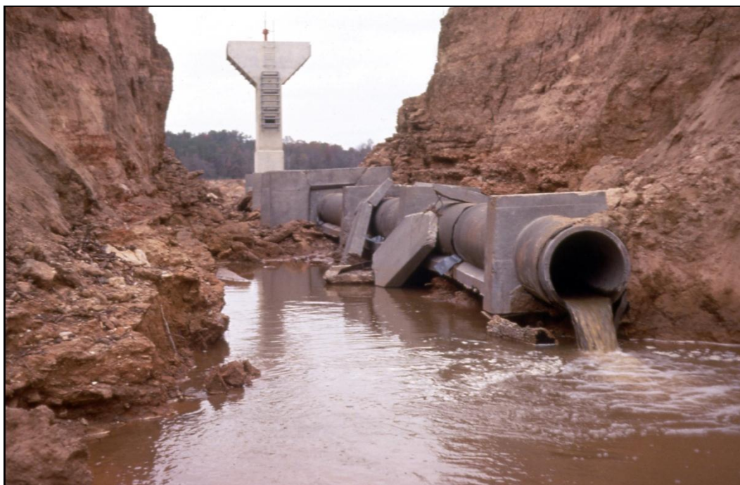
Figure 2-5. Embankment dam breached after piping along the conduit. The view is upstream. Note pre-cast concrete pipe placed on a concrete cradle and the use of seepage collars (Photo credit NRCS).
