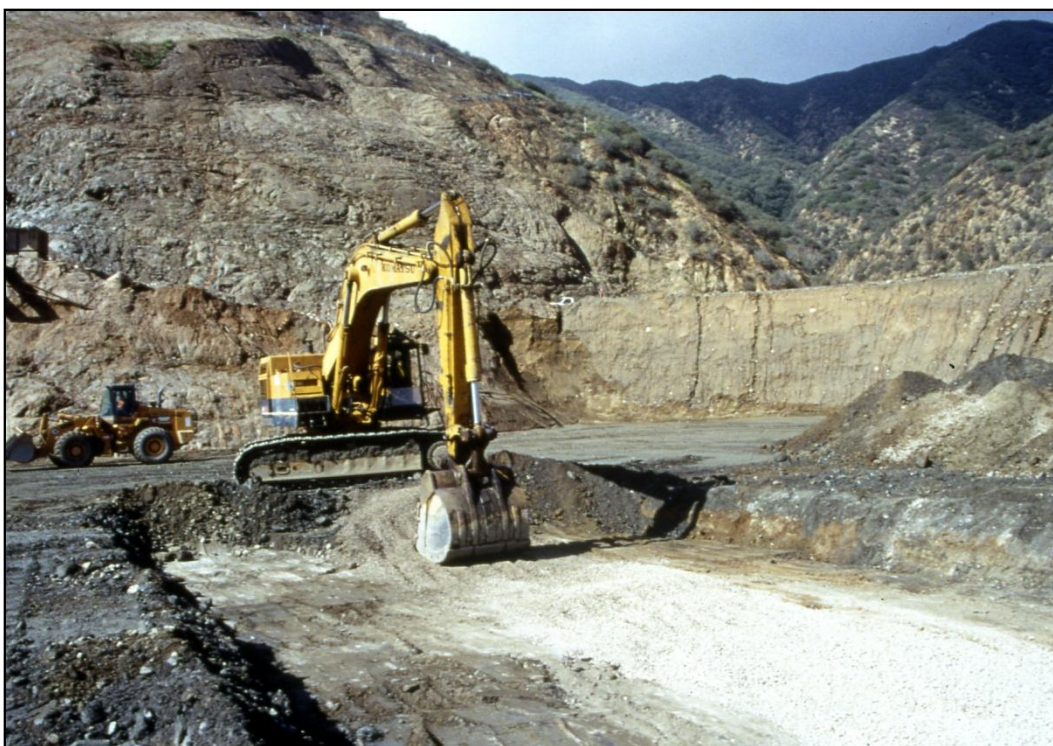
Figure 7-27. Excavation of filter material under equipment crossing.
