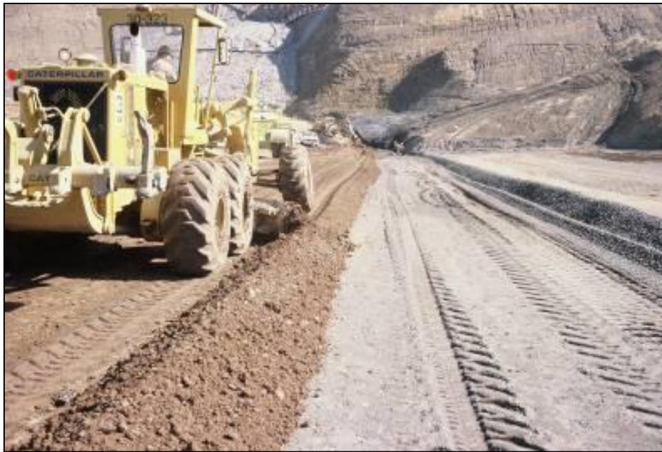
Figure 7-3. Windrowing impervious material adjacent to a filter/drain.
