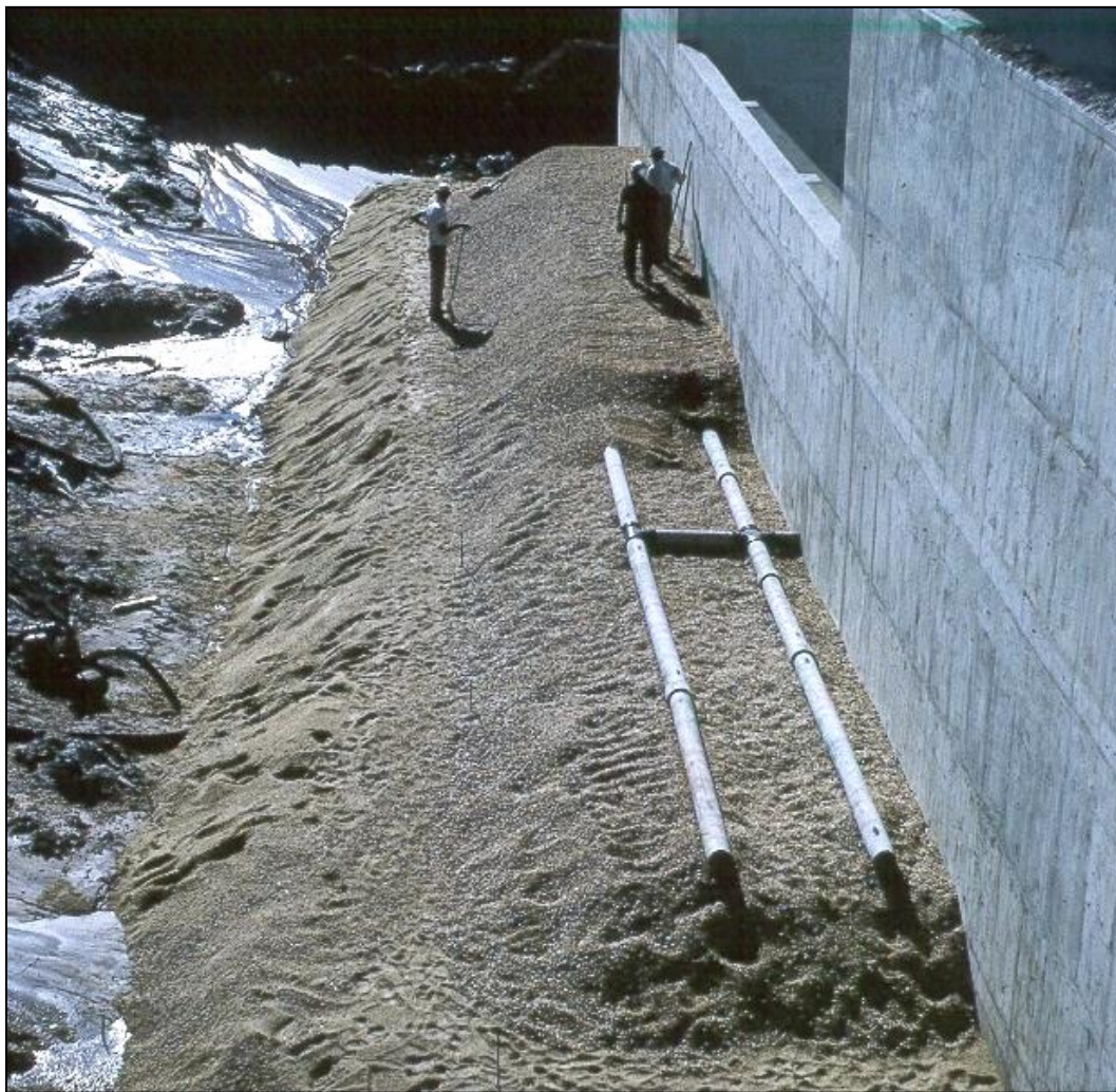
Figure 2-7. Filter and drainage zones to provide pressure relief and drainage of backfill next to training wall for a spillway chute. One individual is standing on top of the sand layer (Photo courtesy of NRCS, Texas).
