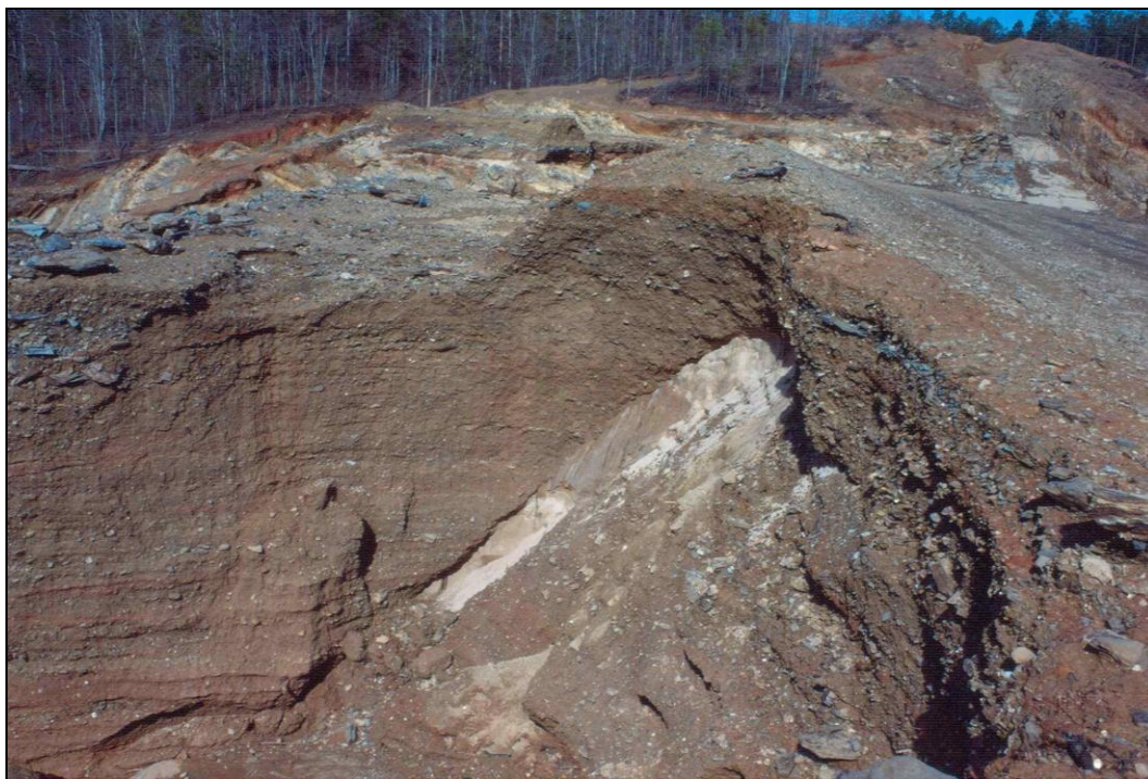
Figure E-4. View toward right abutment showing remnant of chimney filter/drain in cross-sectional view. Chimney filter/drain was 3 ft wide.
