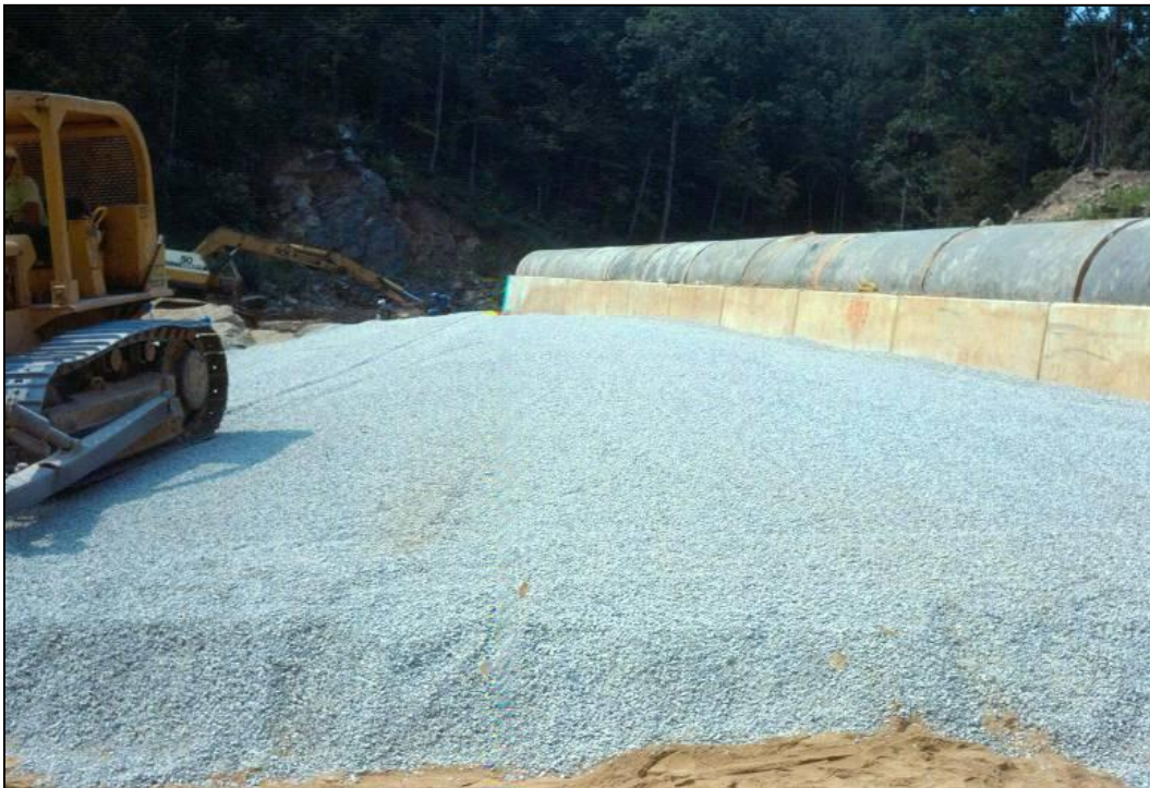
Figure 2-10. Gravel blanket drain being placed over fine filter shown in Figure 2-9. (Photo courtesy of NRCS, Alabama.)
