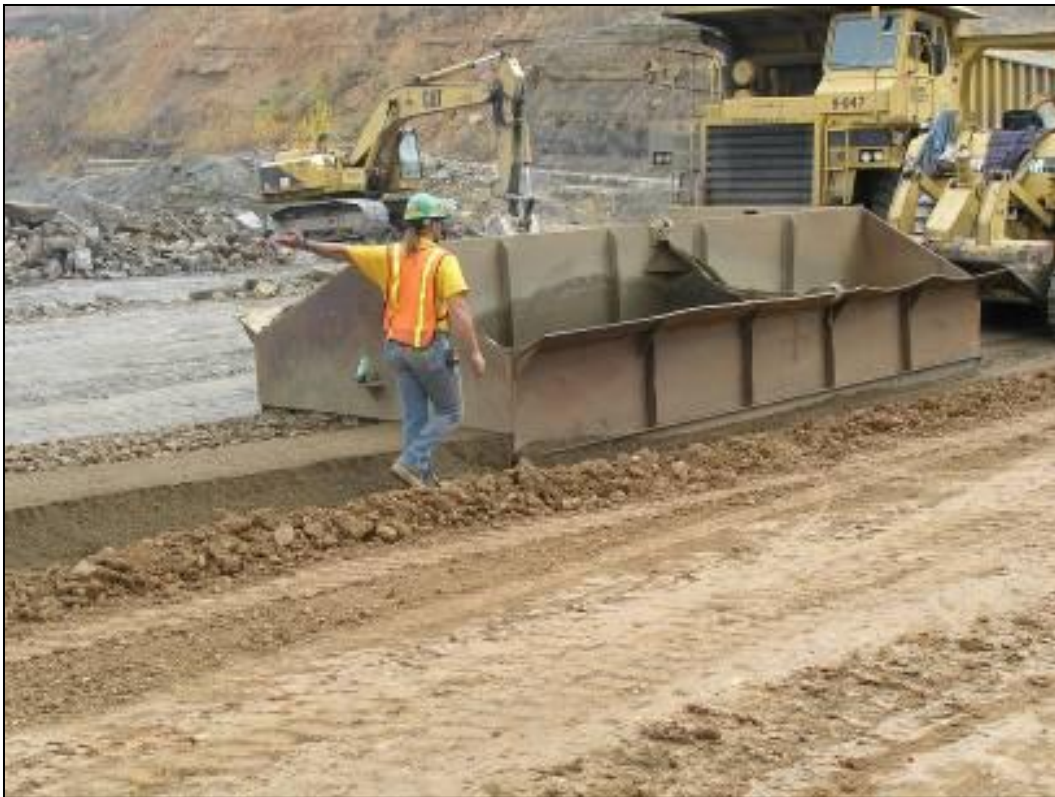
Figure 7-17. Towing spreader box.
