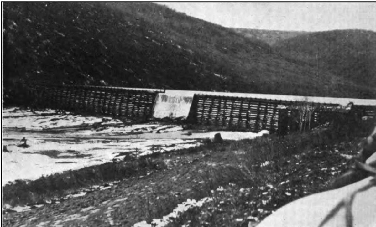
**Figure 4** – Timber-Crib Dam – Completed June 1910 <sup>[10]</sup>
