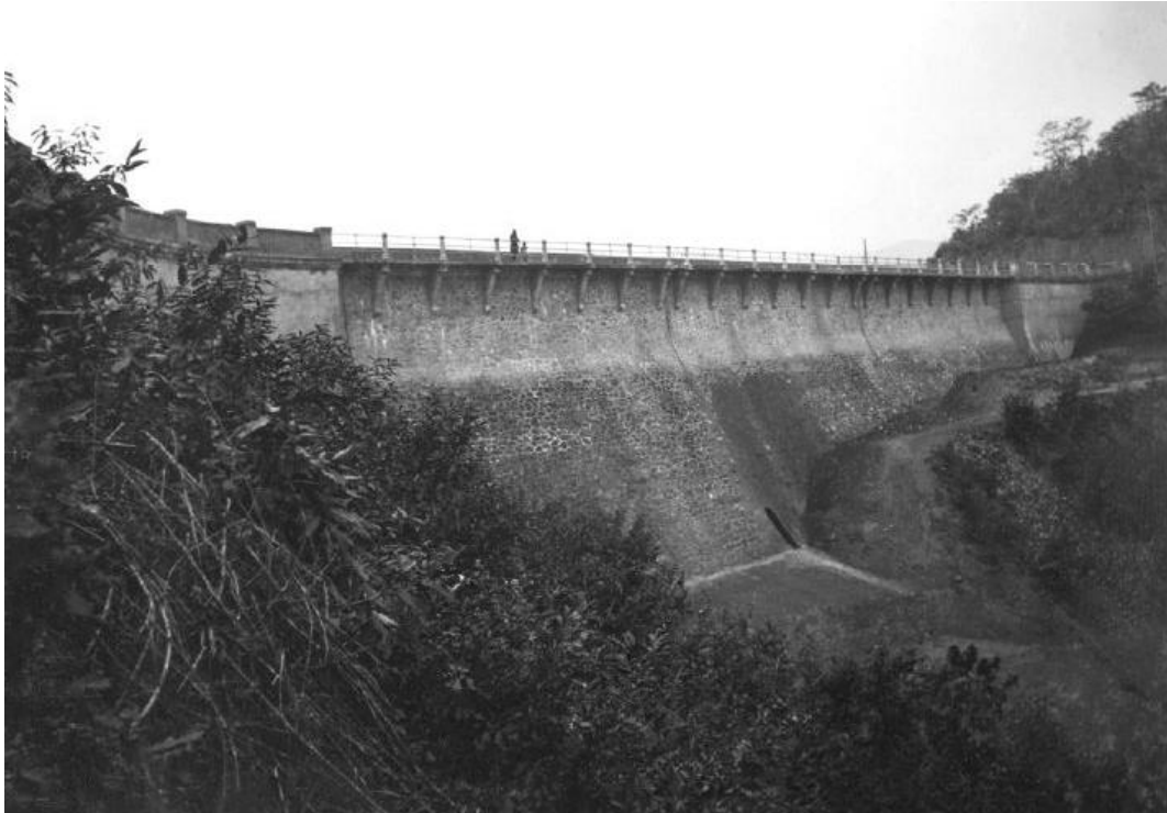
Figure 7. Downstream Face of Secondary Dam
