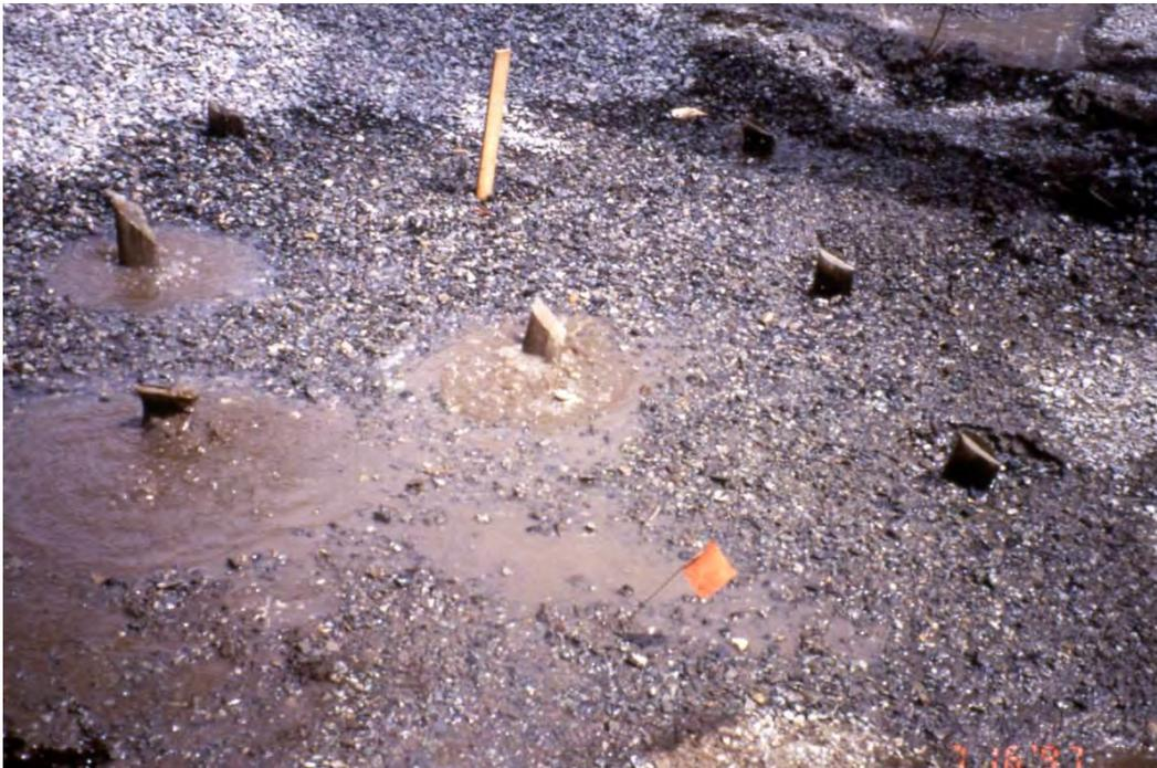
**Figure G9c. Wick drains discharging water during stone column installation, Salmon Lake Dam, Washington.**
