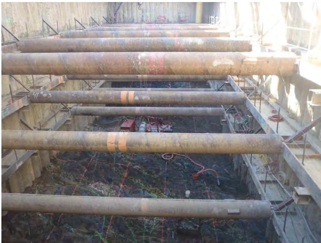
**Figure G4b.** Excavation bracing for the key block at MIAD, Folsom, California (2011).
