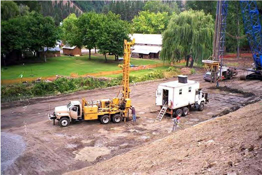
**Figure G2. Verification testing with SPT and CPT to confirm sufficient densification by Stone Column Construction at Salmon Lake Dam. Stone column equipment appears at the far right side of the photograph.**
