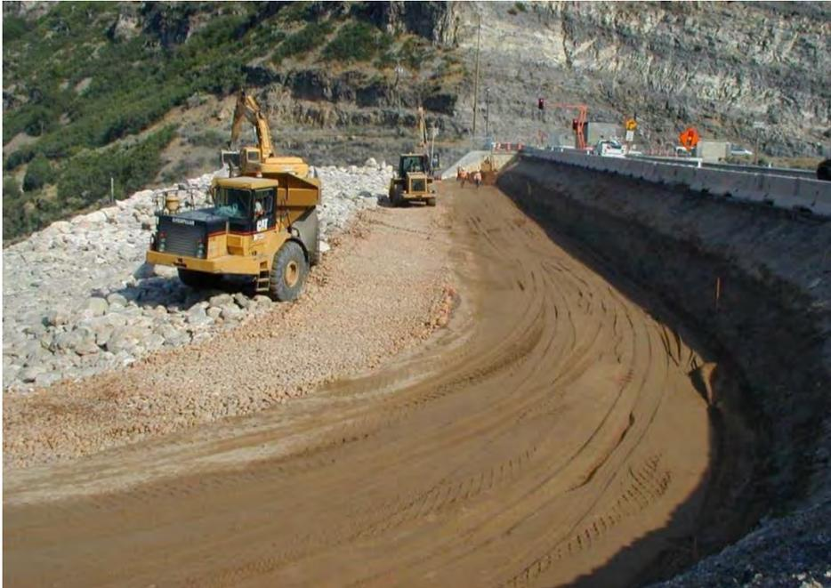
Figure G18. Placement of flowthrough rockfill, transition, and filter zones, downstream to upstream (left to right), Pineview Dam modification, Utah.
