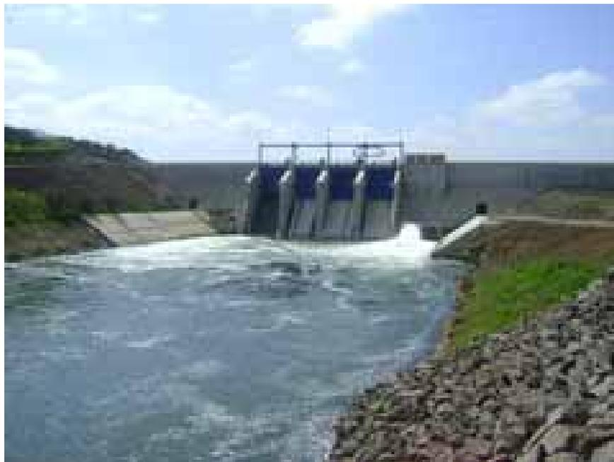
Figure 2. Spillway/outlet from downstream (from Google Maps, R. Castillo).
