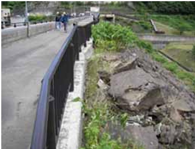
Figure 7. Displaced rock on downstream slope (from Yamaguchi, 2010).
