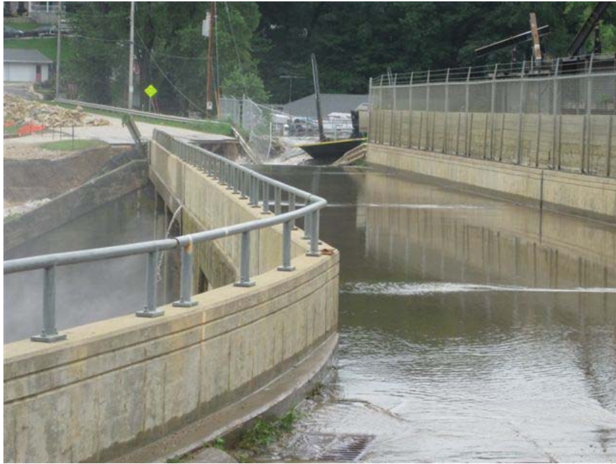
Figure 11. Breach in progress, headcut deepening through roadway. Source: Iowa DNR.
