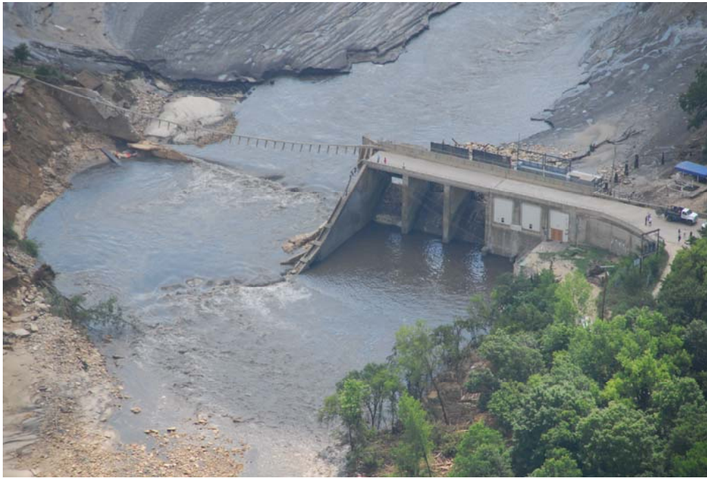
Figure 15. Aerial view of breach. Source: Iowa Wing Civil Air Patrol.
