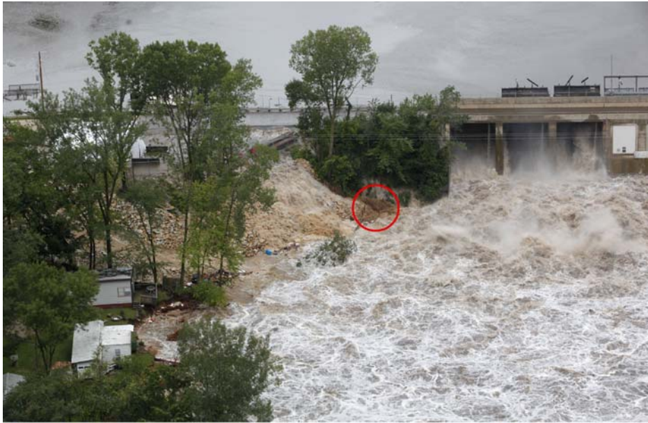
Figure 9. Discolored water (circled) exiting the dam, indicating piping. Source: SourceMedia Group News
