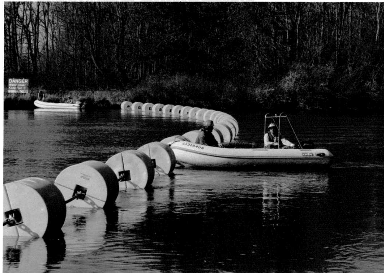
Figure 6: Installation of upstream public safety boom.
